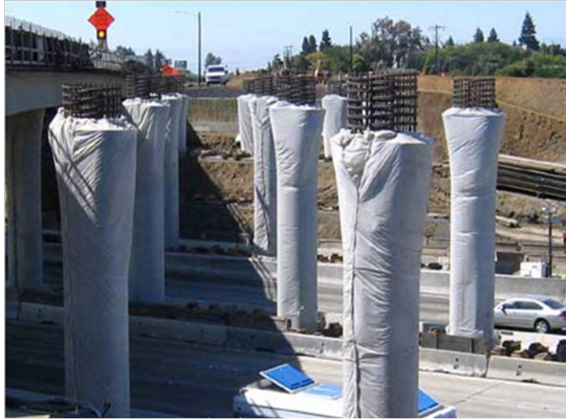
Figure 5-23. Curing Concrete Columns Using Polyethylene Plastic Sheets.
