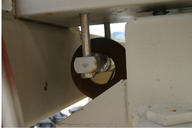
Figure 4-7. Load Cell at One Corner of a Weigh Hopper.
