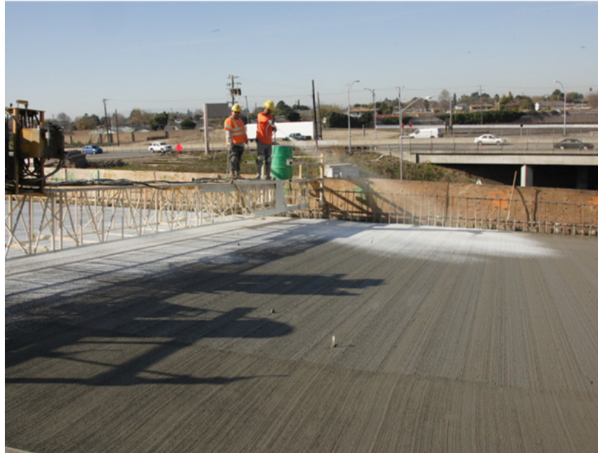
Figure 5-27. Applying Curing Compound Using Power-Operated Spray Equipment.
