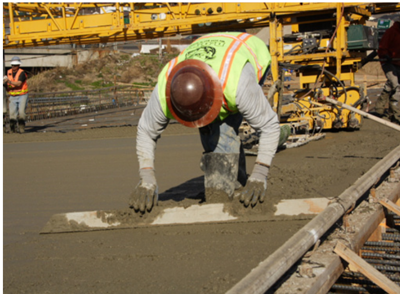
Figure 5-15. Striking Off Bridge Deck Concrete.
