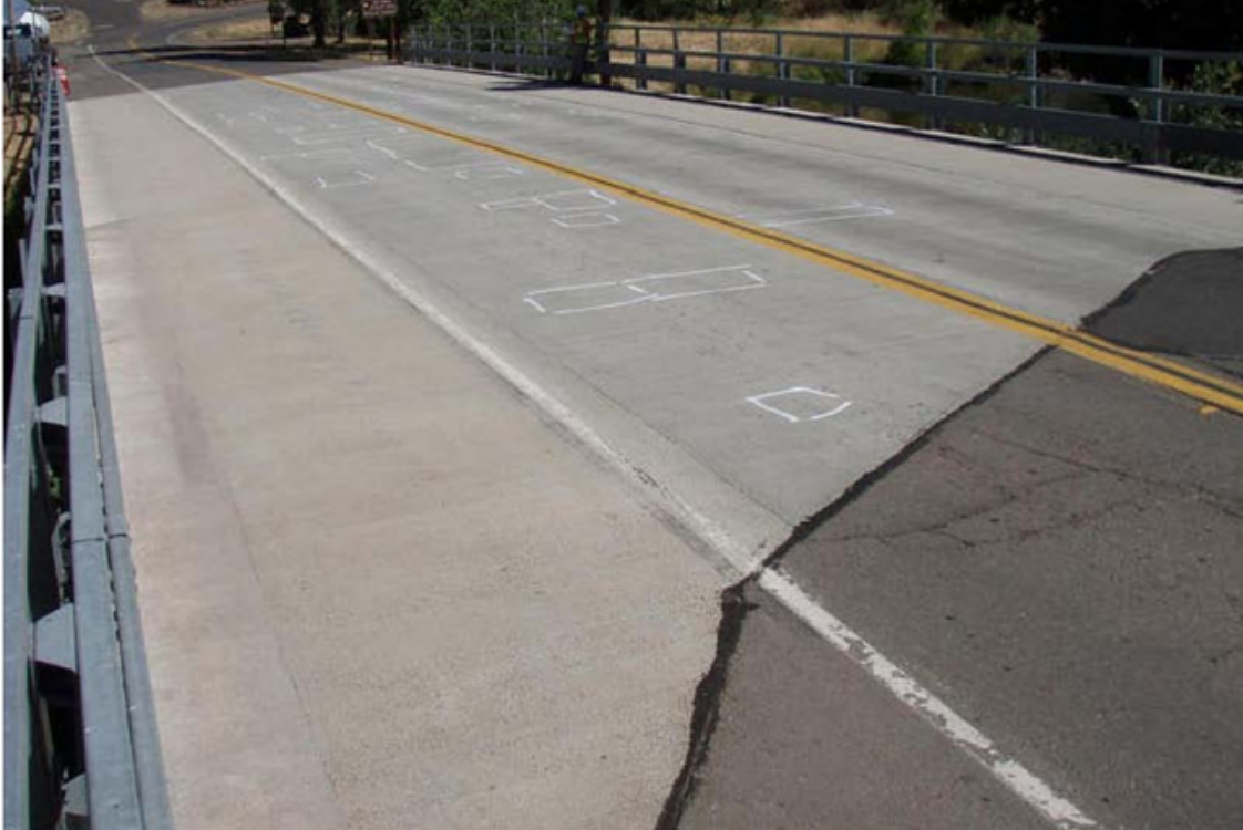
Figure 6-7. Delaminated Deck Surfaces Identified for Replacement.
