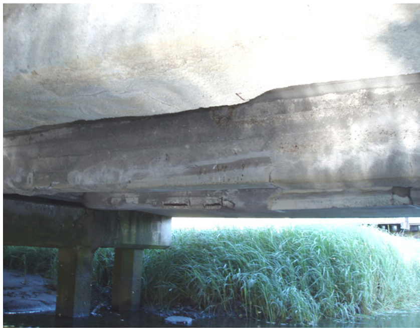
Figure 1-5. Corrosive Girder Spalling.
