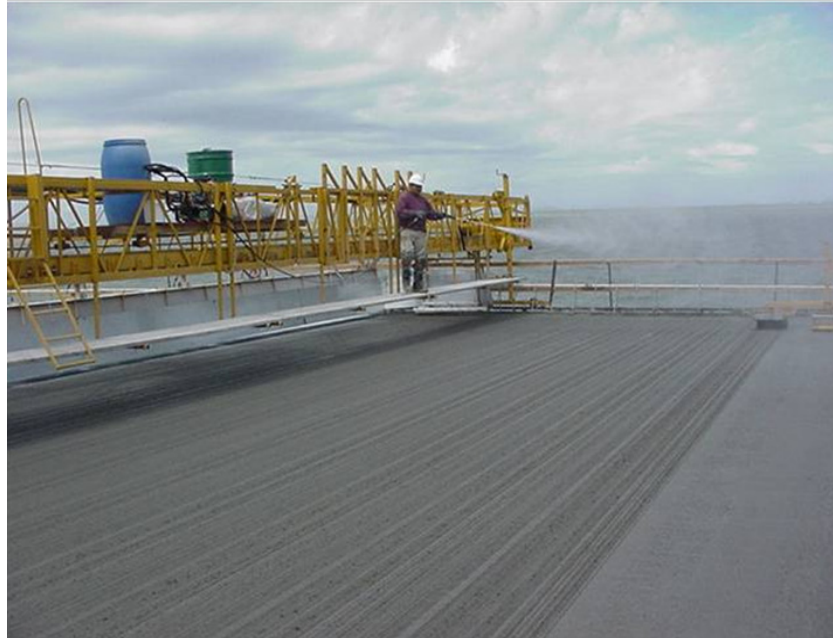
Figure 5-26. Fogging Bridge Deck to Minimize Plastic Cracking.
