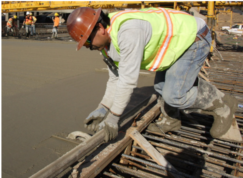
Figure 5-16. Hand Floating a Bridge Deck.
