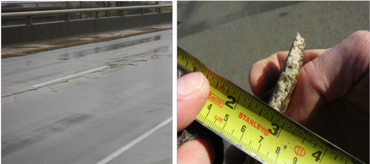
Figure 6-19. Polyester Overlay Spalling.
