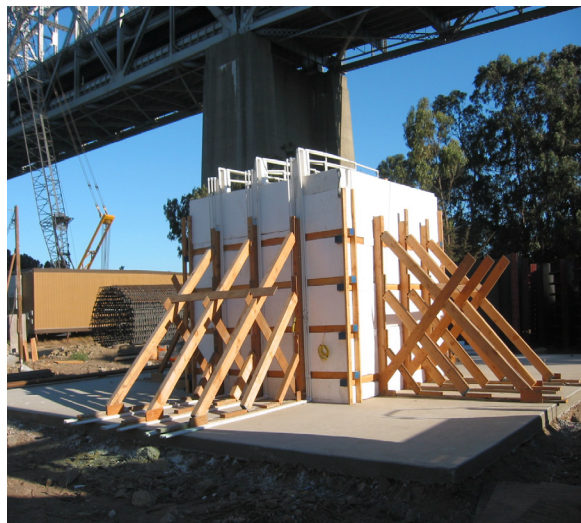
Figure 7-24. Footing Mock-up 10-ft Cube.
