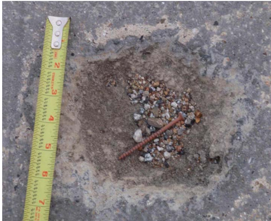
Figure 6-4. Severe Bridge Deck Scaling, Small Pothole.
