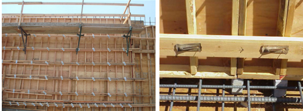
Figure 5-2. Typical Concrete Wall Forms.
