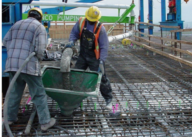
Figure 5-12. Depositing Concrete Using a Drop Chute.
