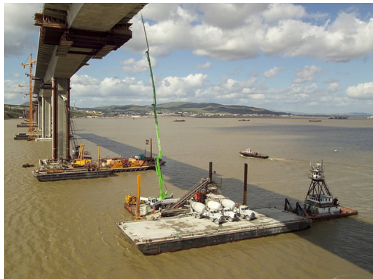
Figure 5-8. Benicia-Martinez Concrete Pumping.
