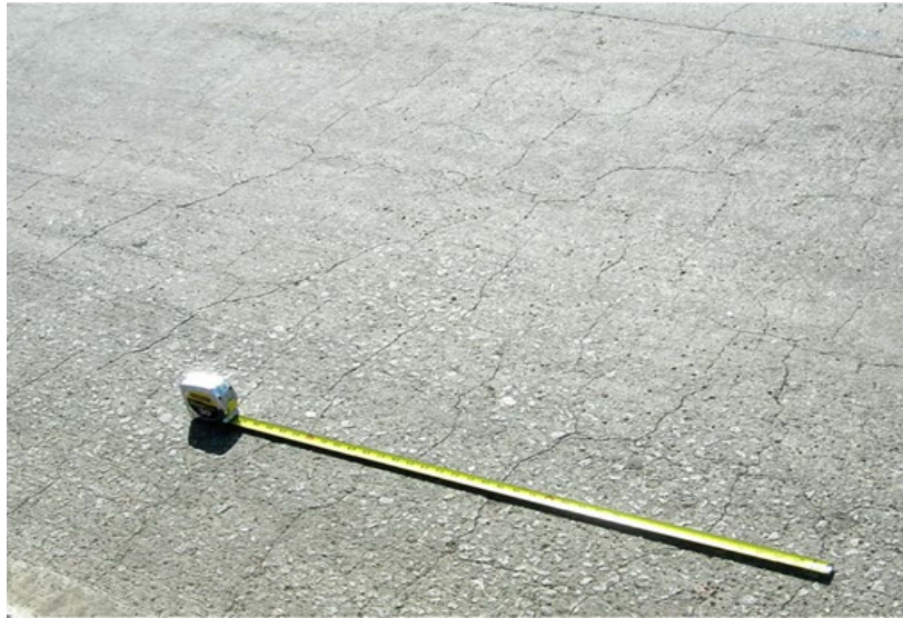
Figure 6-3. Map Cracking.
