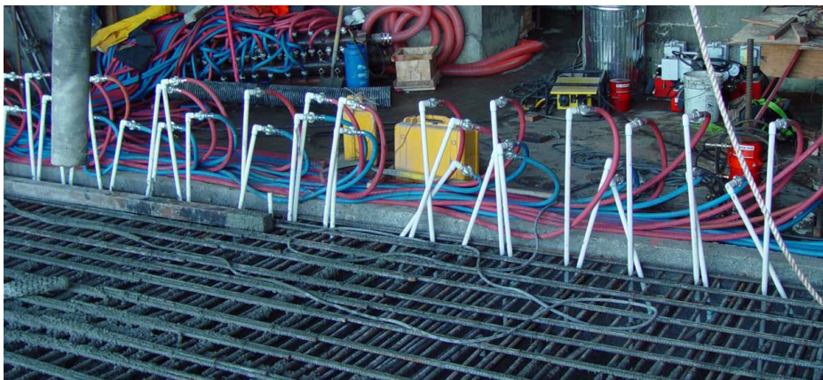
Figure 7-26. Soffit Cooling Pipe Manifold.
