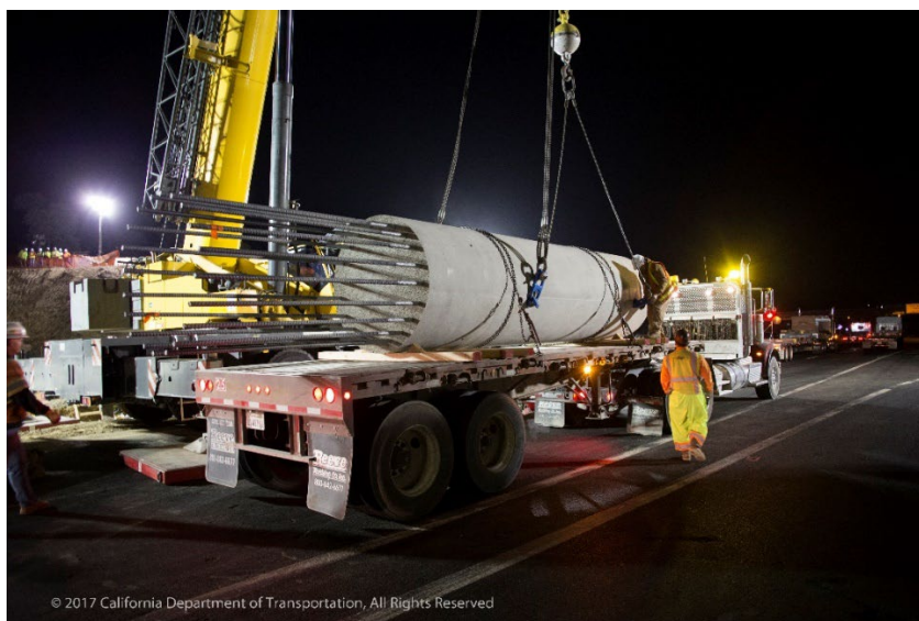
Figure 8-9. PC Concrete Handled at Pick Points
