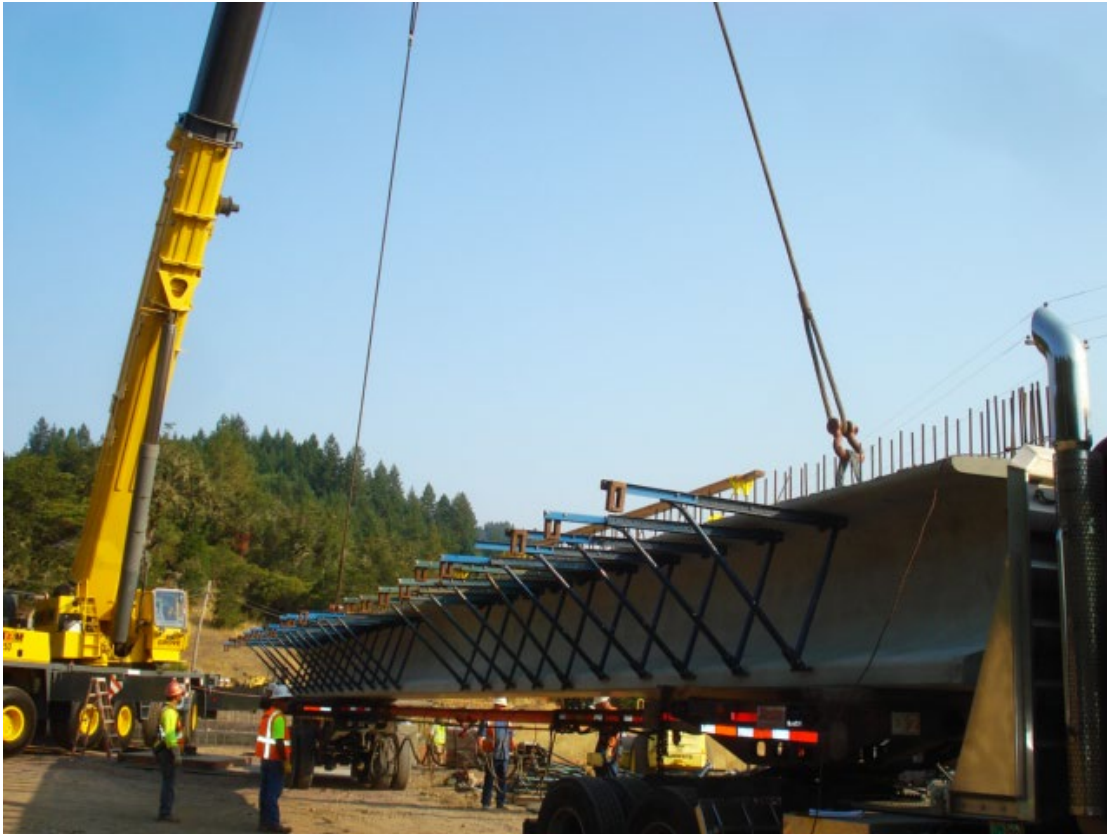
Figure 8-17. Overhang Formwork Brackets Before Girder Installation
