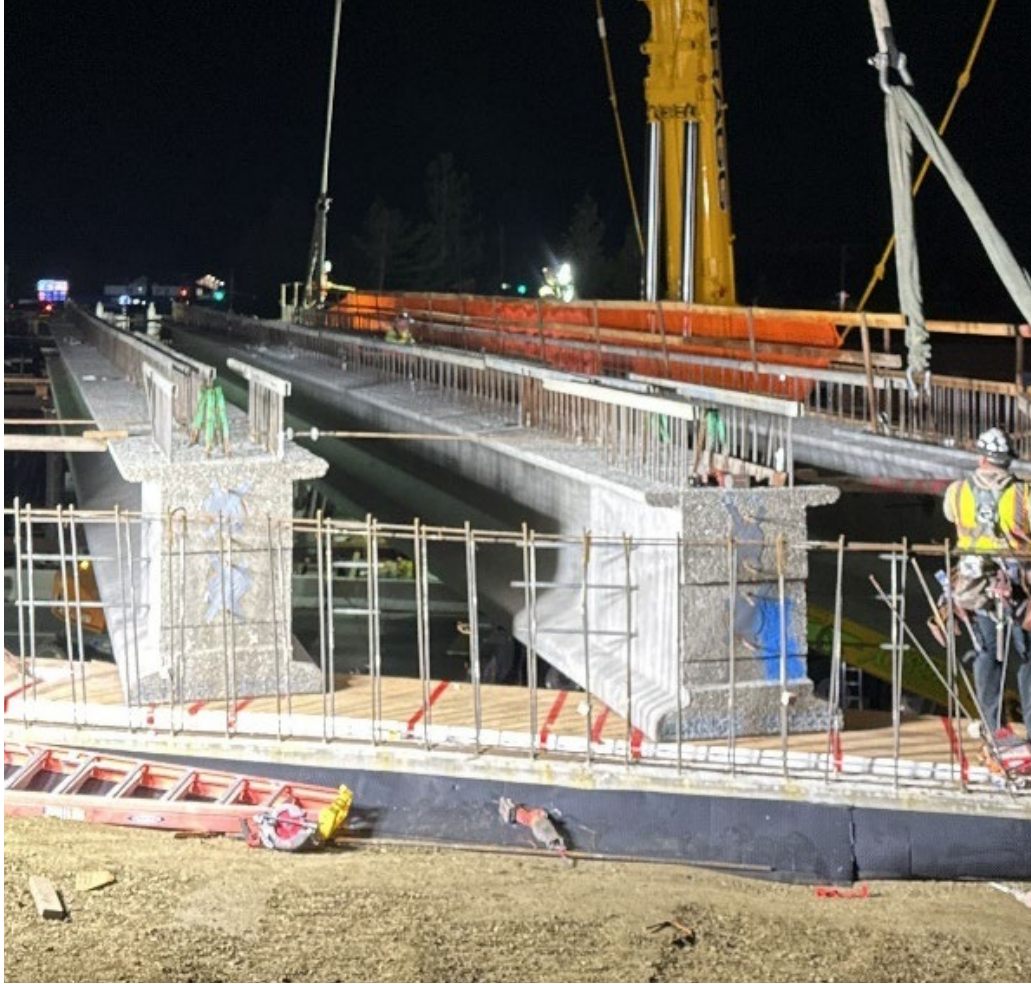
Figure 8-14. Bar Reinforcement Impalement Protection
