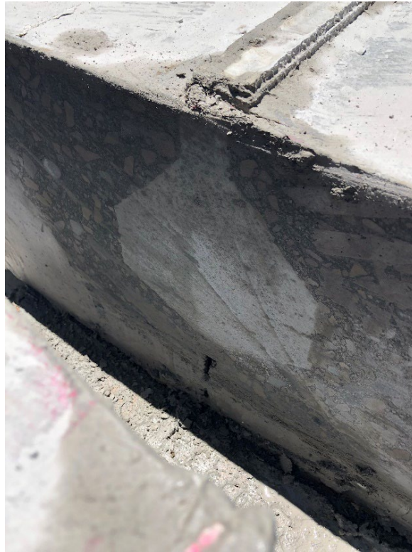
Figure 8-22. Grouted Keyway Filled With UHPC
