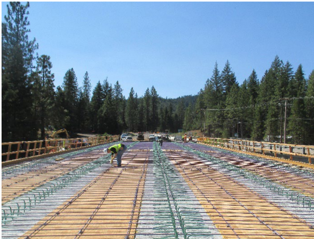
Figure 8-16. Bending of Epoxy-Coated Bar Reinforcement Stirrups
