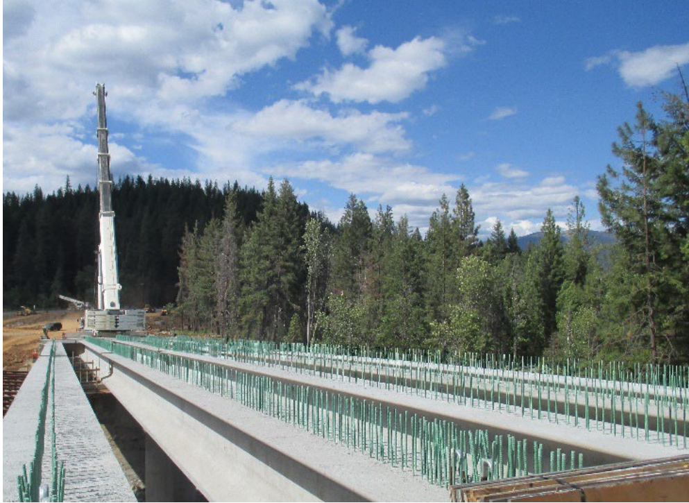
Figure 8-15. Unbent Epoxy-Coated Bar Reinforcement Stirrups
