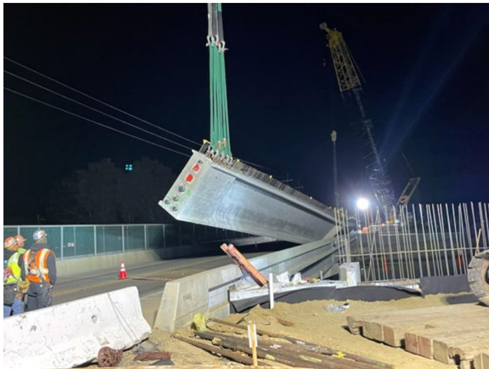
Figure 8-10. PC PS Girder Failure During Picking
