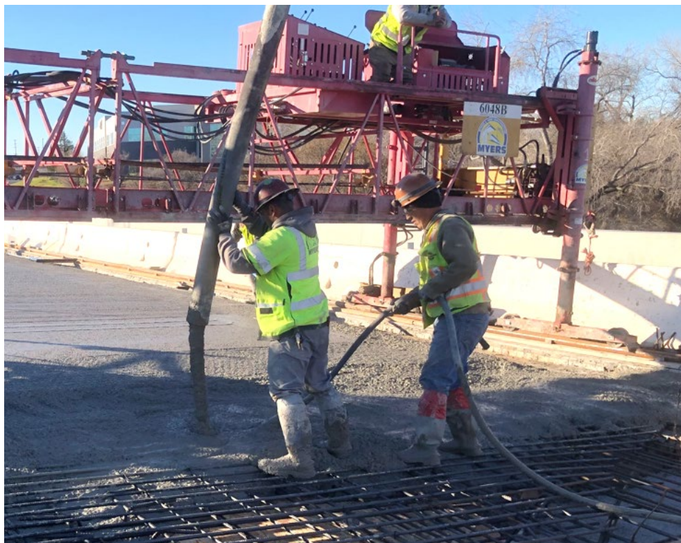
Figure 7-27. Vibrating Concrete on a Deck Pour
