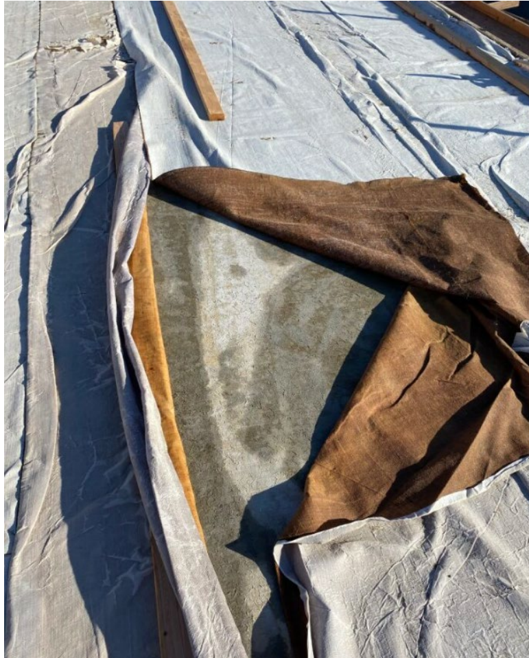
Figure 7-34. Wet Curing Blankets
