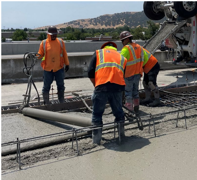
Figure 7-26. Roller Screed for Deck Finishing
