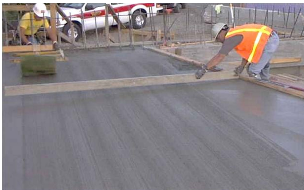
Figure 7-20. Checking Freshly Placed Deck Concrete Near the Expansion Joint Blockout
