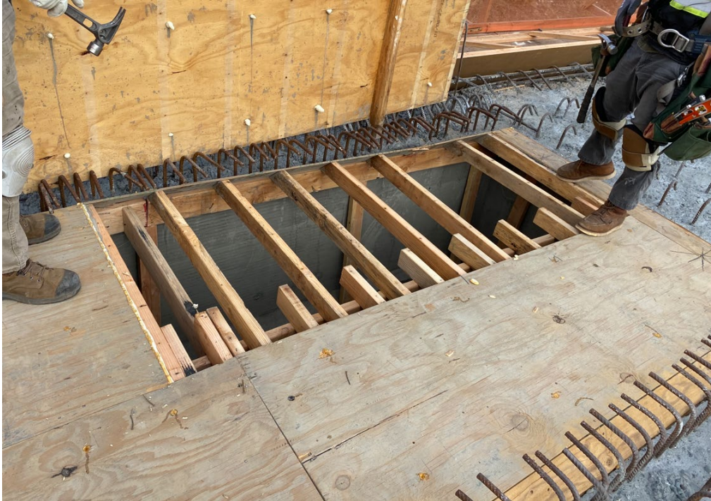
Figure 7-3. Typical Deck Sheathing and Supports on a CIP Box Girder Bridge
