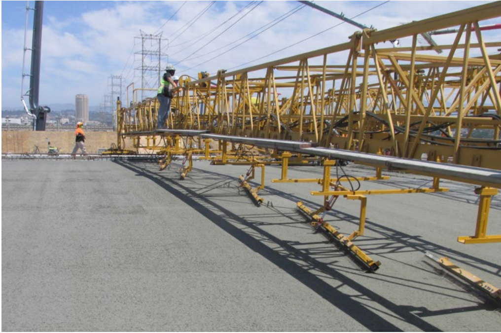
Figure 7-31. Longitudinal Tining from a Work Bridge
