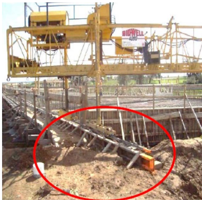
Figure 7-19. Screed Rails Extended Beyond Pour Limits
