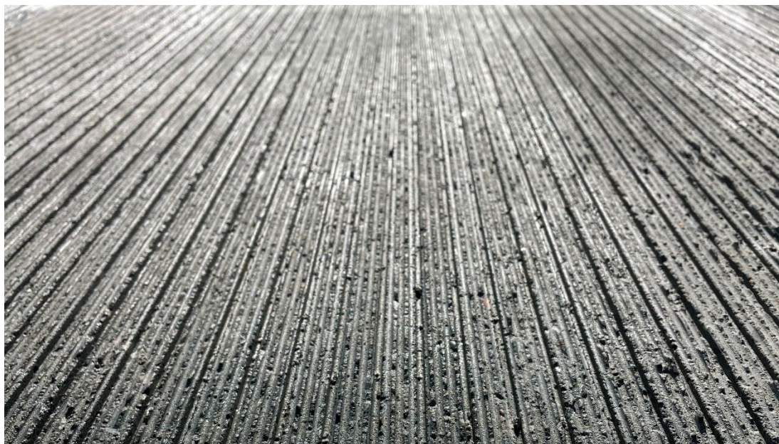
Figure 7-30. Close-up Illustration of Grooved Deck
