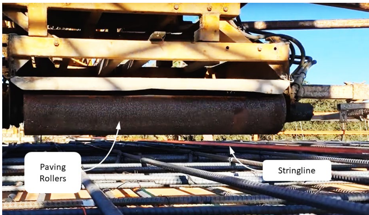
Figure 7-24. Check Finishing Machine Height
