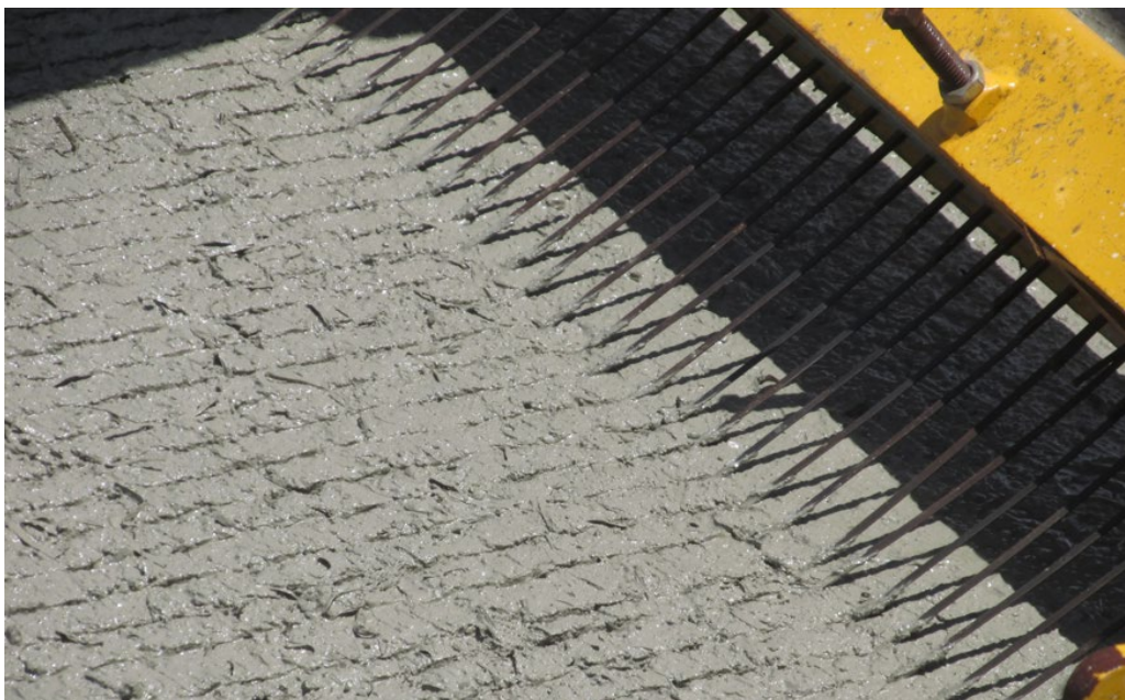
Figure 7-32. Longitudinal Tining
