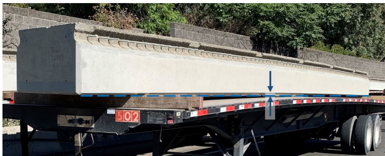
Figure 7-16. PC PS Girder Camber
