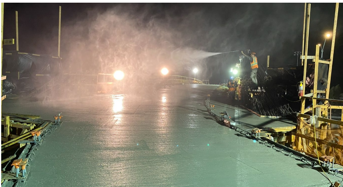
Figure 7-33. Application of Atomized Mist on Bridge Deck
