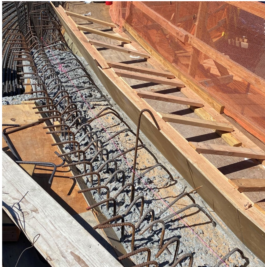
Figure 7-10. Deck Dowels (Hook Bars)
