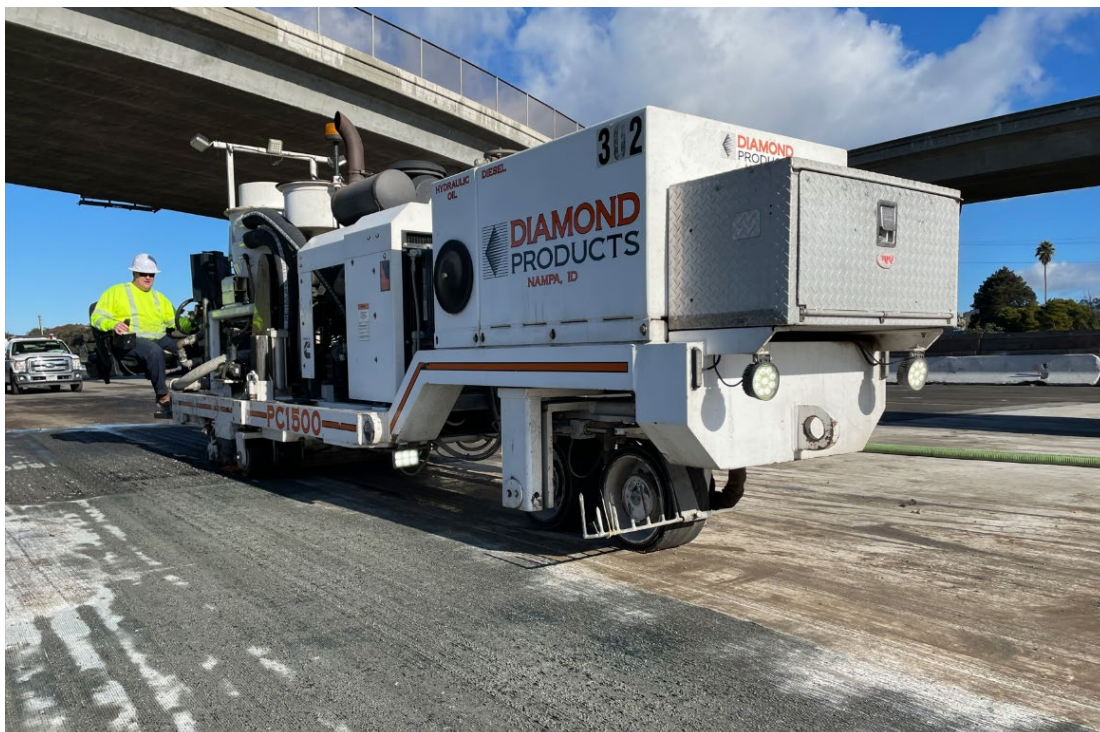
Figure 7-29. Grinding Machine Grooving a Bridge Deck
