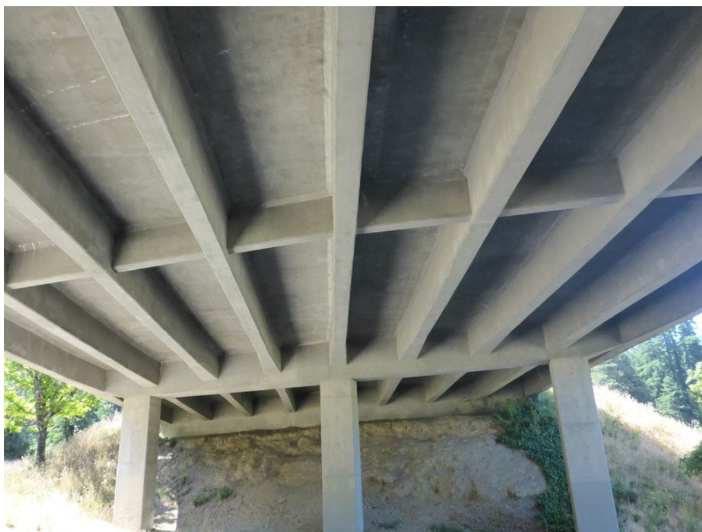
Figure 7-6. Example of a T-Beam Bridge (Newton Road UC, Br No. 04 0125)
