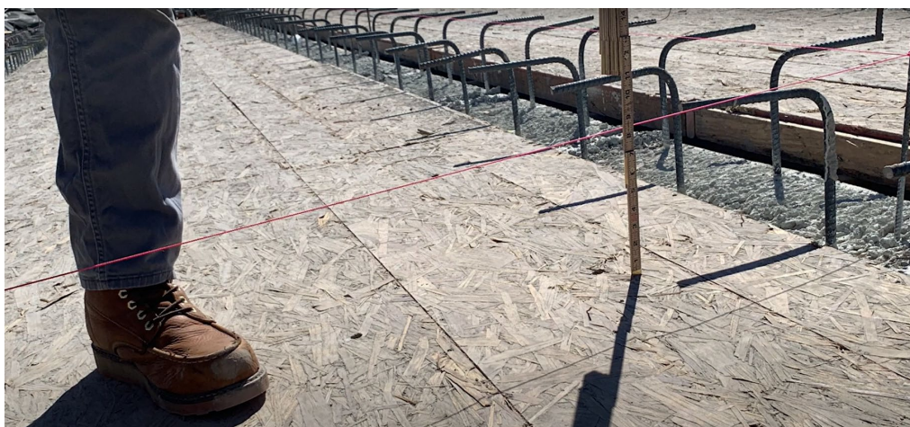
Figure 7-17. Lost Deck Measurements
