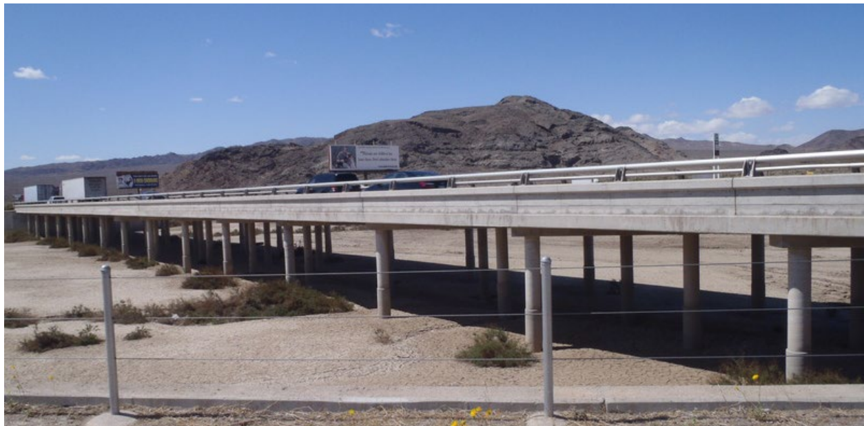
Figure 7-4. Example of a Slab Bridge (Mojave River Bridge, Br No. 54 0278L)
