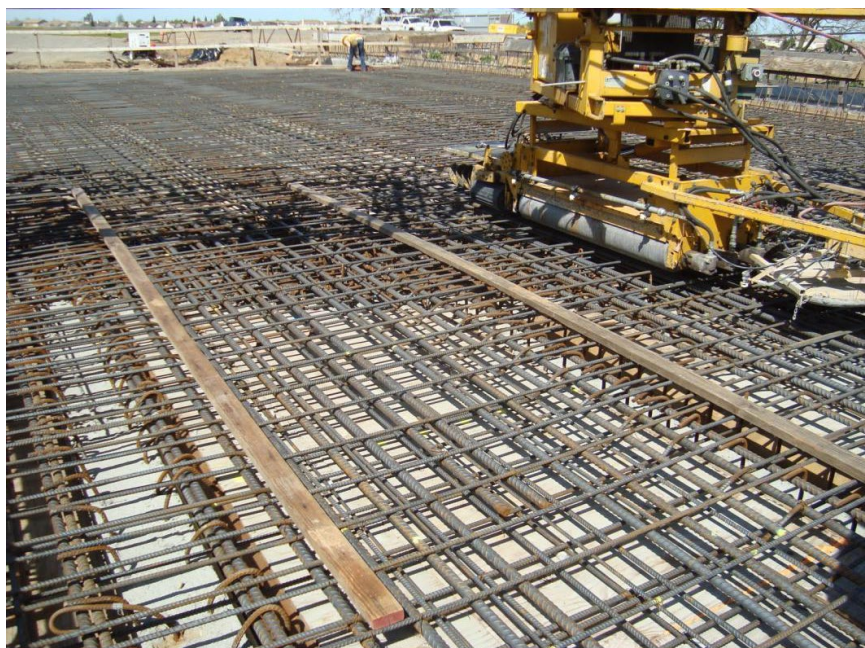
Figure 7-25. Clearance Checking with Lumber
