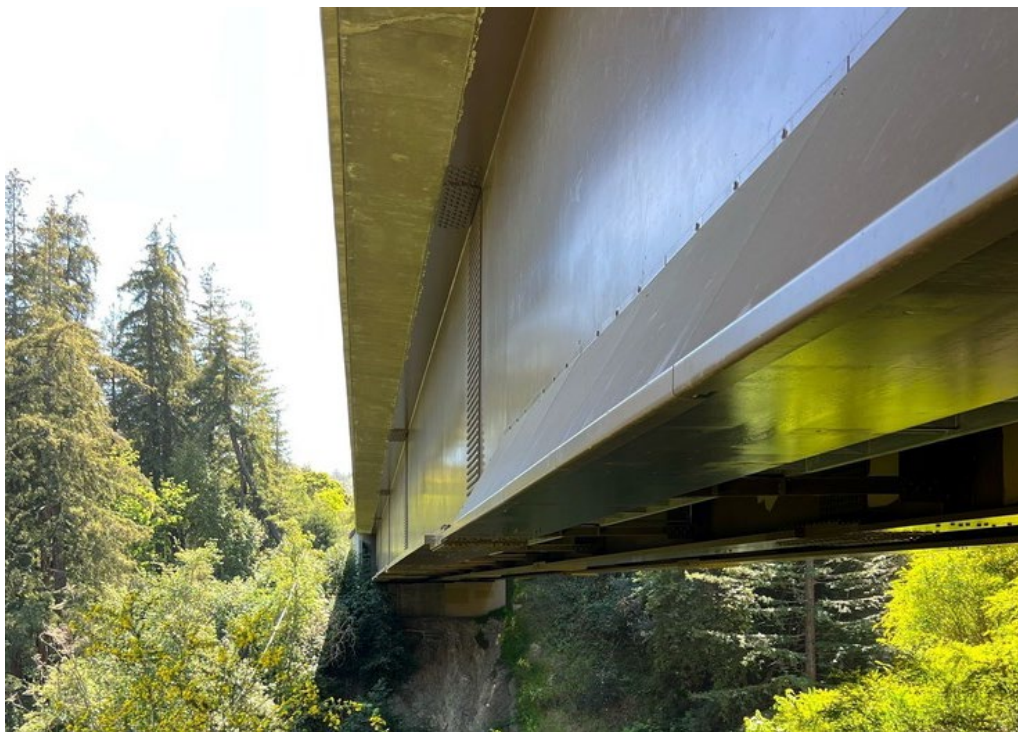
Figure 7-5. Example of a Steel Girder Bridge (Pfeiffer Canyon Bridge, Br No. 44 0298)
