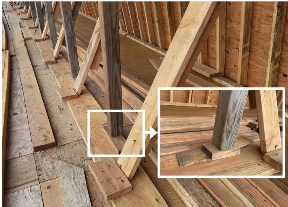
Figure 7-14. Wedge System for the Overhang
