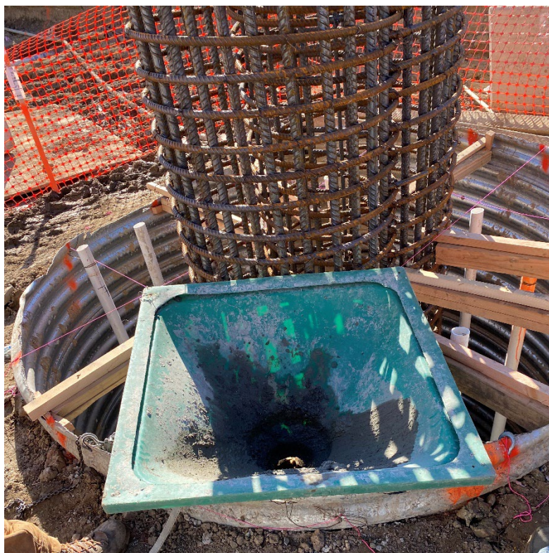
Figure 6-1. Hopper Placed at Top of Drilled Hole
