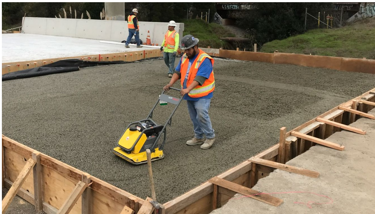
Figure 6-18. Cement Treated Permeable Base for Approach Slab
