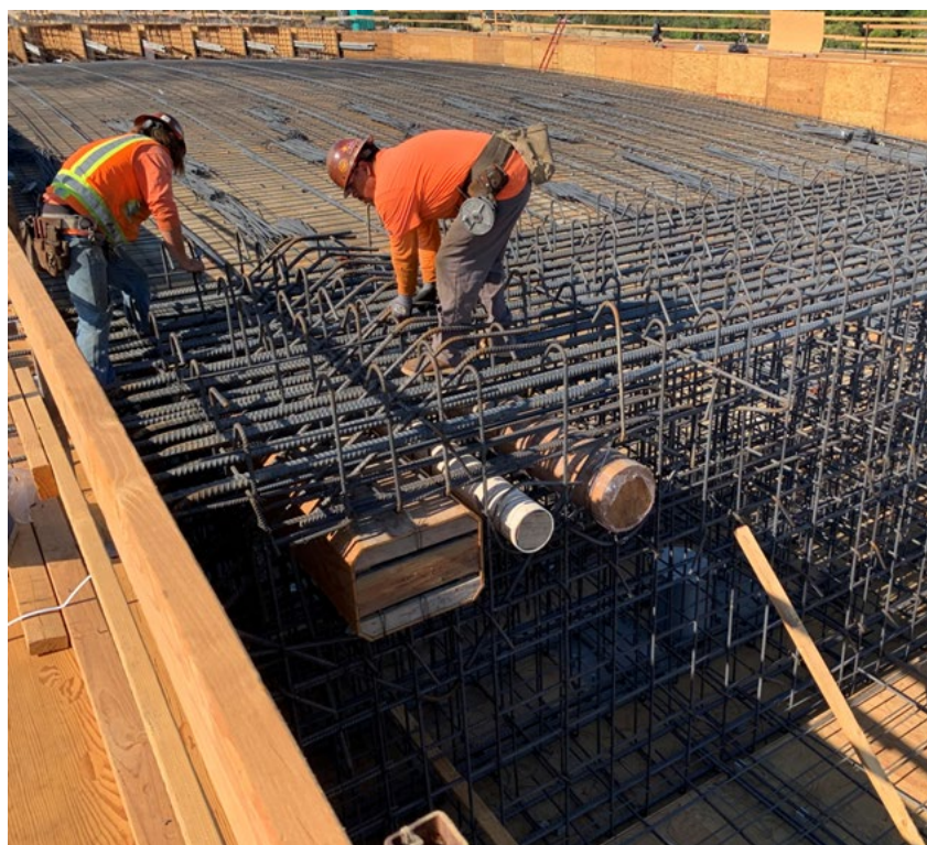
Figure 6-6. Bent Cap Bar Reinforcement Installation with Blockouts
