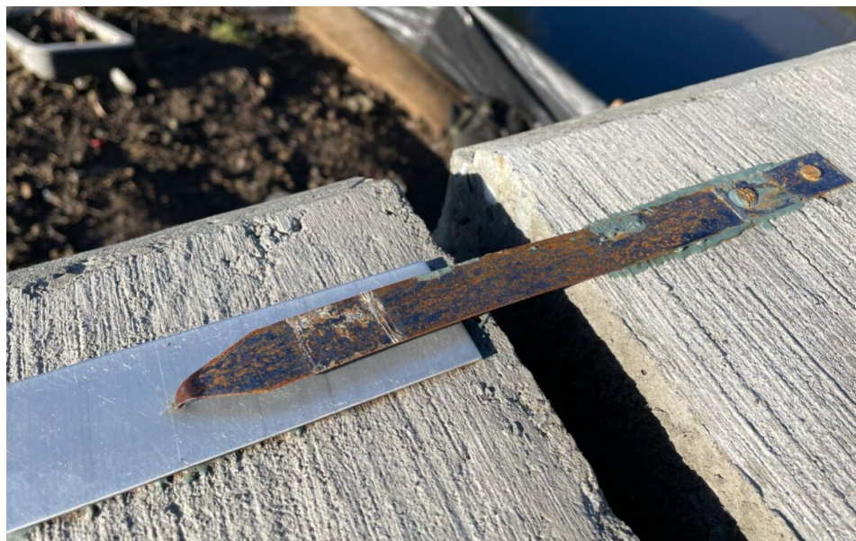
Figure 6-14. Expansion Joint Scribe
