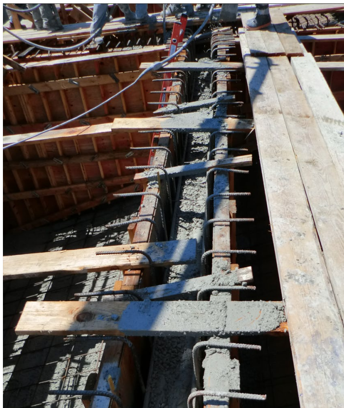
Figure 6-10. Stem and Soffit Concrete Placement
