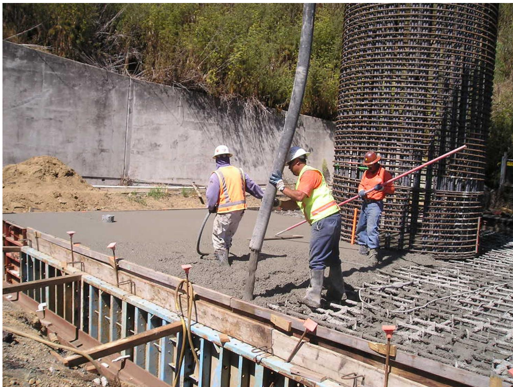
Figure 6-2. Footing Concrete Placement
