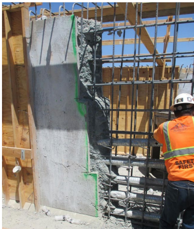
Figure 6-9. Girder Stem Construction Joint
