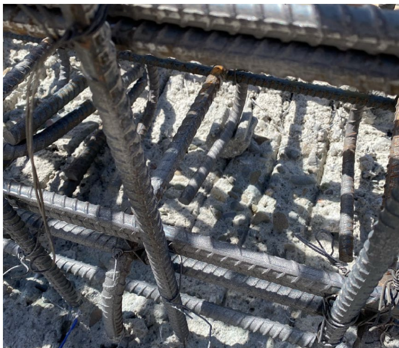
Figure 6-11. Construction Joint 1/4 Inch Roughening
