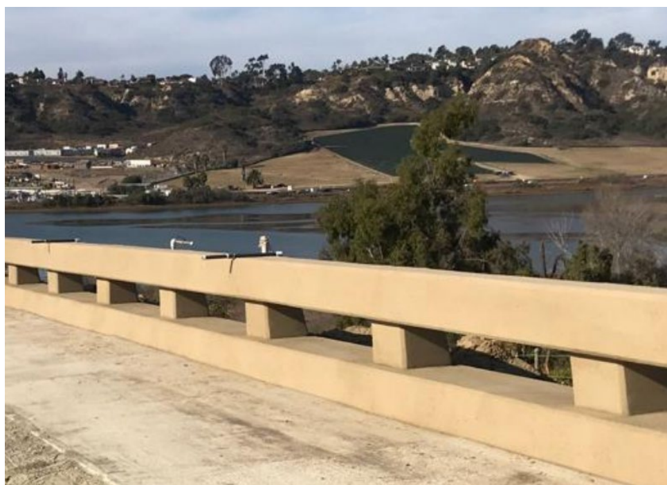
Figure 6-13. Type 80 Series Barrier
