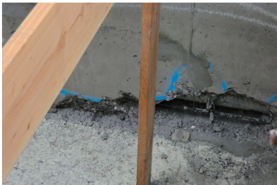
Figure 6-7. Rock Pockets Below Prestressing Ducts
