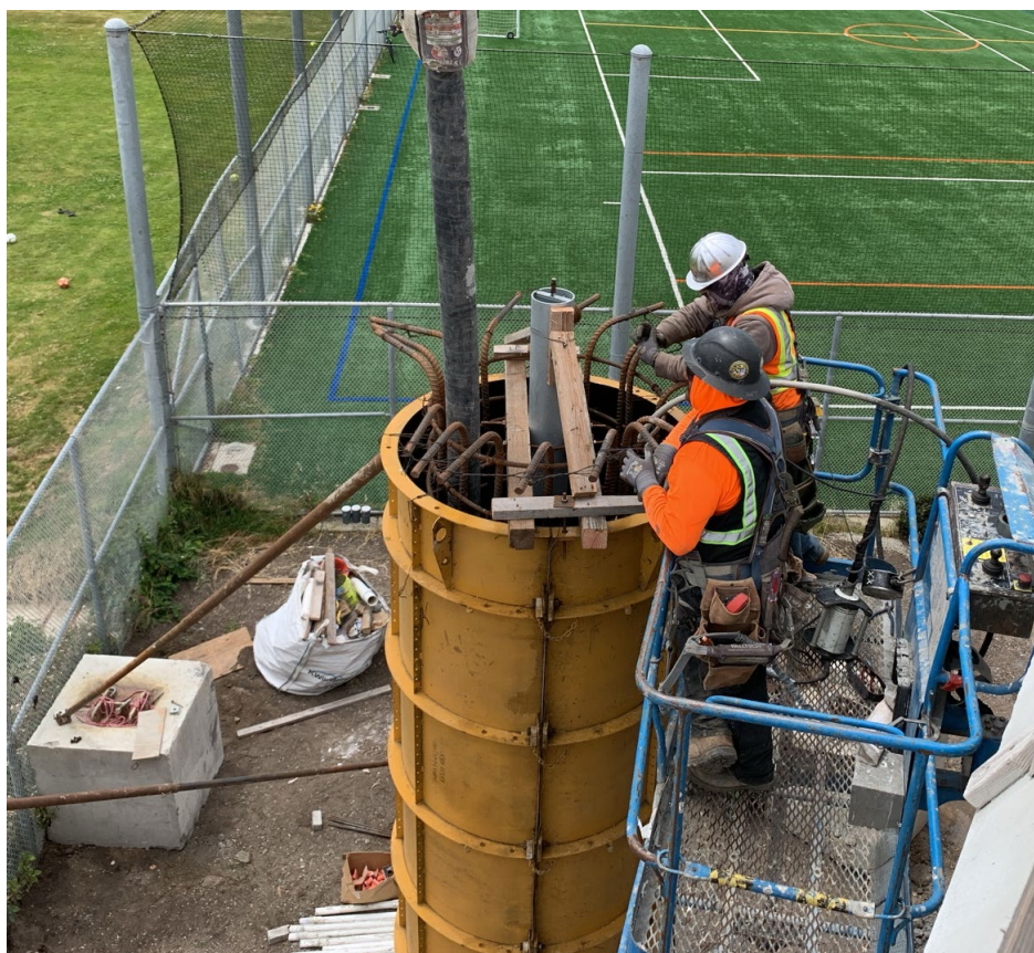
Figure 6-3. Column Concrete Placement
