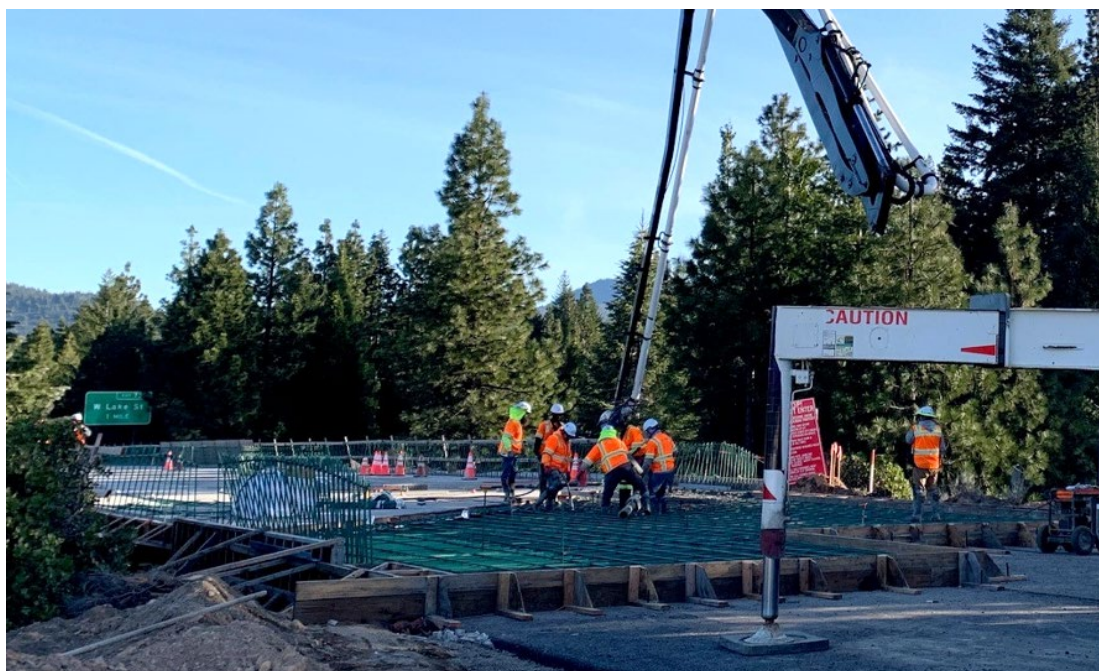
Figure 6-15. Approach Slab Concrete Placement
