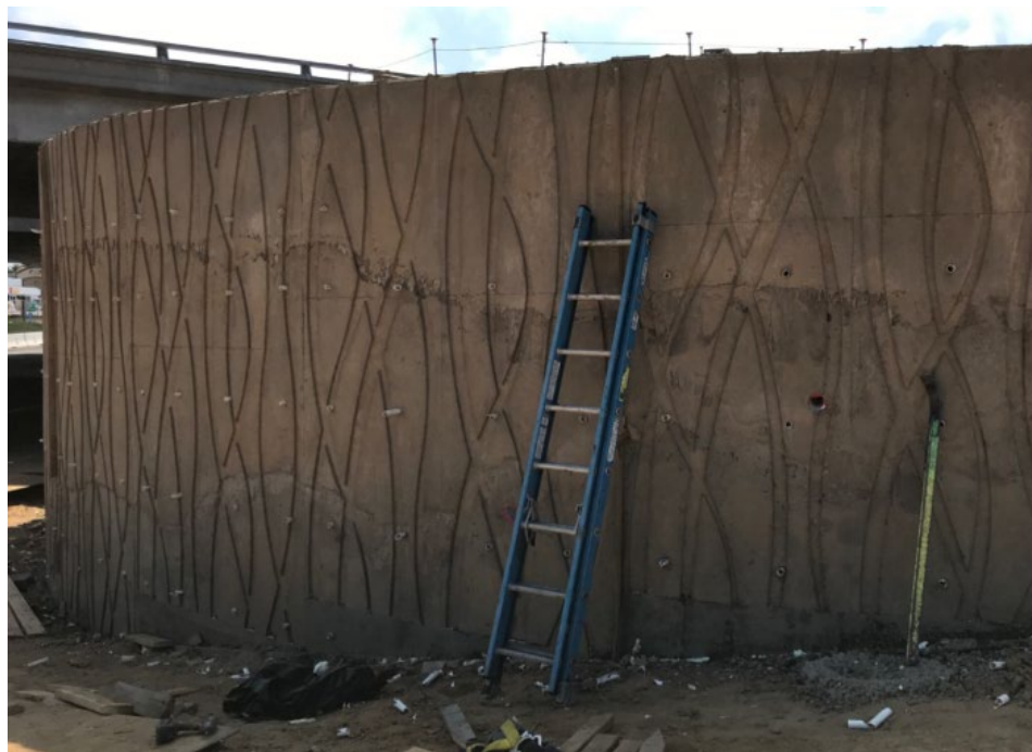
Figure 5-38. Cold Joints on Wall with Architectural Features
