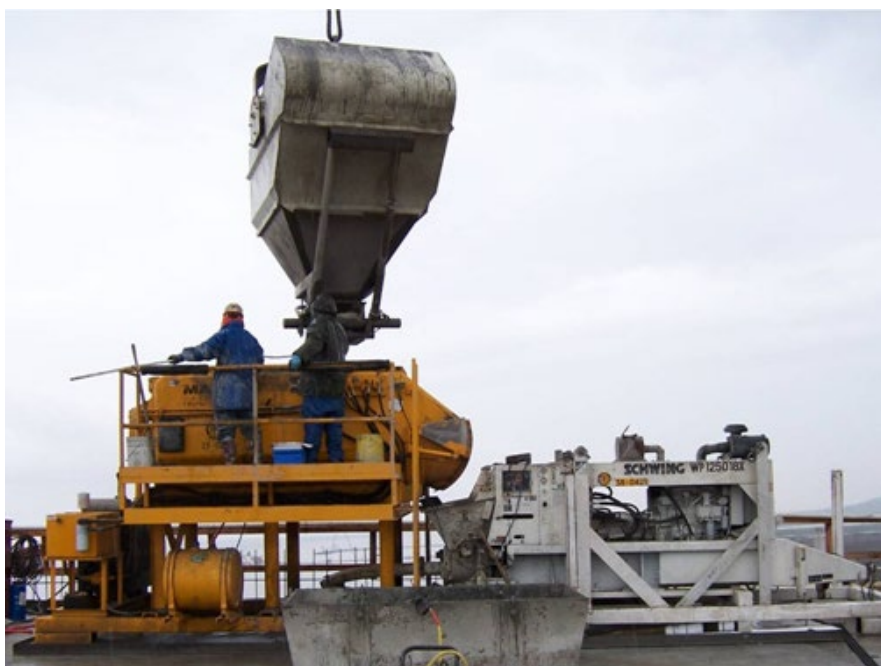
Figure 5-7. High-Capacity Bucket
