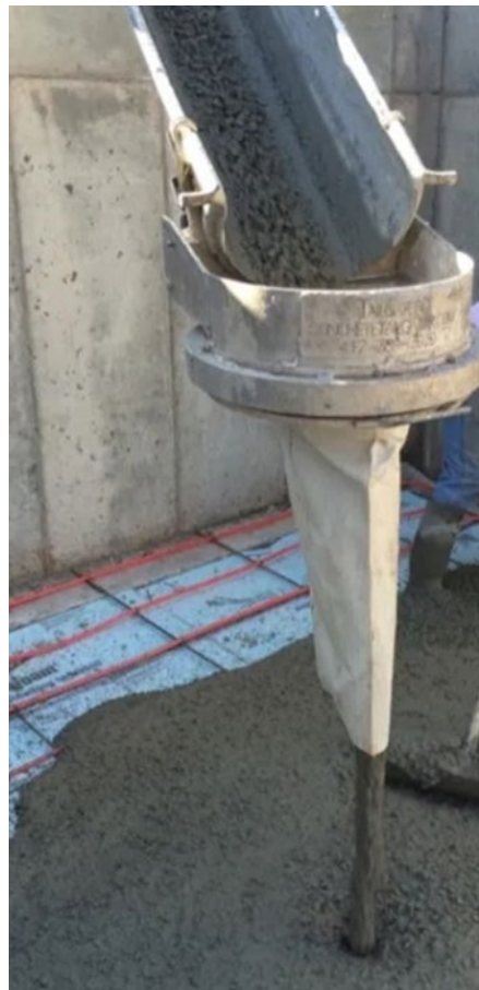
Figure 5-8. Depositing Concrete Using a Drop Chute Attached to a Hopper
