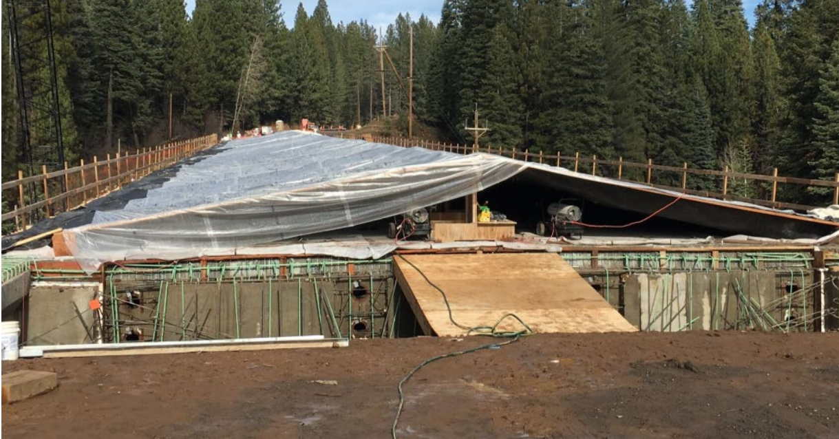
Figure 5-39. Maintaining Concrete Temperature in Cold Weather
