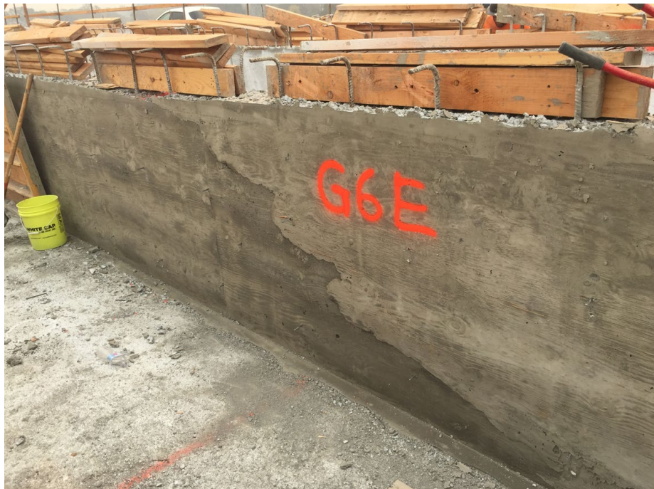
Figure 5-29. Cold Joint
