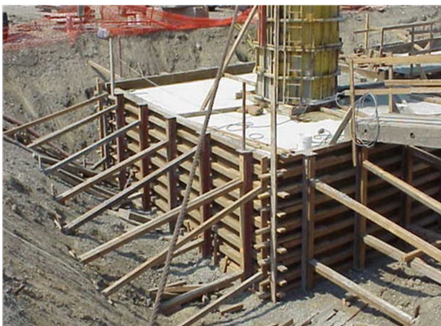
Figure 5-21. Forms-In-Place Curing Method
