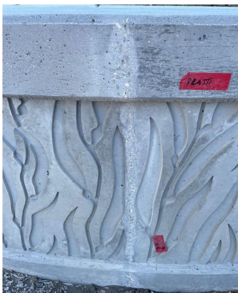
Figure 5-31. Excessive Grinding Exposing Aggregate
