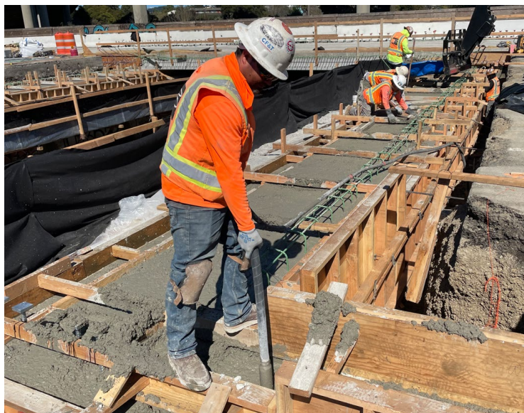
Figure 5-14. Vibrating Using Internal Vibrator
