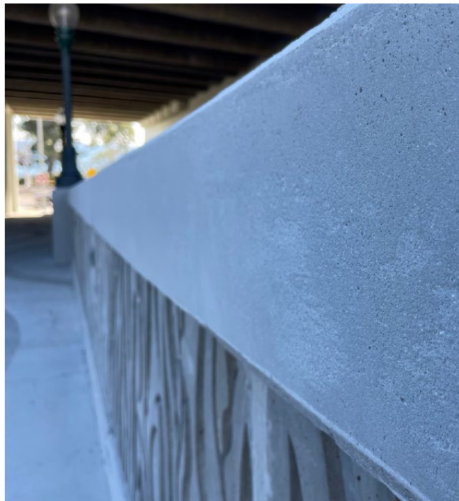
Figure 5-35. Class 2 Surface Finish
