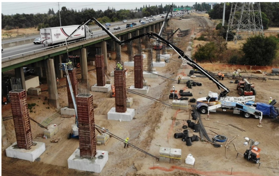
Figure 5-10. Concrete Pump with Extended Boom
