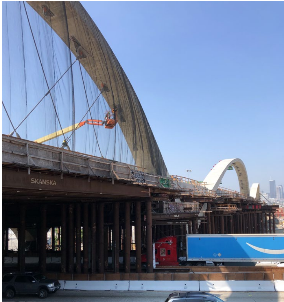
Figure 5-49. Protective Measures over Traffic
