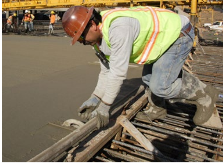
Figure 5-16. Hand Floating
