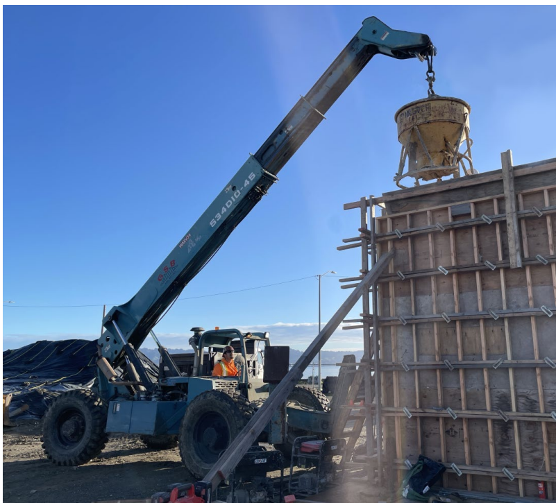
Figure 5-6. Concrete Placement with Bucket and Forklift
