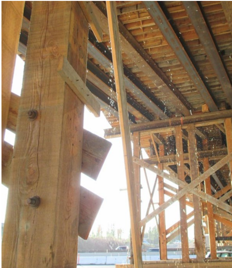
Figure 5-43. Leaking Soffit Forms
