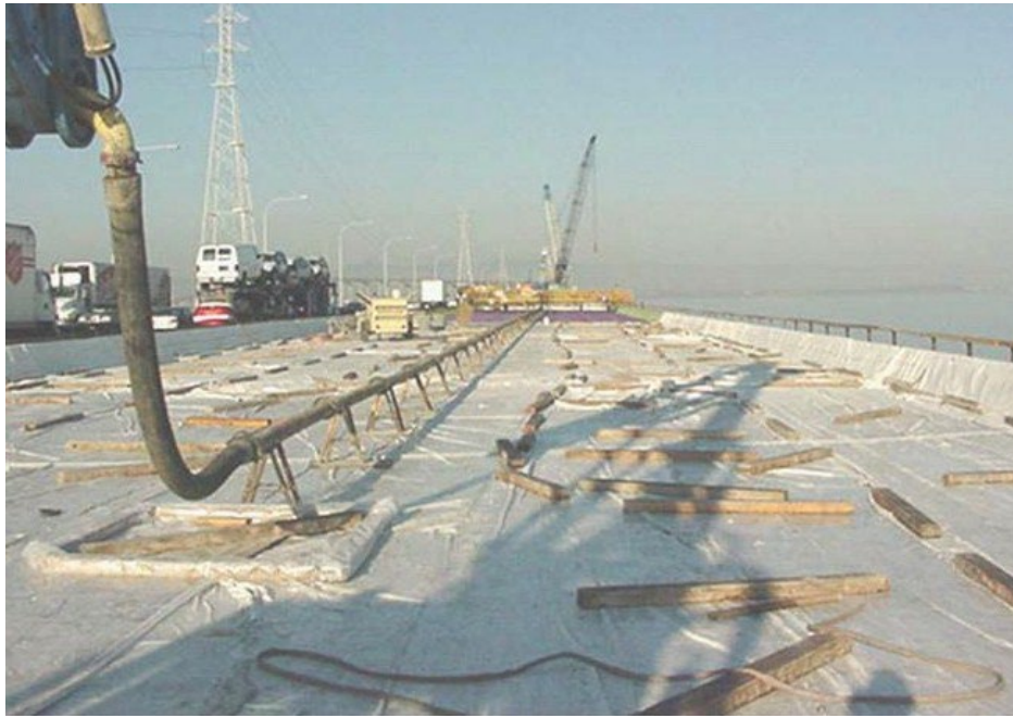
Figure 5-11. Slick Line Used to Deliver Concrete
