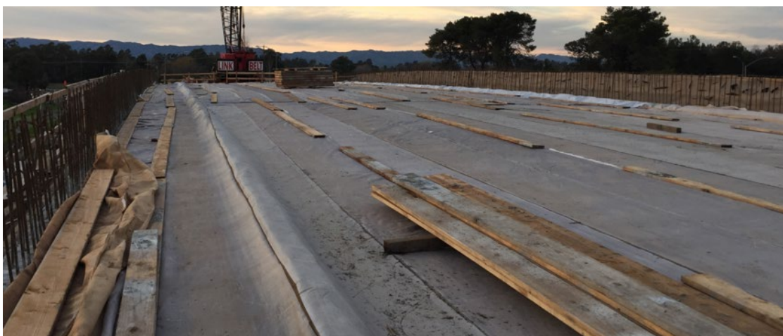
Figure 5-20. Curing with Burlene Curing Blankets
