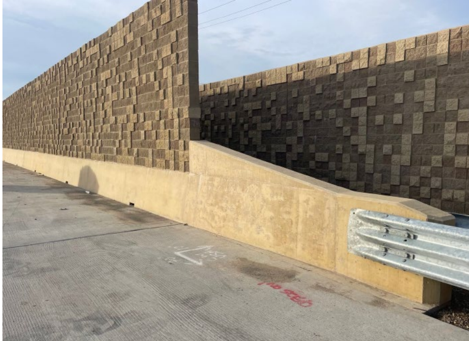
Figure 5-37. Barriers Constructed with Integrally Pigmented Concrete
