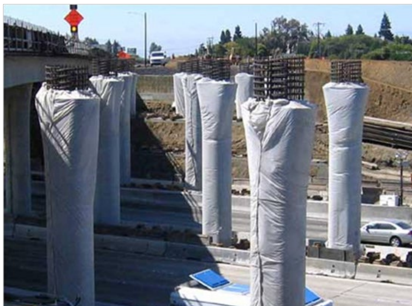
Figure 5-19. Curing Concrete Columns Using Polyethylene Sheets
