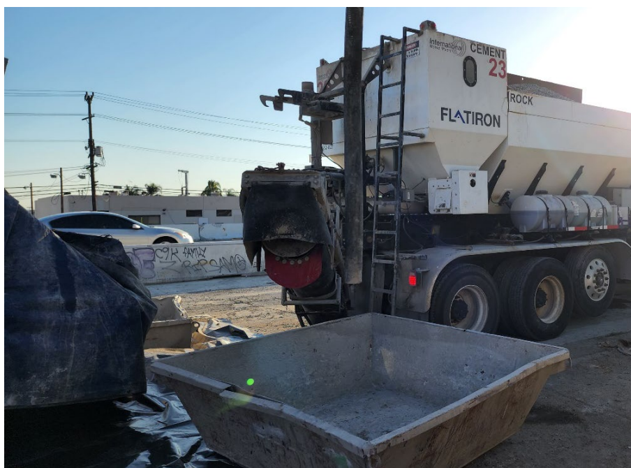
Figure 5-47. Temporary Concrete Washout
