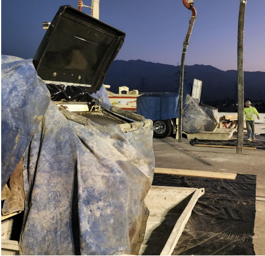
Figure 5-44. Visqueen Protection Under Concrete Pump
