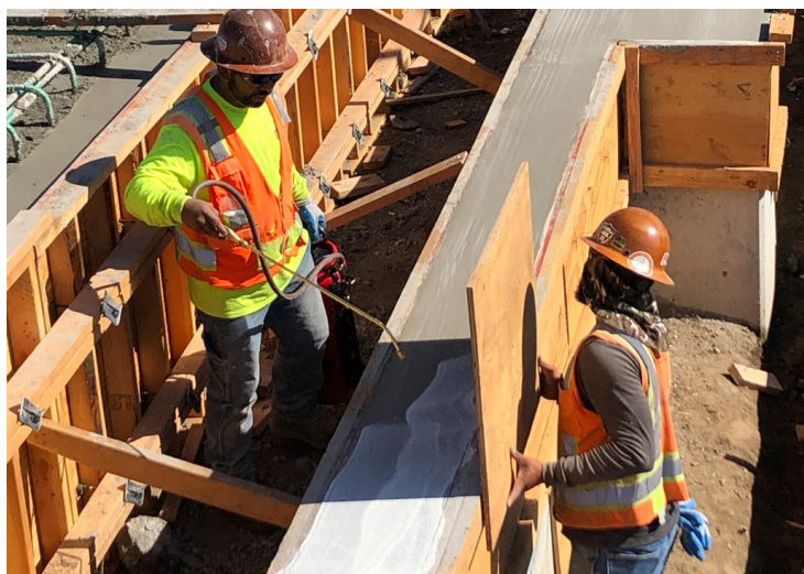
Figure 5-42. Curing Compound Shield
