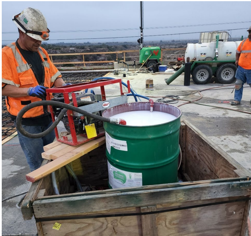
Figure 5-46. Curing Compound Secondary Containment
