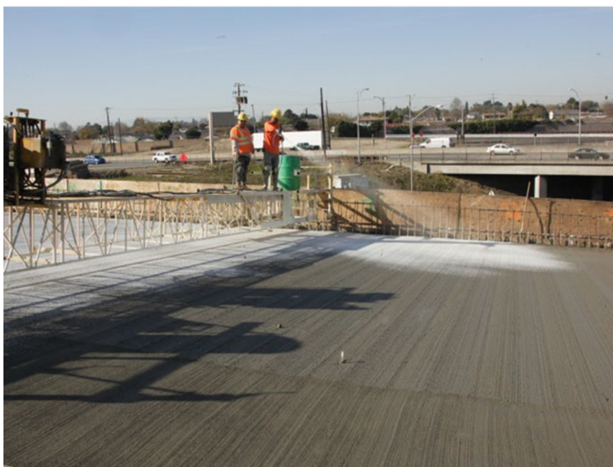
Figure 5-22. Applying Curing Compound Using Power-Operated Spray Equipment
