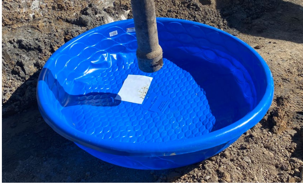
Figure 5-48. Unacceptable Concrete Washout
