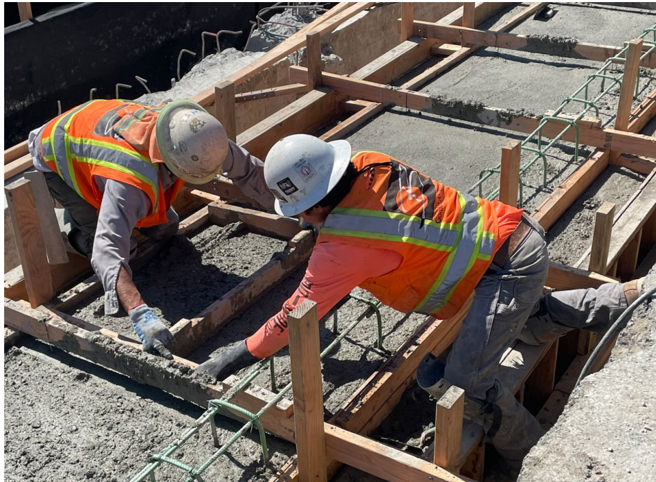
Figure 5-15. Striking Off Concrete
