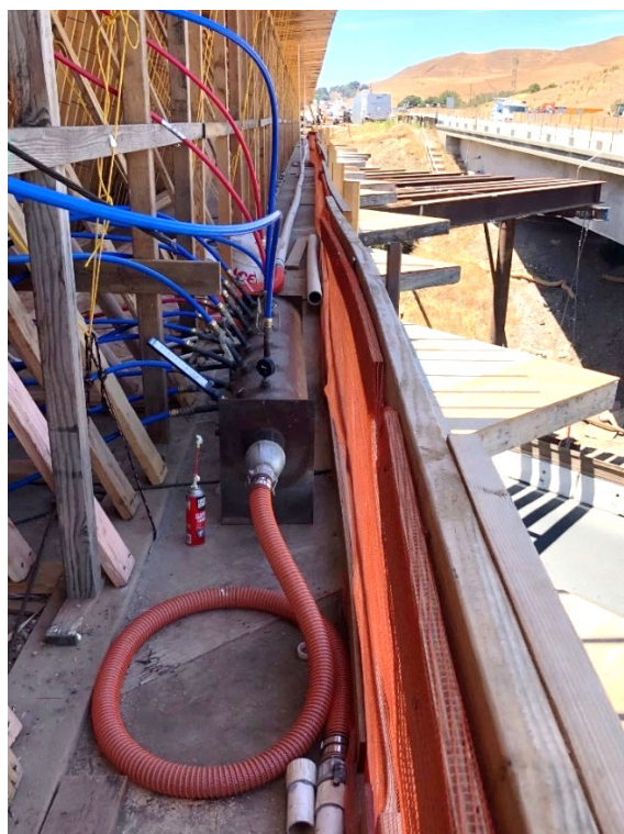
Figure 5-41. Manifold and Cooling Pipes for Mass Concrete Cooling System
