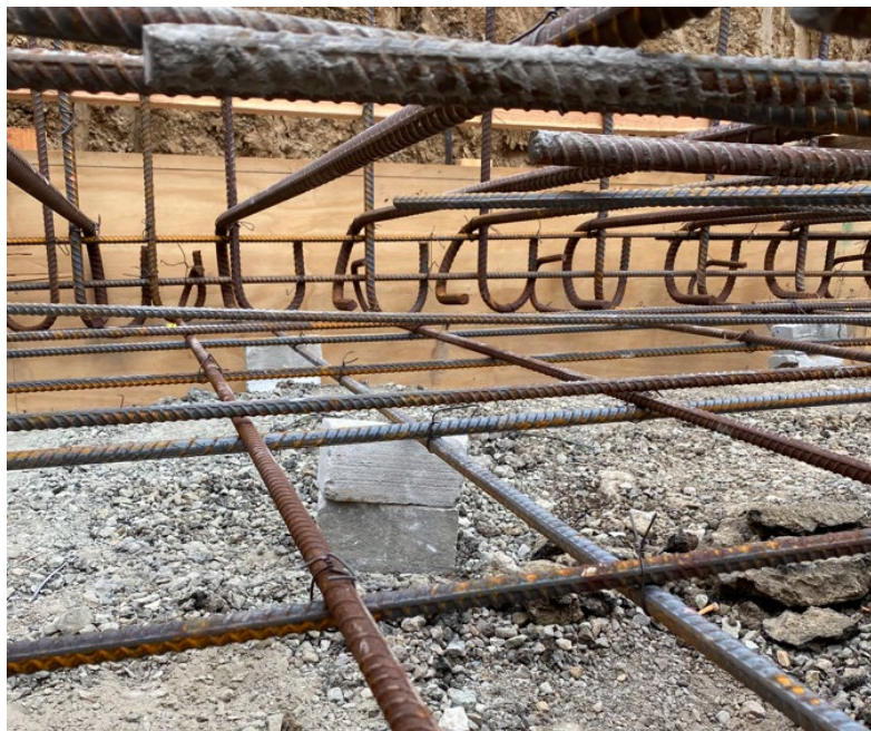
Figure 4-3. Concrete Dobies Under Approach Slab Bottom Mat
