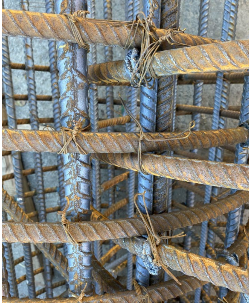
Figure 4-4. Column Reinforcement Ties
