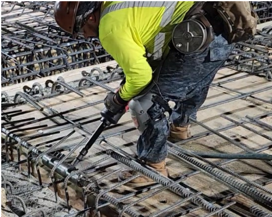
Figure 4-14. Sleeve-Lock Shear Bolt Mechanical Coupler Installation
