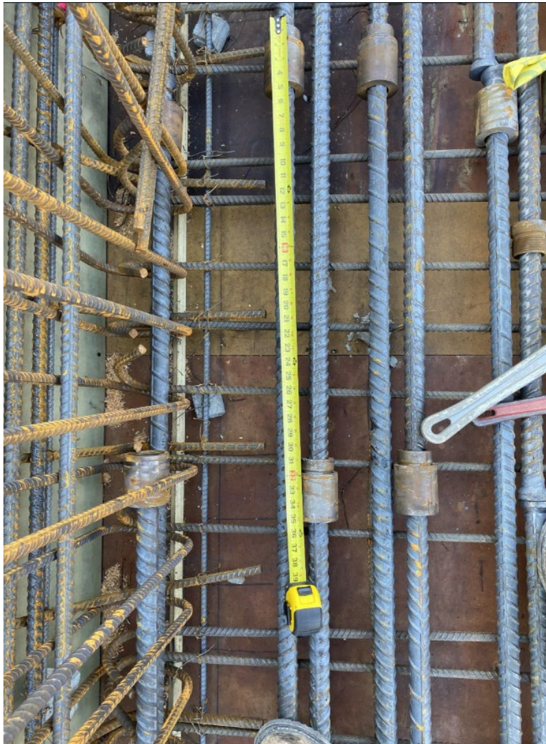
Figure 4-13. Staggered Splices with Couplers
