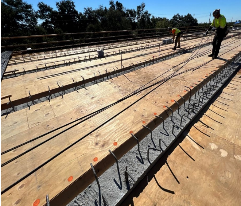
Figure 4-2. Bar Reinforcement Layout
