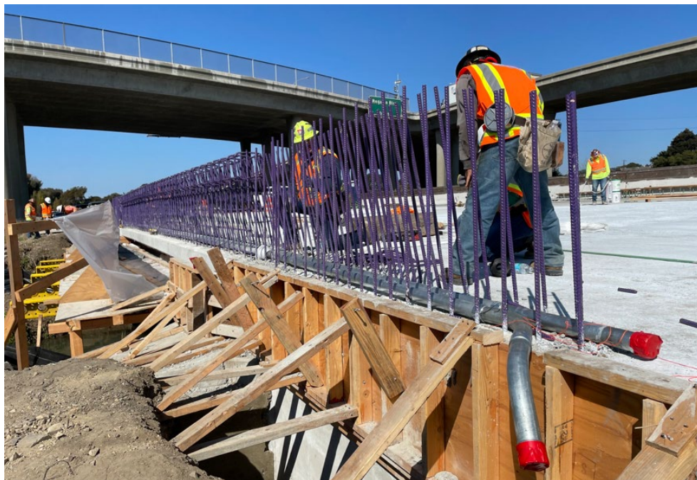
Figure 4-10. Epoxy Coated Prefabricated Reinforcement (Purple)
