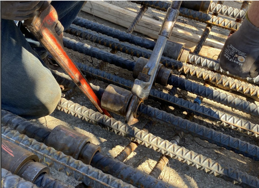
Figure 4-15. Two Piece Sleeve/Forged End Mechanical Coupler Installation
