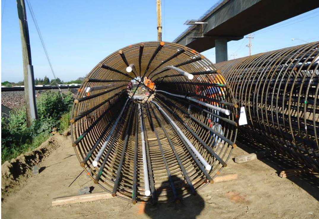
Figure 4-7. Bar Reinforcement Cage Laid on its Side
