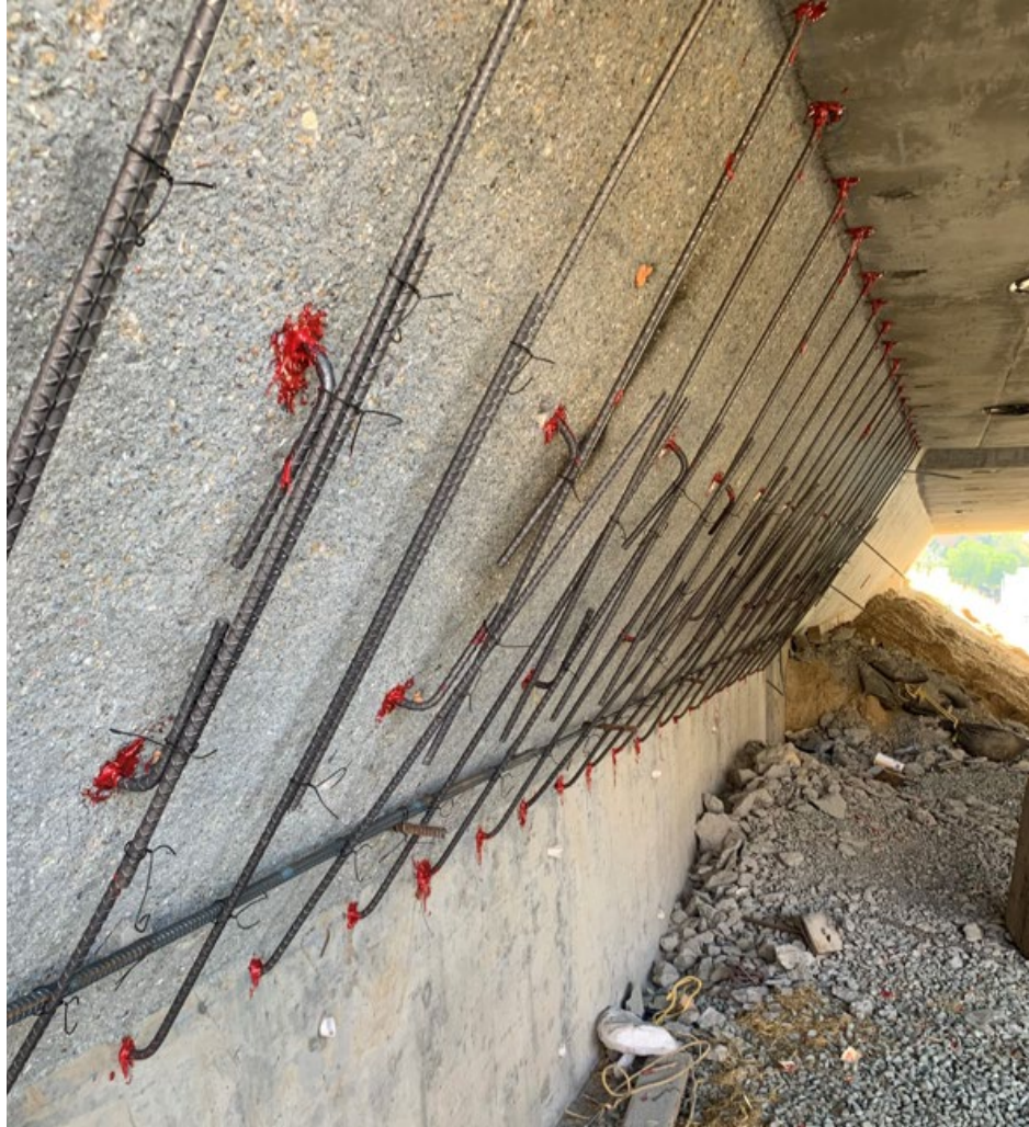
Figure 4-22. Drill and Bond Dowel – Chemical Adhesive
