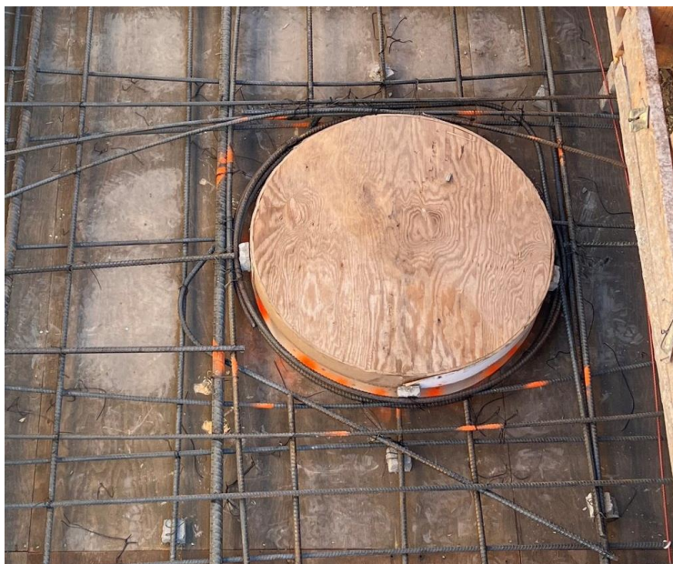
Figure 2-1. Blockout for Soffit Access Opening
