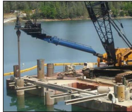
Figure 6-16. Crane Mounted Drill Rig.
