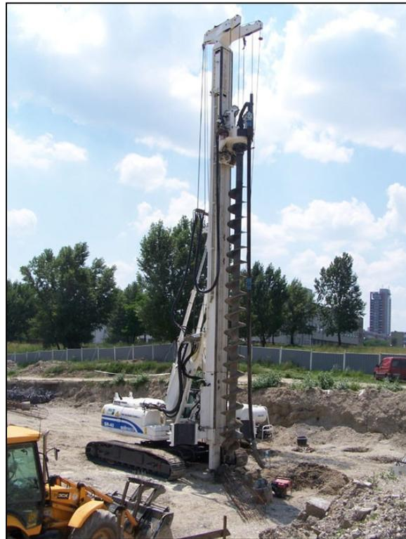
Figure 6-2. Continuous Flight Auger.
