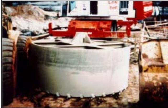
Figure 6-8. Core Barrel.
