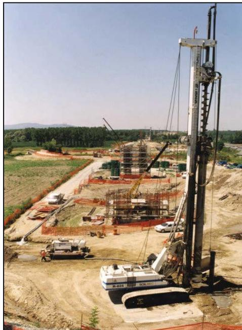
**Figure 6-14. Crawler Mounted Drill Rig.**
