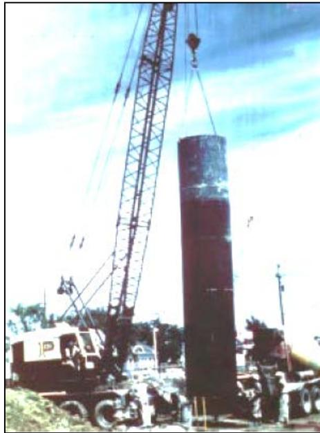
**Figure 6-13. Steel Casing.**
