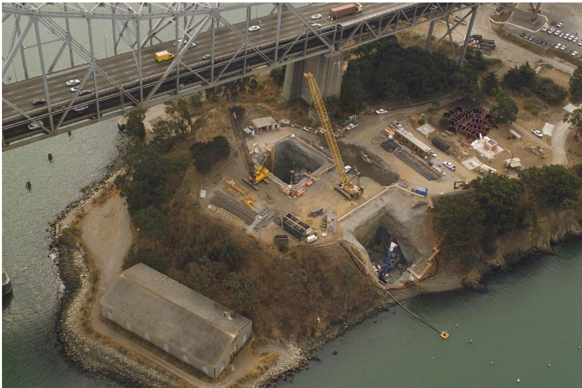
Figure D-2. SFOBB East Span Pier W2 Footing Excavations.
