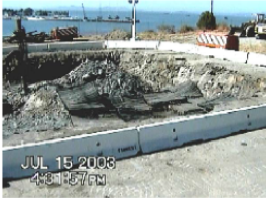
Photo 1. Pier W2. Before detonation. Blasting mats on top.
