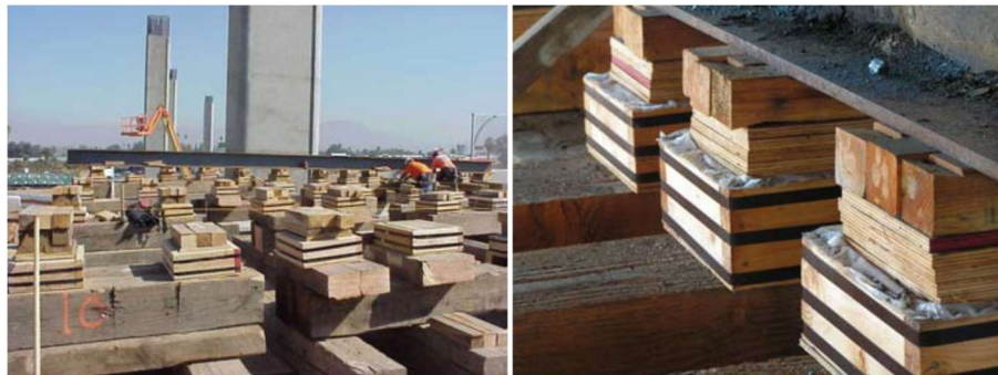
Figure 9-1. Wood Sand Jacks.
