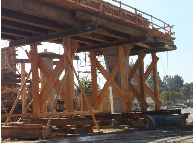
Figure 1-1. Common Falsework System
