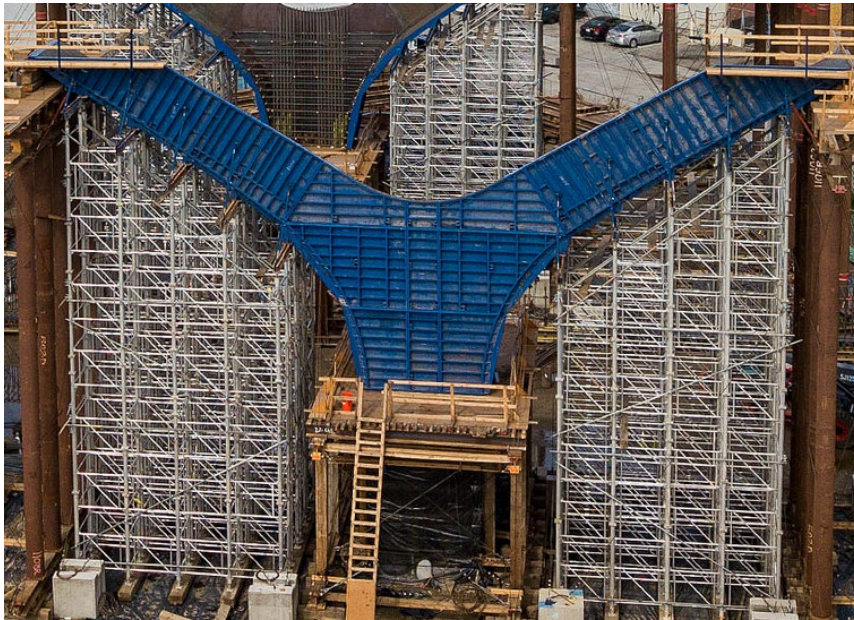
Figure 1-3. Proprietary Shoring System
