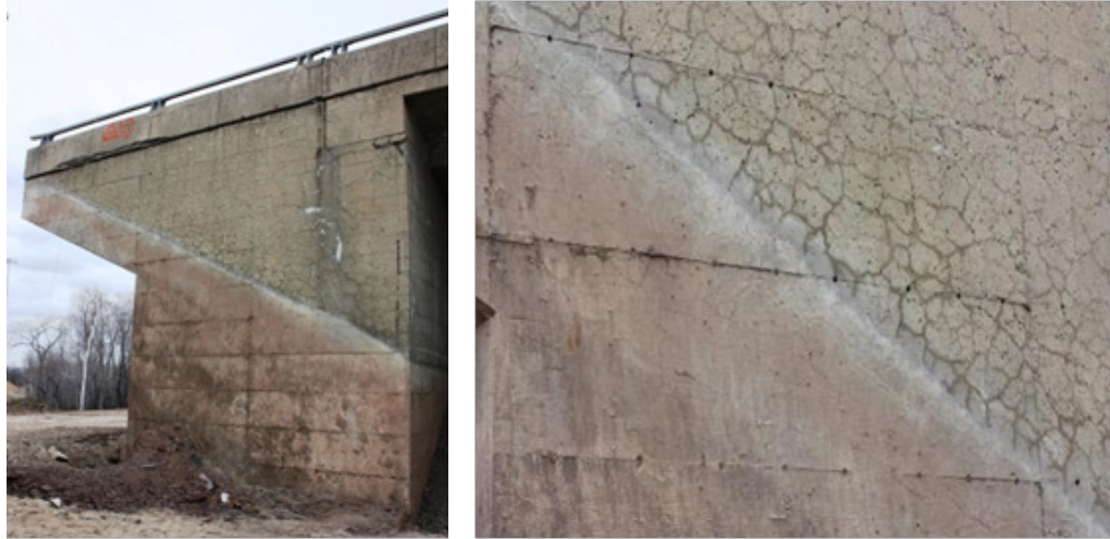
Figure 1-7. Concrete Deterioration Due to Alkali-Silica Reaction 4 .
