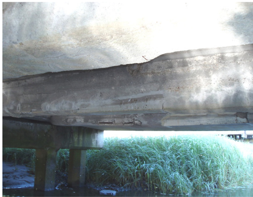
Figure 1-5. Corrosive Girder Spalling.
