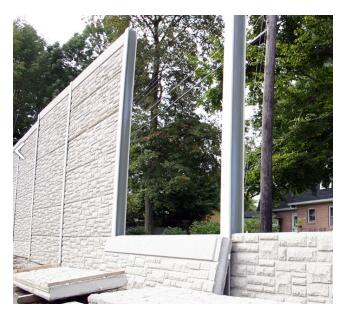
Figure 3. Example of Precast Sound Wall in Construction
