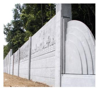
Figure 4. Example of a Constructed Precast Sound Wall
