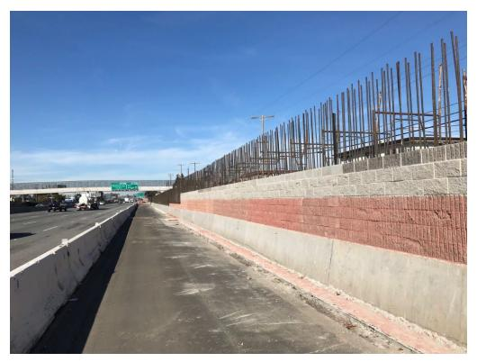
Figure 2. Masonry Block Sound Wall in San Mateo, CA on Hwy 101, EA 04-1J5694
