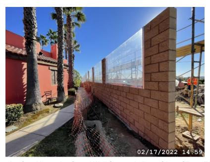
Figure 5. Sample of an Alternative Sound Wall System in Brea, CA on SR 57, EA 12-0C1104
