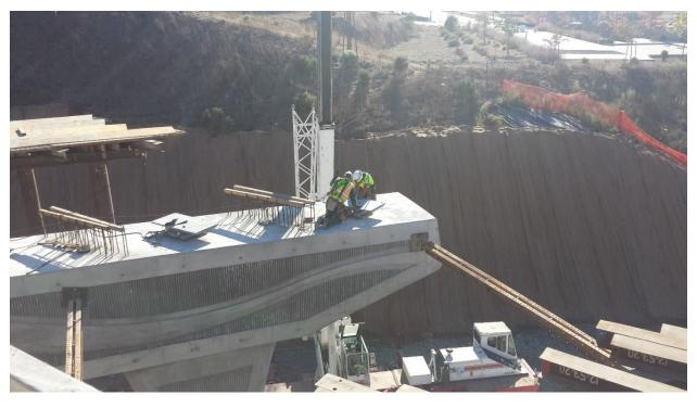
Figure 3. Installation of PTFE Spherical Bearings (Petaluma River Bridge Project)
