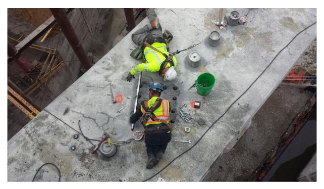
Figure 2. Lug Installation and Checking the Level of the Concrete Surface to Receive the PTFE Spherical Bearing (Petaluma River Bridge Project)
