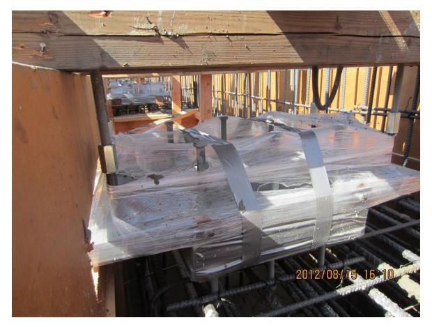
Figure 1. Protective Measures Taken to Protect the PTFE from Concrete Intrusion During Concrete Placement (SFOBB Touchdown Project)
