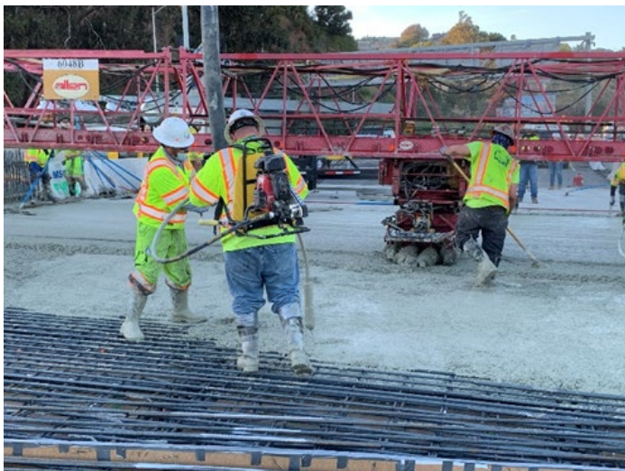
Figure 5. Placing concrete and an up-close view of concrete mix
