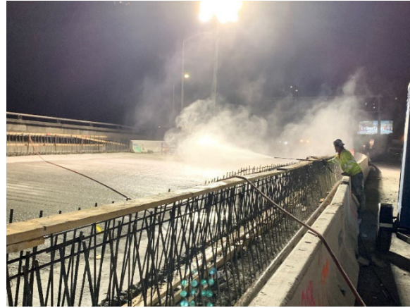
Figure 6. Spray misting top of concrete
