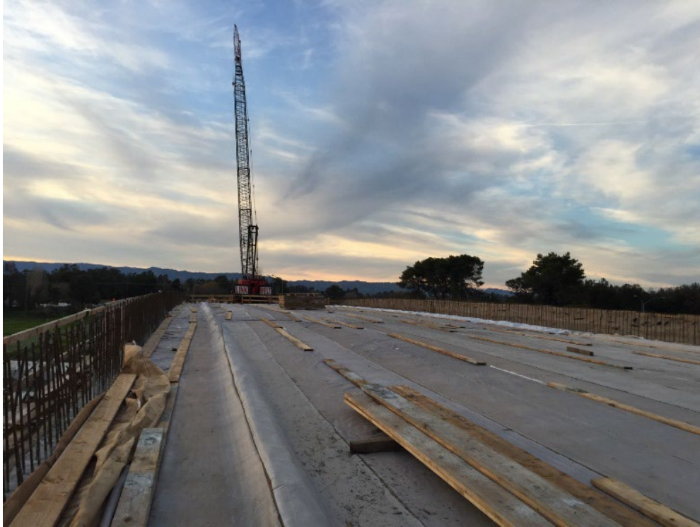
Figure 8. Continue water method curing for 7 days
