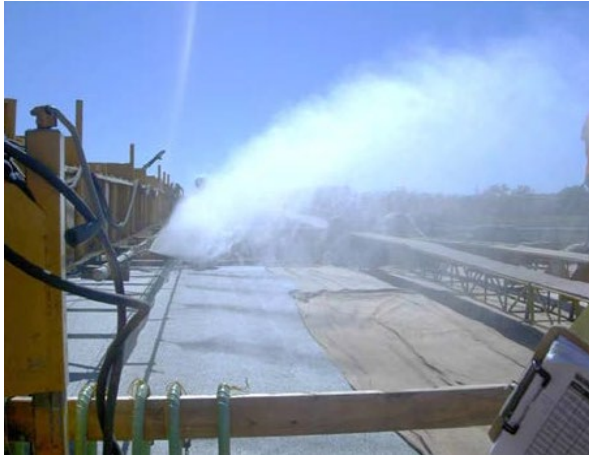
Figure 7. Continue misting while curing medium for water method is placed
