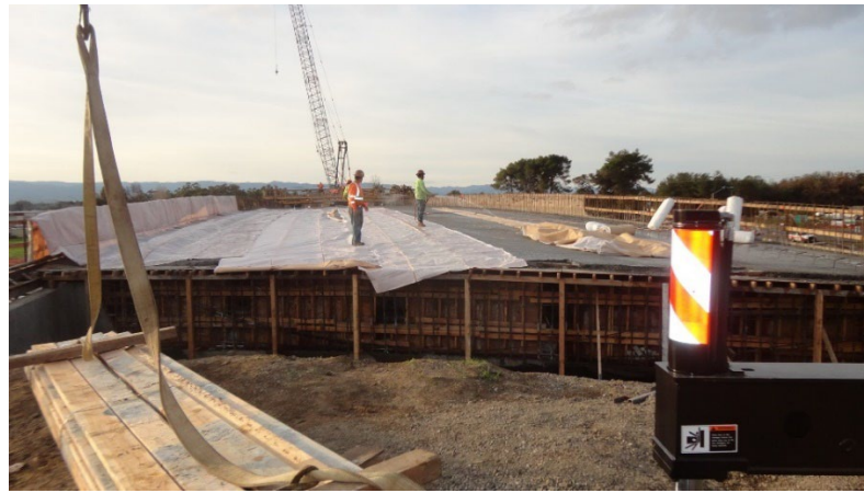
Figure 7. Continue misting while curing medium for water method is placed
