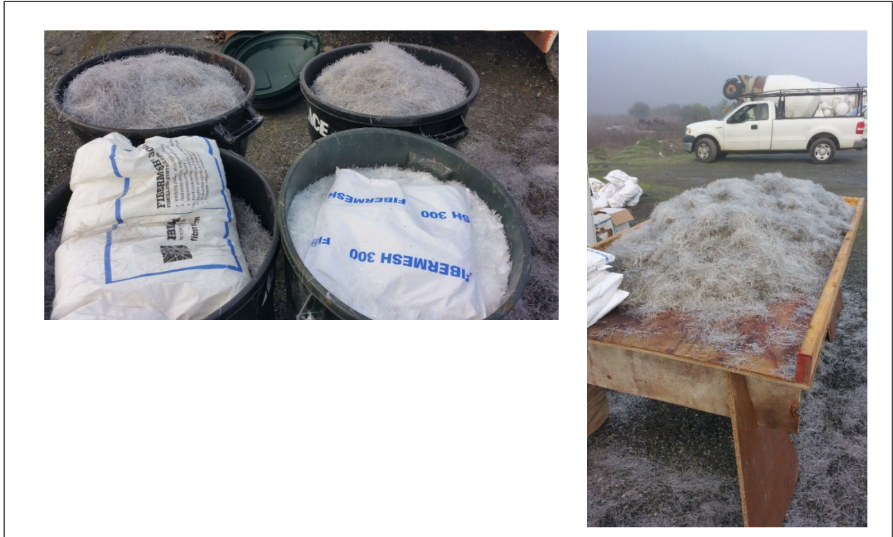
Figure 3. Polymer Fibers on the Jobsite
