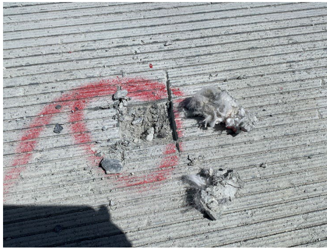
Figure 10. Clumps of unmixed fiber before and after grinding and grooving the deck.
