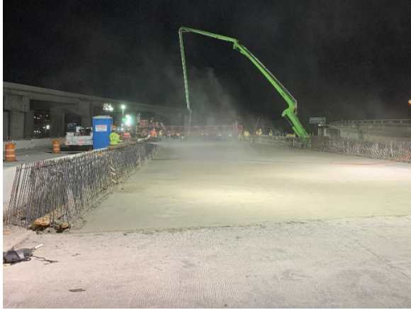
Figure 6. Spray misting top of concrete
