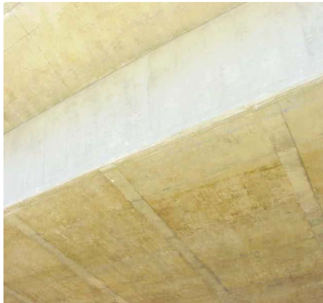
Figure 3. Form Filler Strip of Plywood
