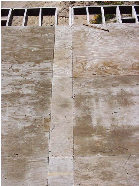
Figure 2. Typical Gang Form
