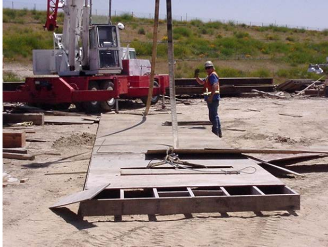
Figure 1. Typical Gang Form
