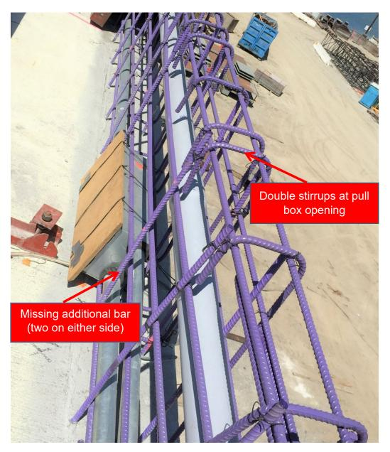
Figure 2. Additional Rebar at Pull Box Location
