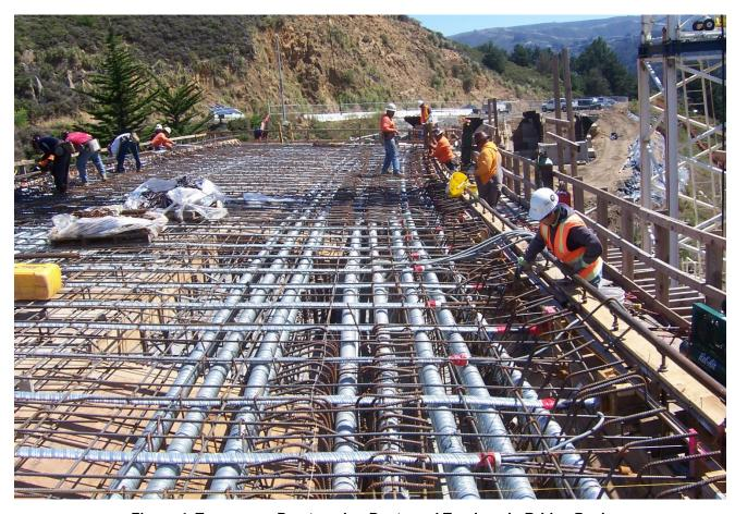
Figure 4. Transverse Prestressing Ducts and Tendons in Bridge Deck
