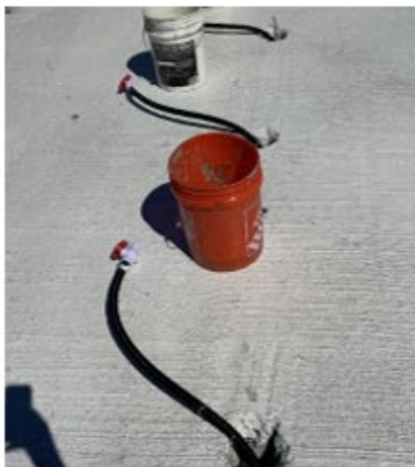
When grouting, buckets are placed at every grout tube on the deck for overflow. When grout flows out at a consistent viscosity, valves are shut. Verify availability of concrete washout prior to grouting operation.
