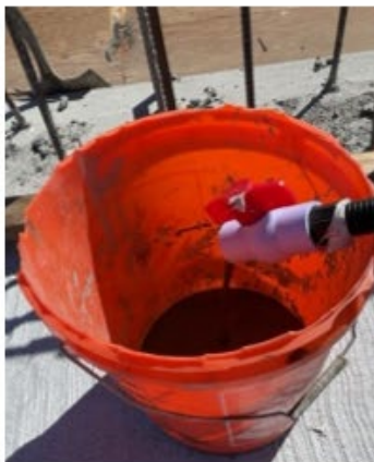
When grouting, buckets are placed at every grout tube on the deck for overflow. When grout flows out at a consistent viscosity, valves are shut. Verify availability of concrete washout prior to grouting operation.
