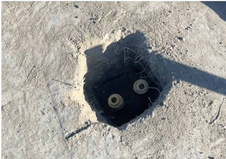
High-point grout vents (to be removed and patched after grouting tendons).
