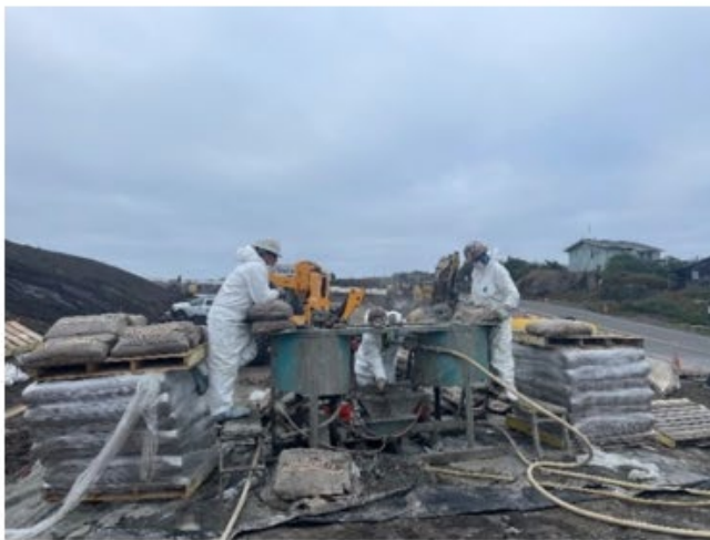
Grouting operation and apparatus for CT 541.
