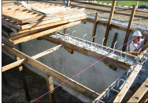
Figure 2.1-11. A String-Line Strung Between Deck Dowels.
