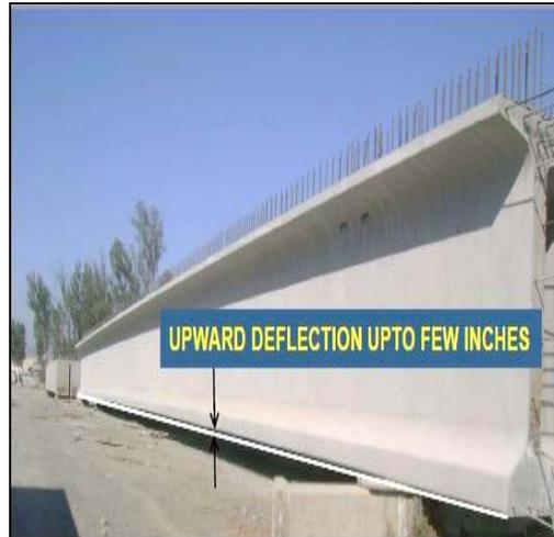
**Figure 4.1-3. Measuring for Precast, Prestressed “I” Girder Camber.**
