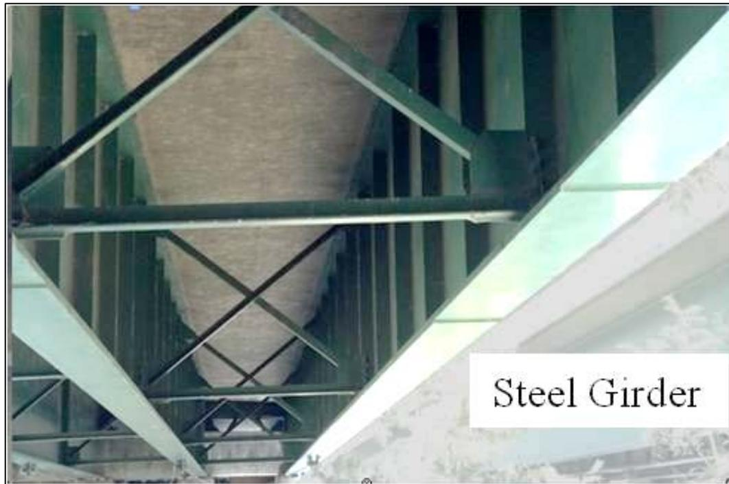
Figure 2.1-5. Example of a Steel-Girder Bridge.
