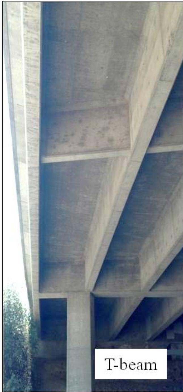
Figure 2.1-6. Example of a T-Beam Bridge.
