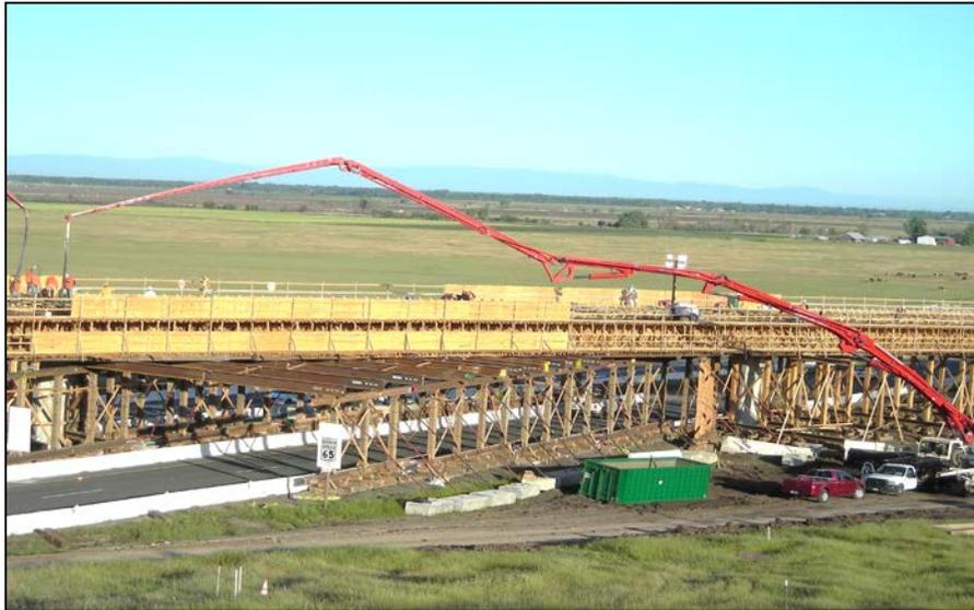
**Figure 5.2-2 Concrete Pump.**
