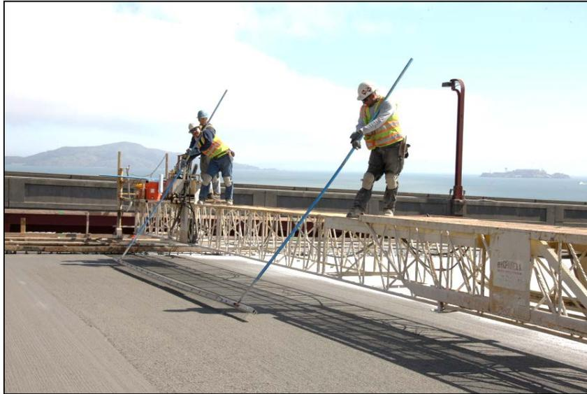
**Figure 6.1-6. Longitudinal Tining Typical Process.**
