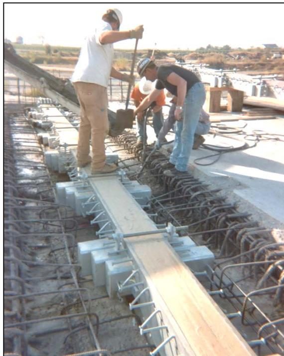
Figure 2.2-3. Threaded Spacer Rods Used to Hold the Correct Width.
