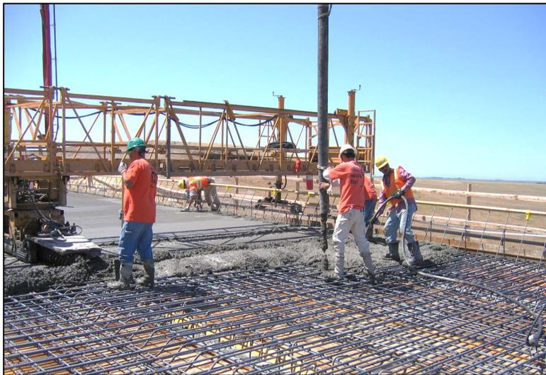
**Figure 5.3-1. Vibrating Concrete.**
