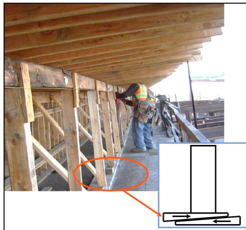
**Figure 4.2-1. Wedge System for the Overhang.**
