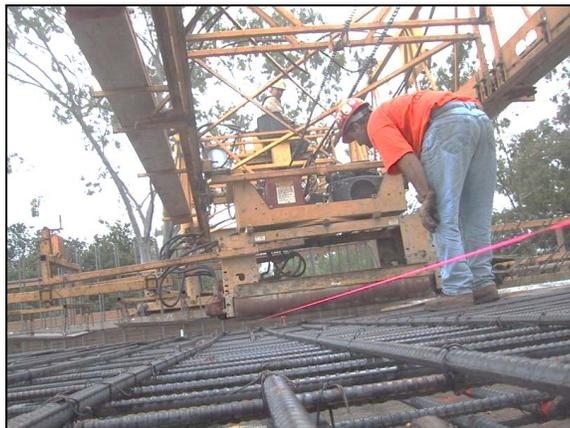
**Figure 4.2-5. Check Finishing Machine Height.**
