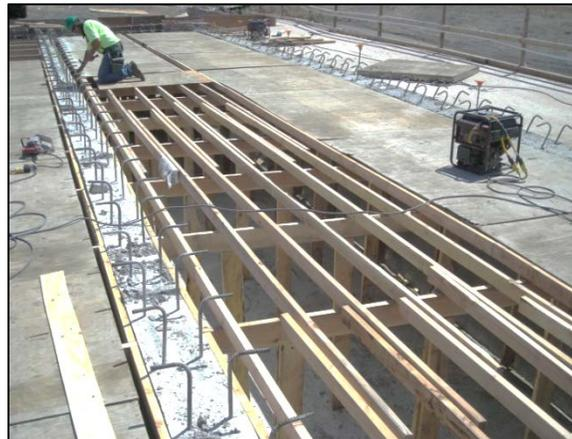
**Figure 2.1-2. Typical Deck Sheathing Supports on a Concrete Box Girder Bridge.**
