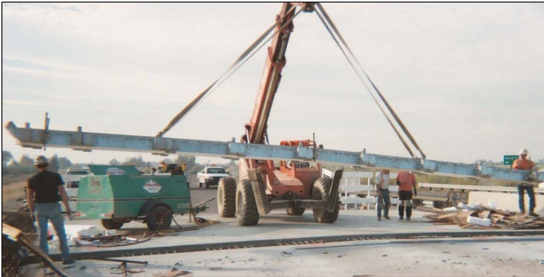
**Figure 2.2-4. Joint Seal Assembly Installation.**
