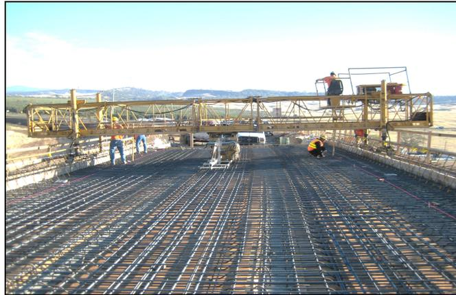
**Figure 4.2-4. Inspect Adjustment of the Finishing Machine.**
