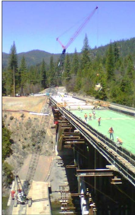
Figure 5.2-1. Crane and Bucket Concrete Placement.
