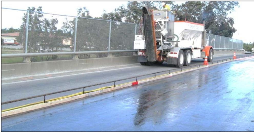
**Figure 6.1-4. Typical Grade Rail Setup.**
