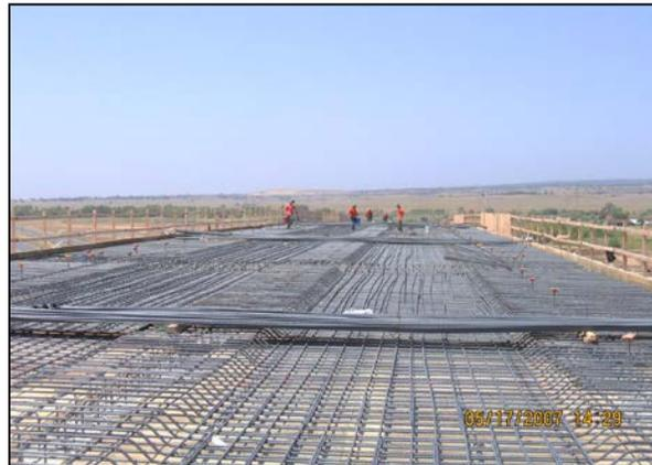
**Figure 3.2-2. Truss Bars Must Not be Allowed to Rotate out of Vertical.**
