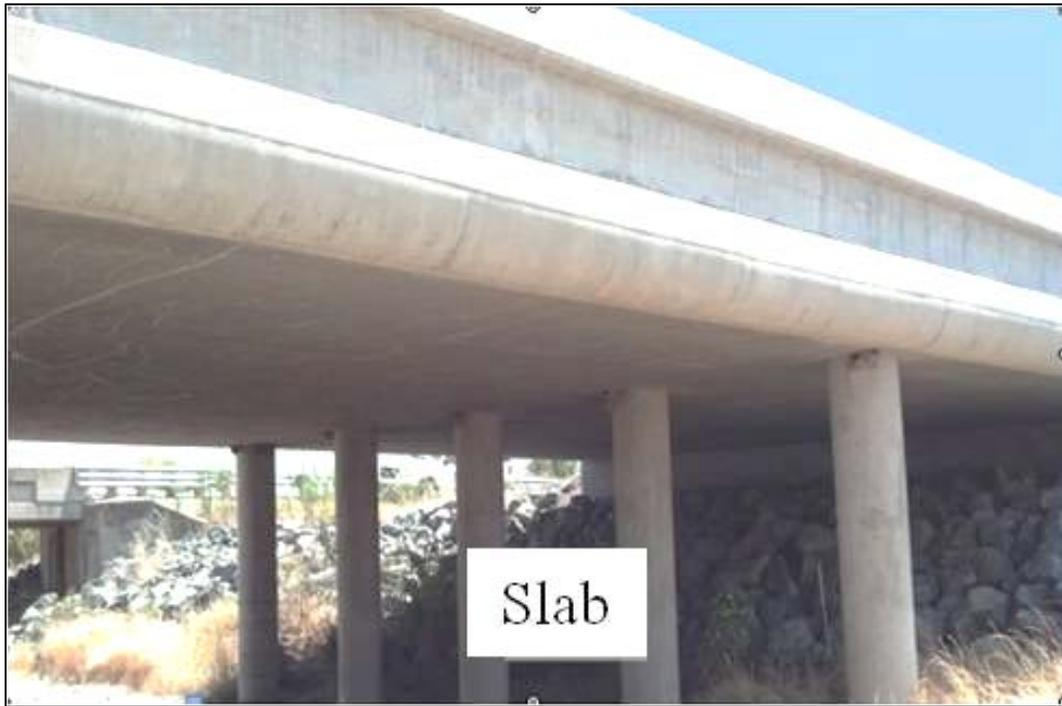
Figure 2.1-4. Example of a Slab Bridge.
