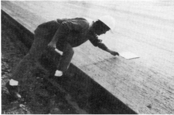
FIGURE 1. Placing Test Pads on Pavement
