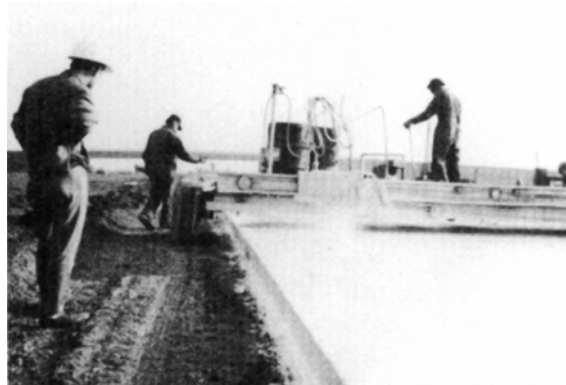
FIGURE 3. Spray Equipment Passing Over Test Pads
