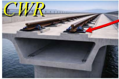
Rail- A continuous Beam on Discrete Nonlinear Springs
