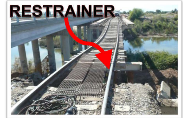
RAIL BRIDGES: Bridge to protect the Restrainer (Rail)
