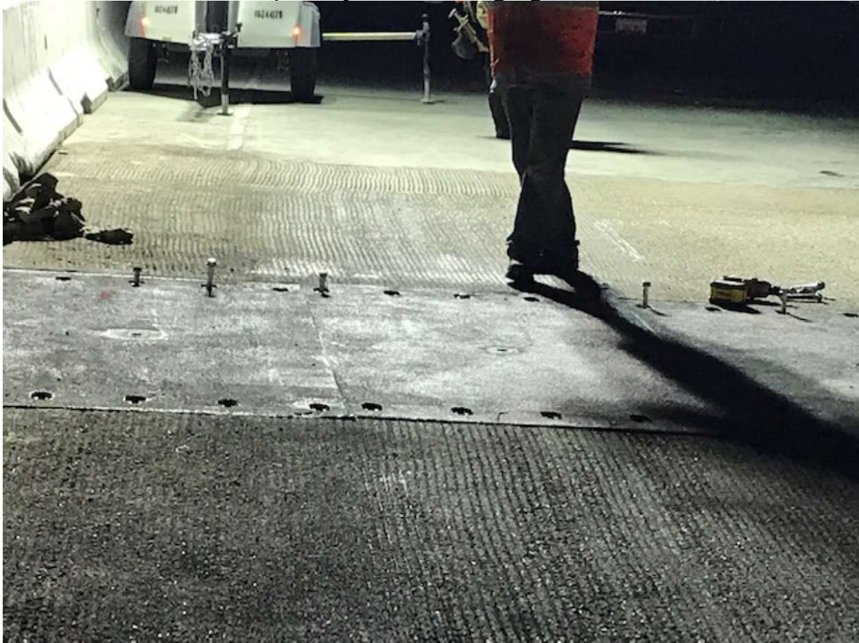
Figure 3: Anchor bolt installation.
