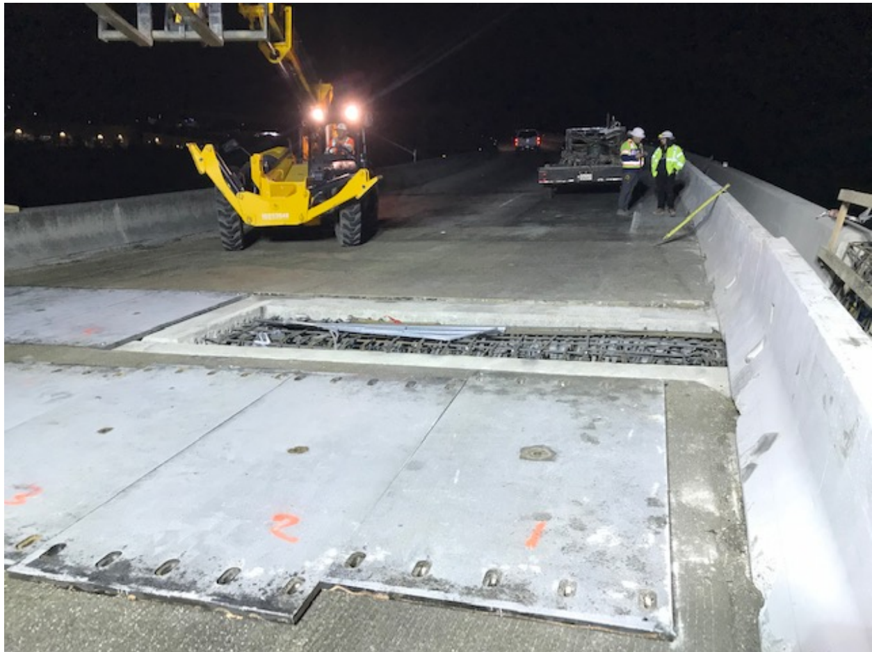
Figure 1: Hinge Bearing Replacement.
