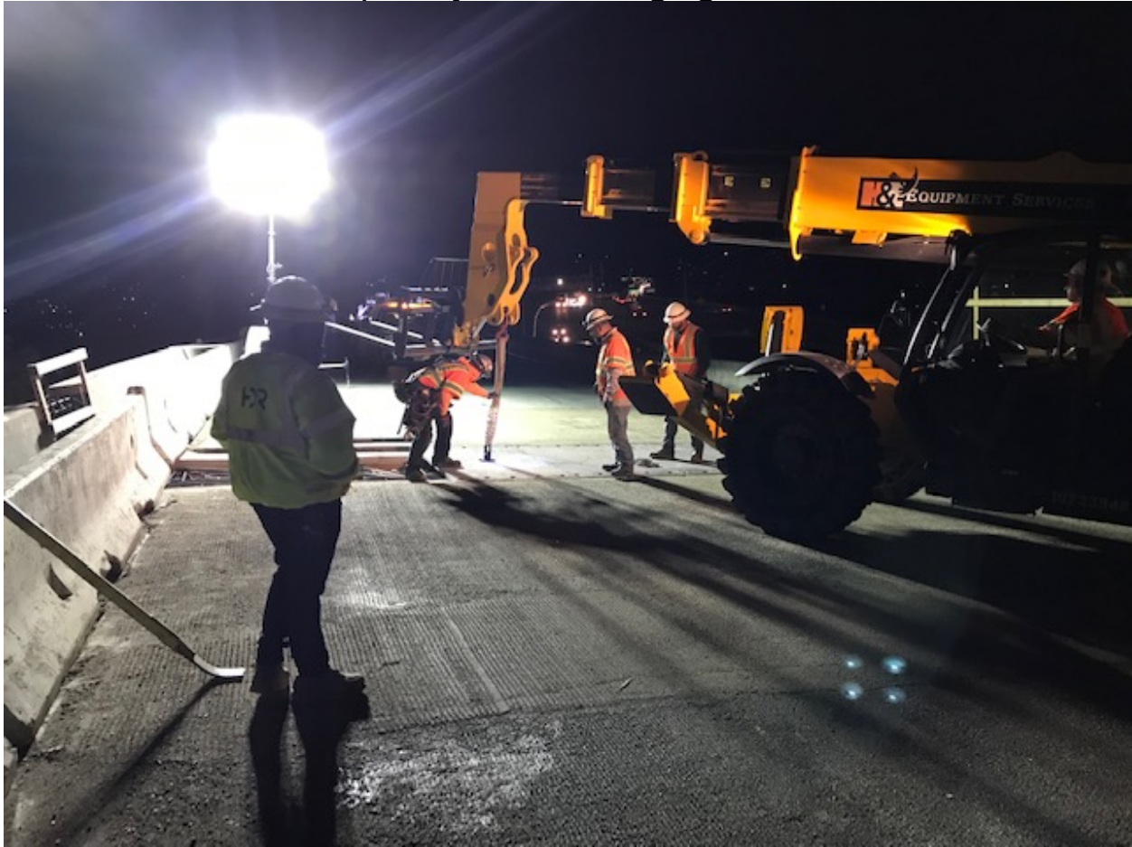
Figure 2: Note polyester concrete taper in foreground.
