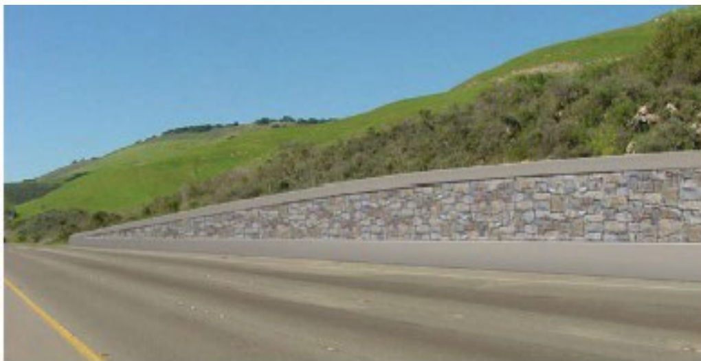
Figure 2.8.4-3 Undesirable Wall Profile
