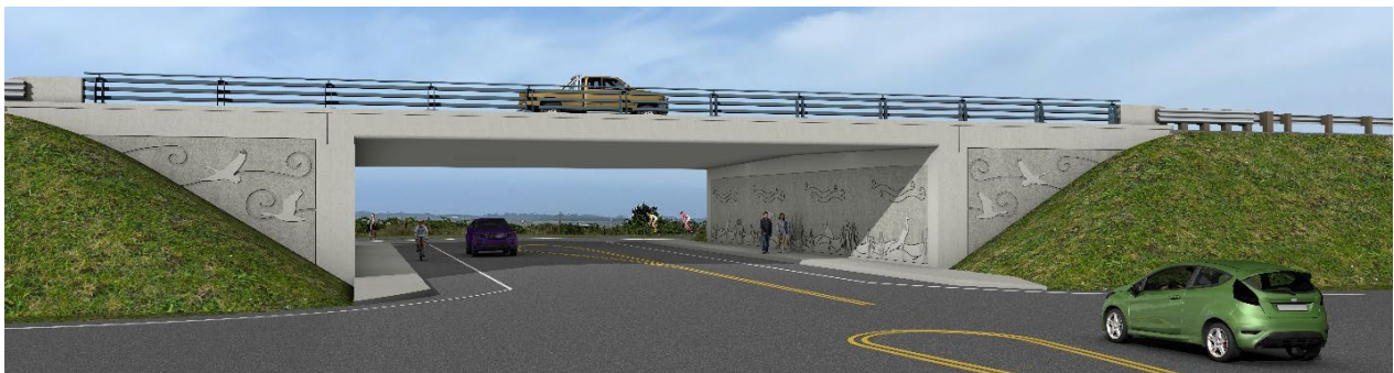
Figure 2.8.3.5-2a Closed-End Abutment
