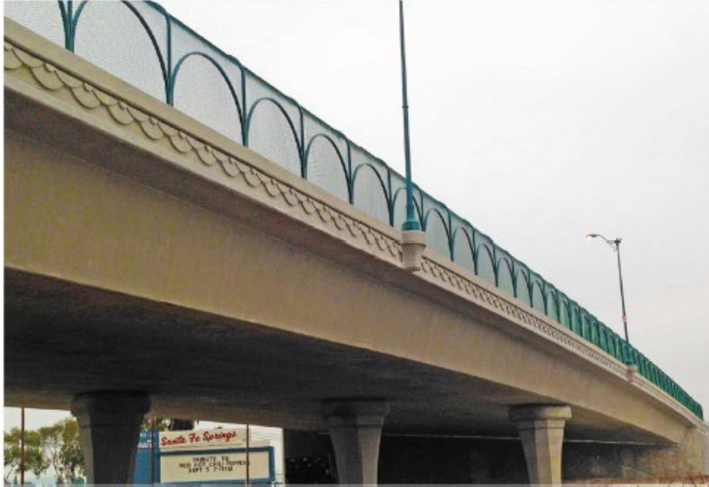
Figure 2.8.3.8-7 Treated Modified Type 6 Steel Chain Link Railing
