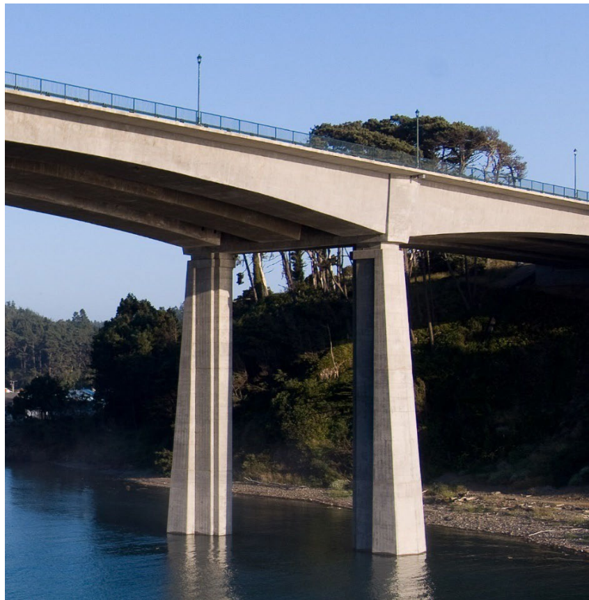
Figure 2.8.3.4.4 Non-Standard Column Type – Noyo Bridge Route 1
