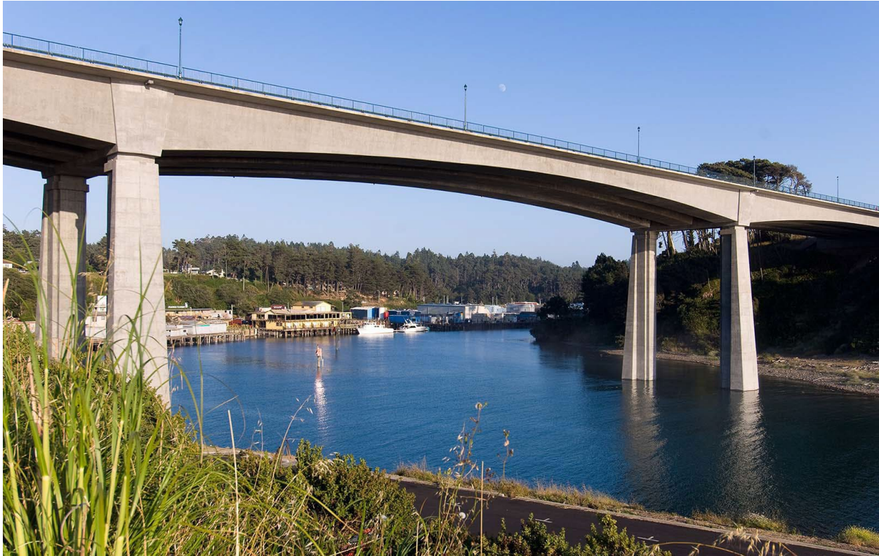
Figure 2.8.3-1 Noyo Bridge Route 1
