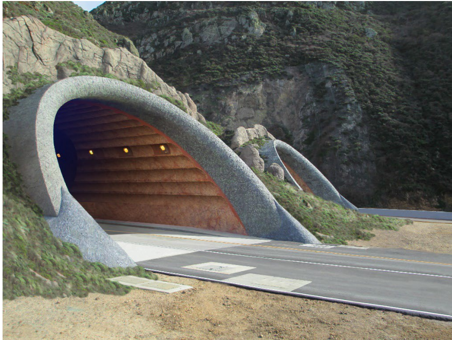
Figure 2.8.7-1 PCH RTE 1 Devil's Slide South Portals
