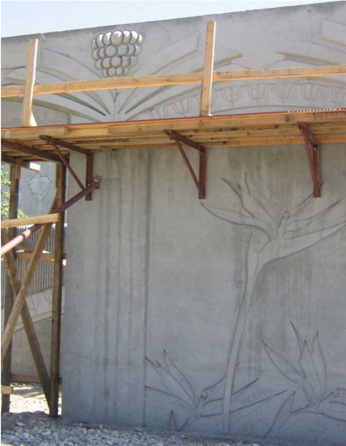
Figure 2.8.9.2-3 Full Height Test Panel Example
