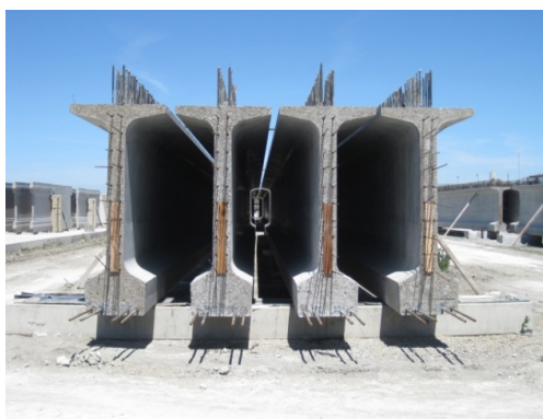
A) Pretensioned bulb-tee girders
