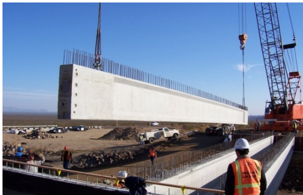
Figure 5.3.3-1 Single-Span I Beam Lowered onto Abutments at Mustang Wash Bridge (Bridge No. 54-1279L, Caltrans)
