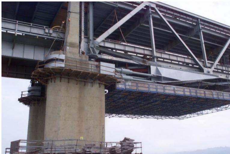
**Figure 20.2.8-53 Seismic Isolation Bearings and Viscous Dampers**
