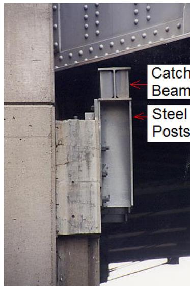
**Figure 20.2.8-4 Catchers for Steel Girder Bridge**
