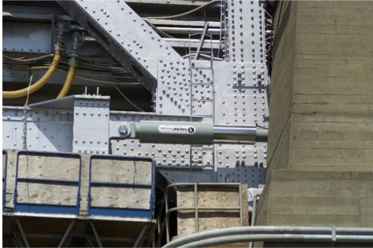
**Figure 20.2.8-68 Suspension Span Dampers**
