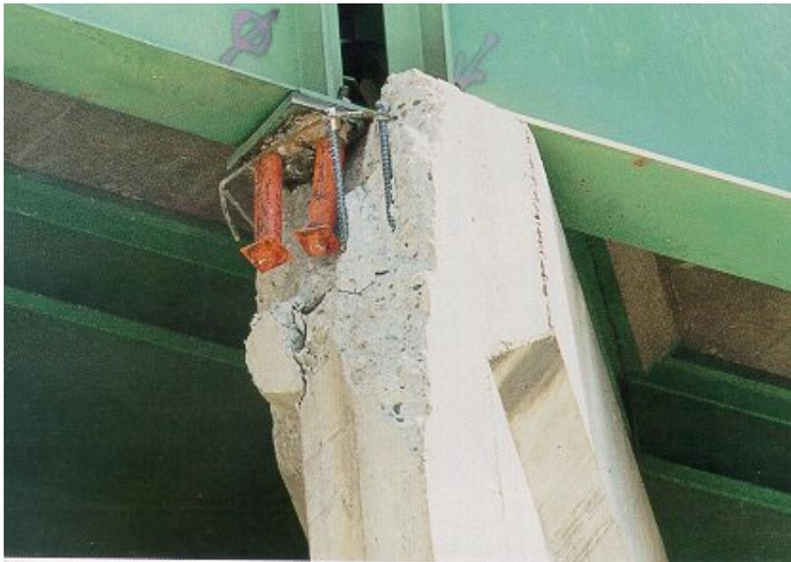
**Figure 20.2.2-5 Anchorage Assembly Failure – Santa Ana River Bridge, 1994 Northridge Earthquake (Astaneh-Af, A. et al., 1994)**
