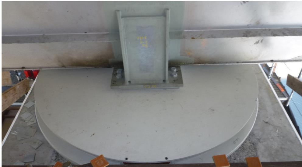
**Figure 20.2.8-32 Typical Isolator Bearing Installed**
