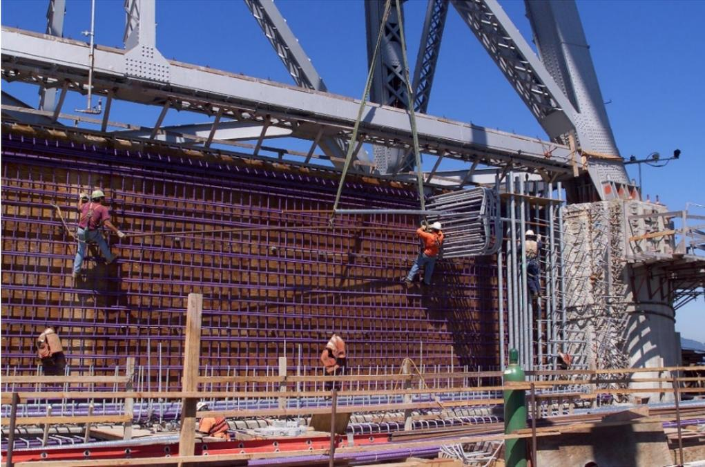
**Figure 20.2.8-57 Diaphragm Strengthening for Four-Bell Piers Under Construction**
