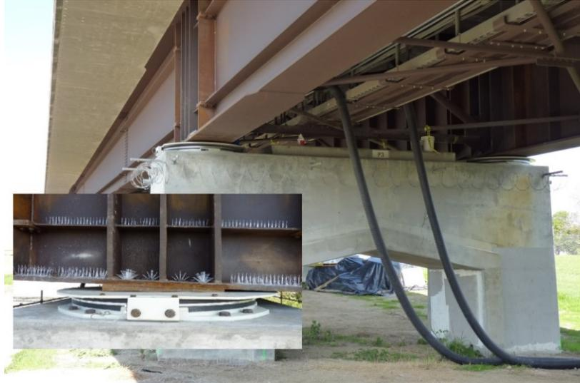
**Figure 20.2.8-25 Typical Seismic Isolation Bearings Installed**
