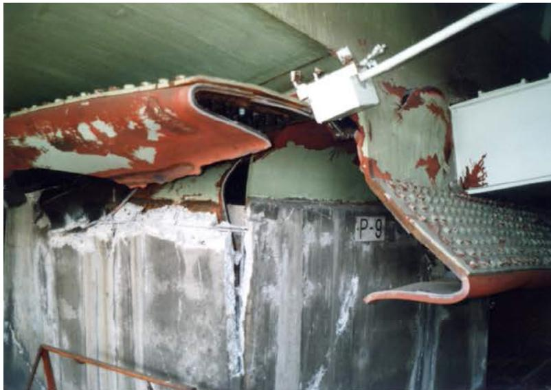
**Figure 20.2.2-3 Iwaya Viaduct Steel Pier Failure, 1995 Hyogo-Ken Nanbu Earthquake, Japan (Goto, 2014)**
