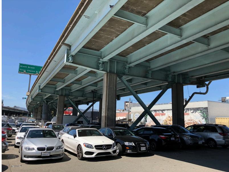
**Figure 20.2.8-10 San Francisco Bayshore Viaduct – Concrete Column Bents**
