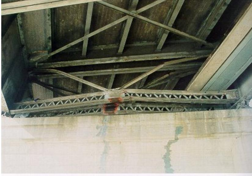
**Figure 20.2.2-6 End cross frame inelastic buckling
