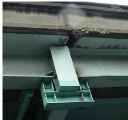
Figure 20.2.8-16 Bayshore Viaduct Superstructure Girder Seat Extension
