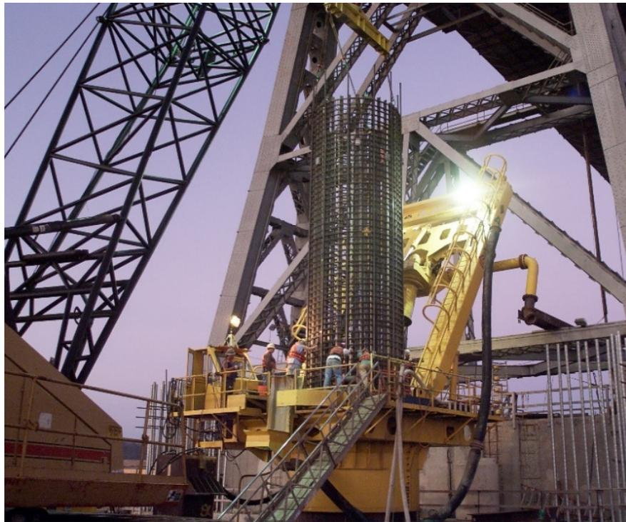
**Figure 20.2.8-58 Cast-in-Steel-Shell (CISS) Piles under Construction**
