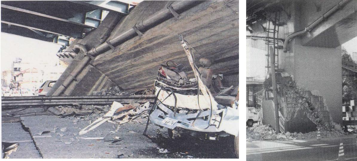
**Figure 20.2.2-2 Concrete Column Brittle Failure, 1995 Hyogo-Ken Nanbu Earthquake, Japan**
