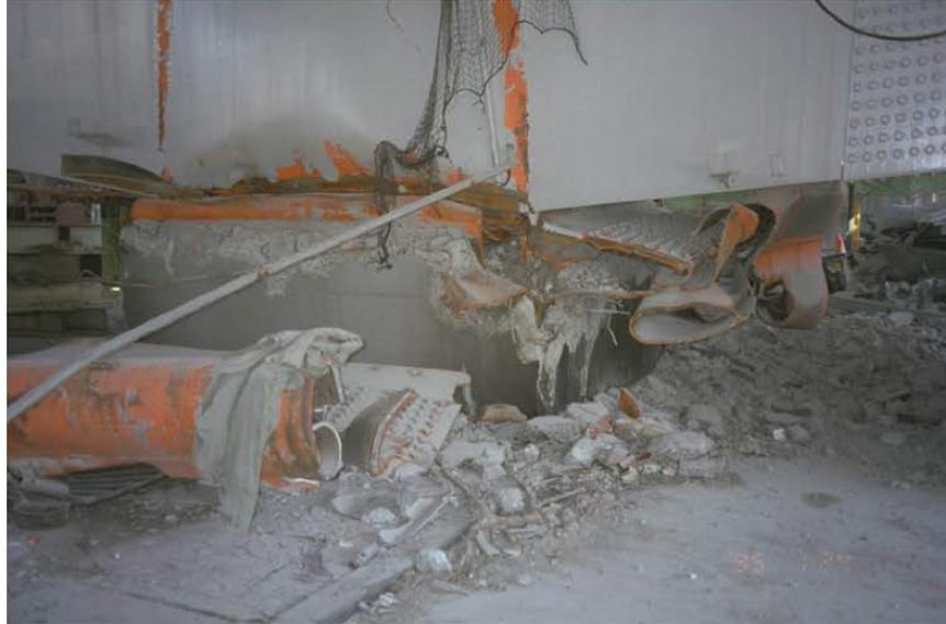
**Figure 20.2.2-4 Tateishi Viaduct Steel Pier Failure. 1995 Hyogo-Ken Nanbu Earthquake, Japan (Goto, 2014)**
