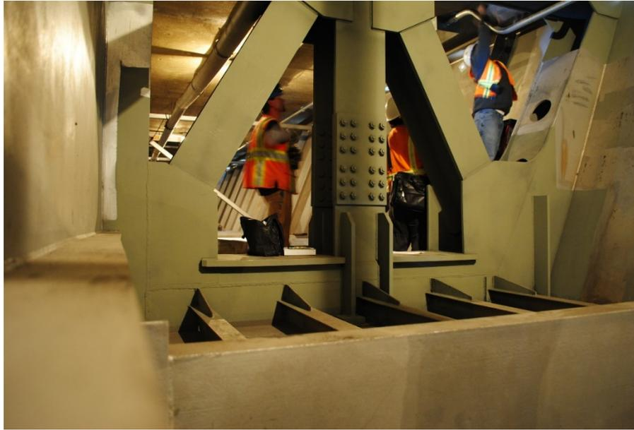
**Figure 20.2.8-33 Typical Strengthened Cross Frame at Piers**
