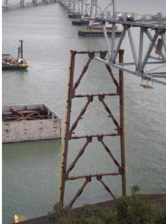
**Figure 20.2.4-5 Eccentrically Braced Frames – Temporary Tower for San Francisco Oakland Bay Bridge East Span Construction**
