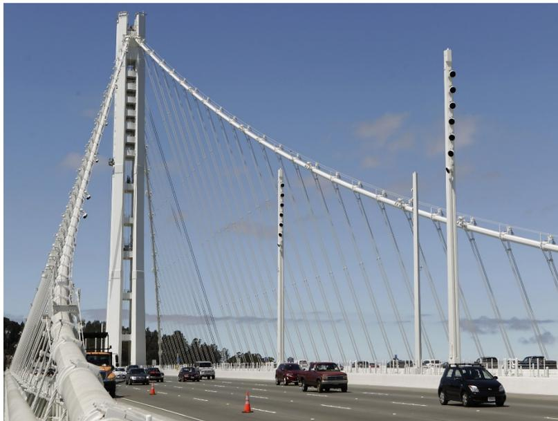
**Figure 20.2.4-4 Eccentrically Braced Frames - Self-Anchor Suspension Bridge Tower – San Francisco Oakland Bay Bridge East Span**
