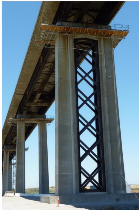
**Figure 20.2.8-26 Pier Cross Frame Bracings under Construction**
