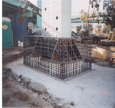
**Figure 20.2.8-19 Steel Column, Grillage, and Footing Retrofit**
