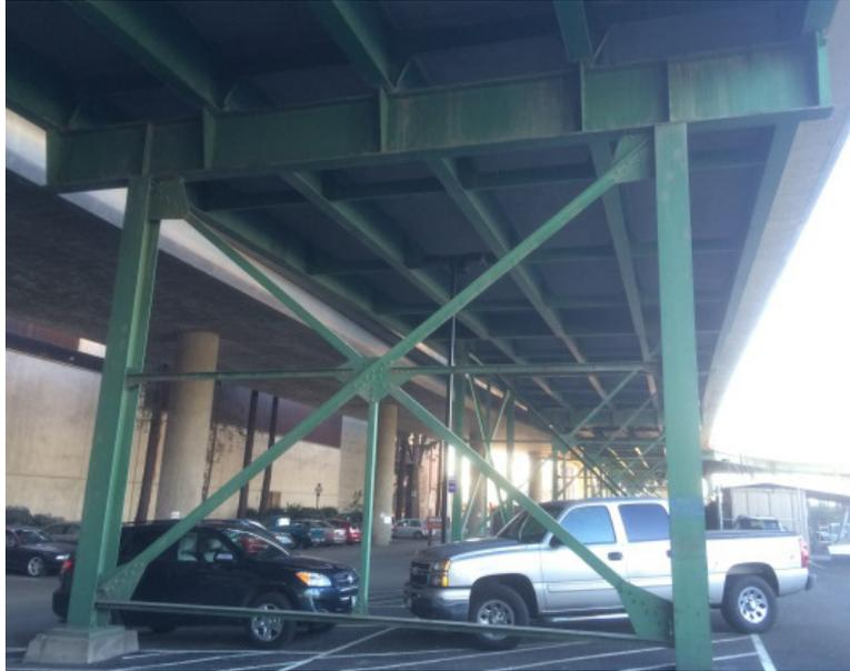
**Figure 20.2.4-3 Concentrically Braced Frame –I-5 Ramp in Sacramento Valley Station**
