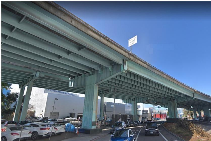
**Figure 20.2.8-9 San Francisco Bayshore Viaduct – Steel Column Bents**
