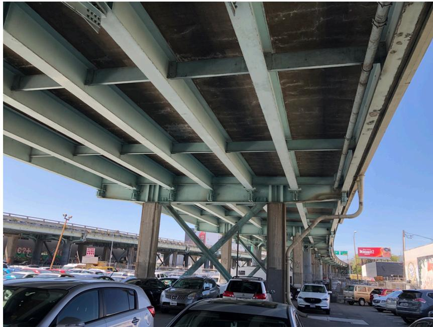
**Figure 20.2.8-18 Concrete Bent Retrofit - Diagonal Cross Bracings**
