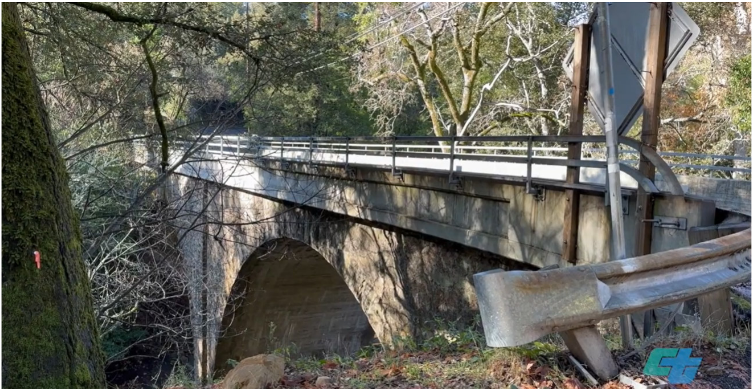
Saratoga Creek Bridge Rehabilitation Project
