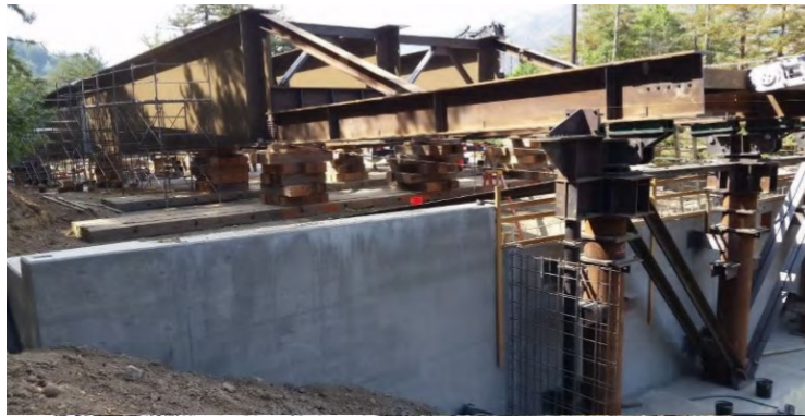
(a) Launch setup at abutment
