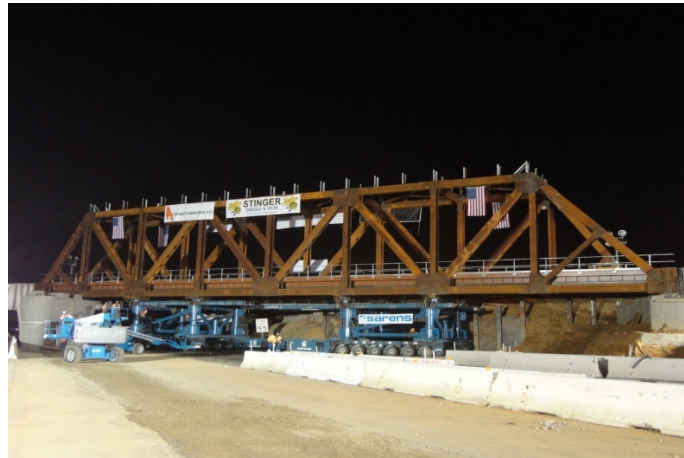
(b) SPMT move of a truss span
