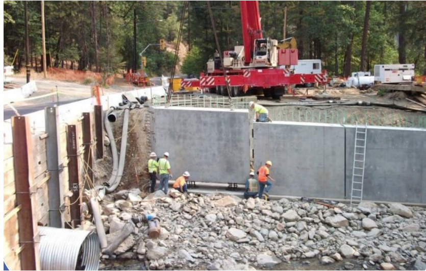
Figure 4.9.4.4.4-1 Precast Abutment Wall Element Placement – Fort Goff Creek Bridge
