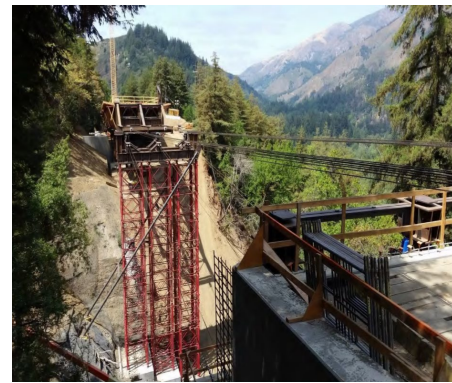
(b) Temporary launch tower
