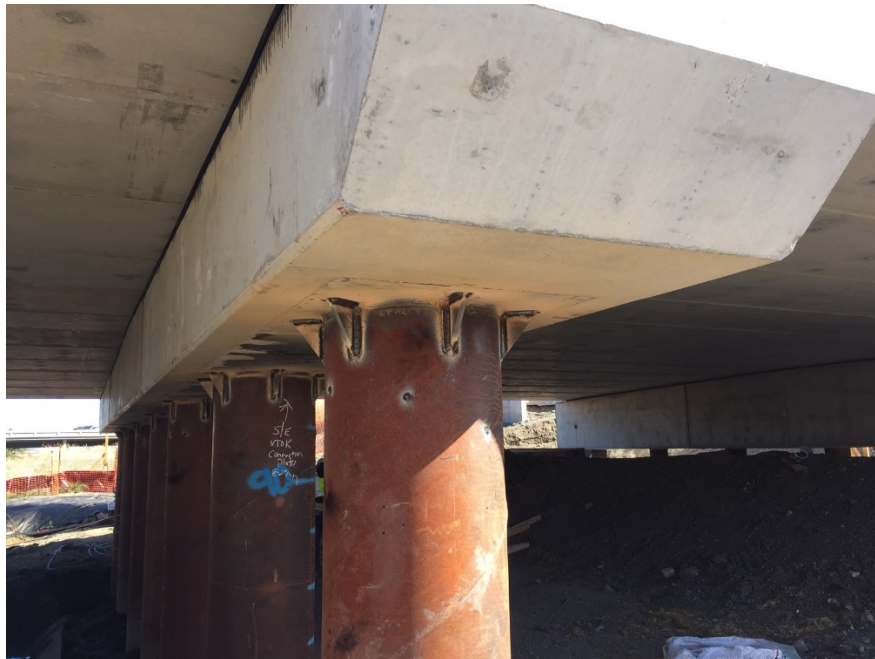
Figure 4.13.1.3-1 CISS Piles supporting a precast concrete bent cap and voided slabs, Old Mountain View Bridge in the City of Sunnyvale (Courtesy of KIE-CON, Inc.)
