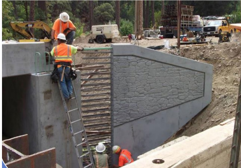
Figure 4.9.4.4.5-1 Precast Cantilever Wing Wall – Fort Goff Creek Bridge
