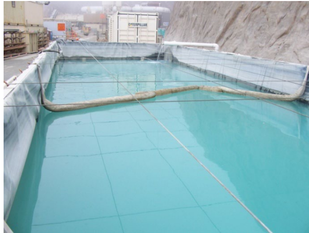
Figure C-3. Sedimentation Tank (Devil's Slide)
