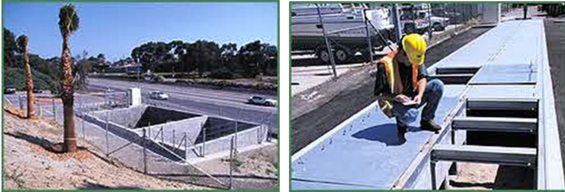
Figure B-16. Caltrans Pilot Media Filters (Austin Sand Filter [left], Delaware Sand Filter [right])
