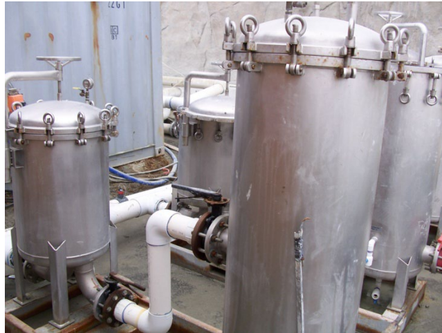
Figure C-4. Bag/Cartridge Filters (Devil's Slide)
