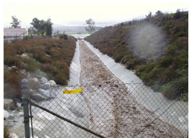
Figure 865.2 Concrete Lined Channel
