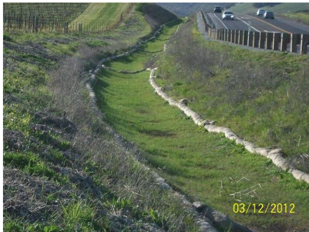
Figure 865.1 Steep-Sloped Channel with Composite Vegetative Lining
