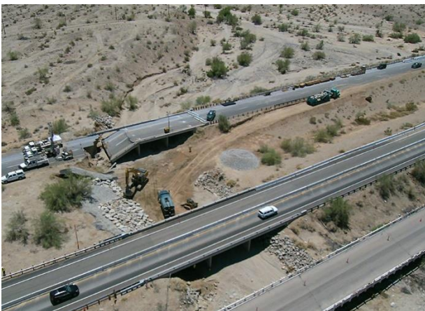
Bridge Abutment Failure at Tex Wash on I-10 after a Flood Larger Than the Design Flood
