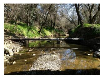
Figure B4.8. Typical Bed Material Size, Arcade Creek site 13. Note exposed pipeline, which is diagnostic of channel incision.
