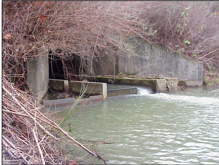
Figure 7-8. Enhancements at box culvert outlets might include training walls and notched weir sills to maintain flow depth in the main channel section, along with secondary entrances to promote better conditions for juveniles during higher flow conditions. (Photo courtesy of ODOT)
