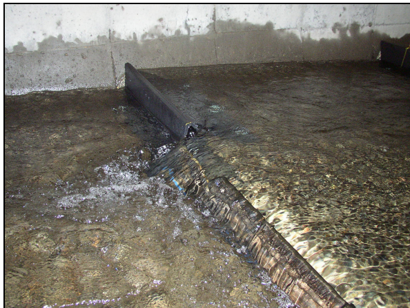
Baffle weirs spanning a steep-slope box culvert. (Photos courtesy of ODOT)
