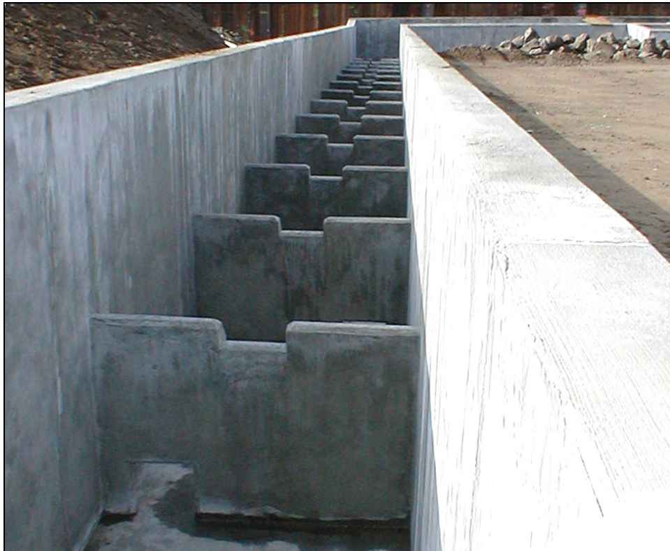
Figure 9.1. Pool and weir ladder.
