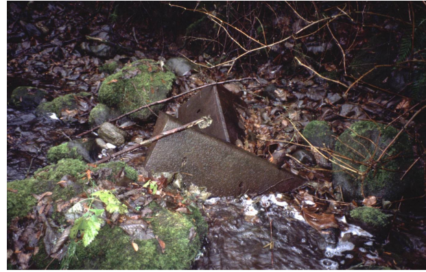
b) failure due to insufficient anchoring
