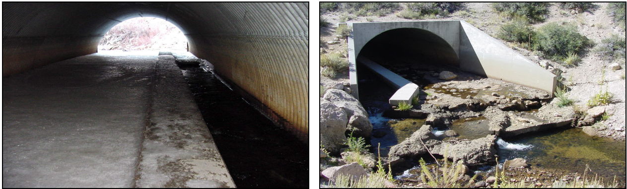
Figure 7-2. Longitudinal channel weir and grade control rock weirs at the Crooked Creek retrofit project.
