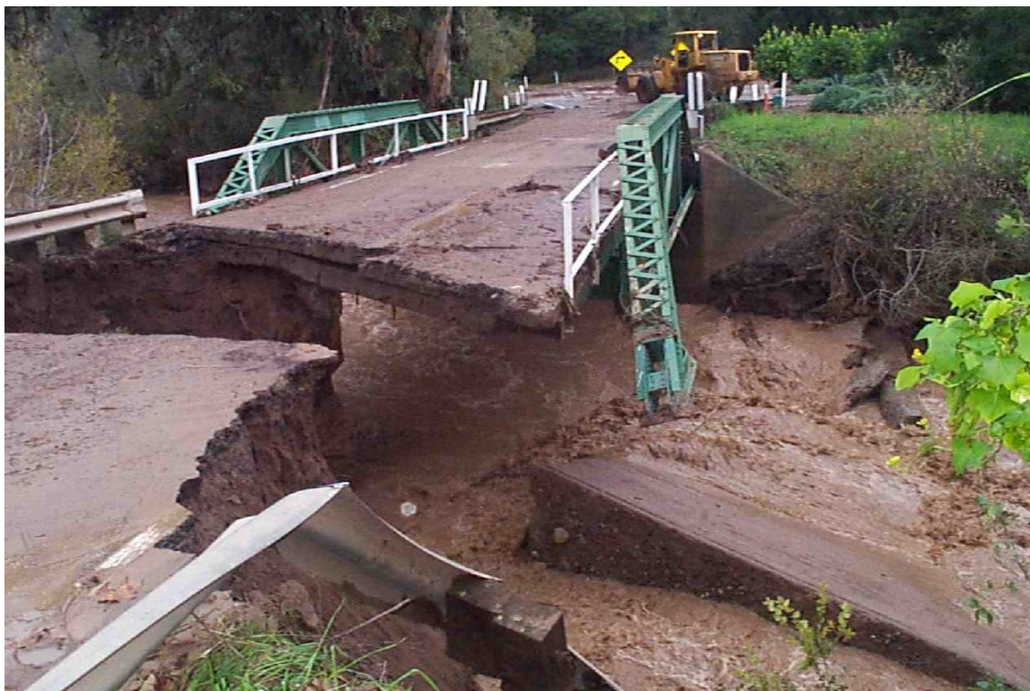
Figure 2- Highway 150 Bridge Failure, Central Coast, Winter 2005
