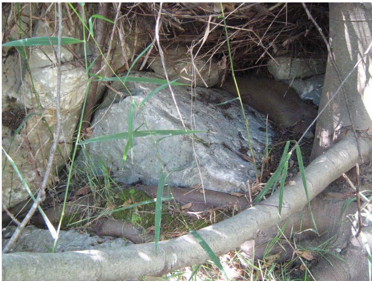
Figure 7- Weaver Creek, Root System through Soil and RSP
