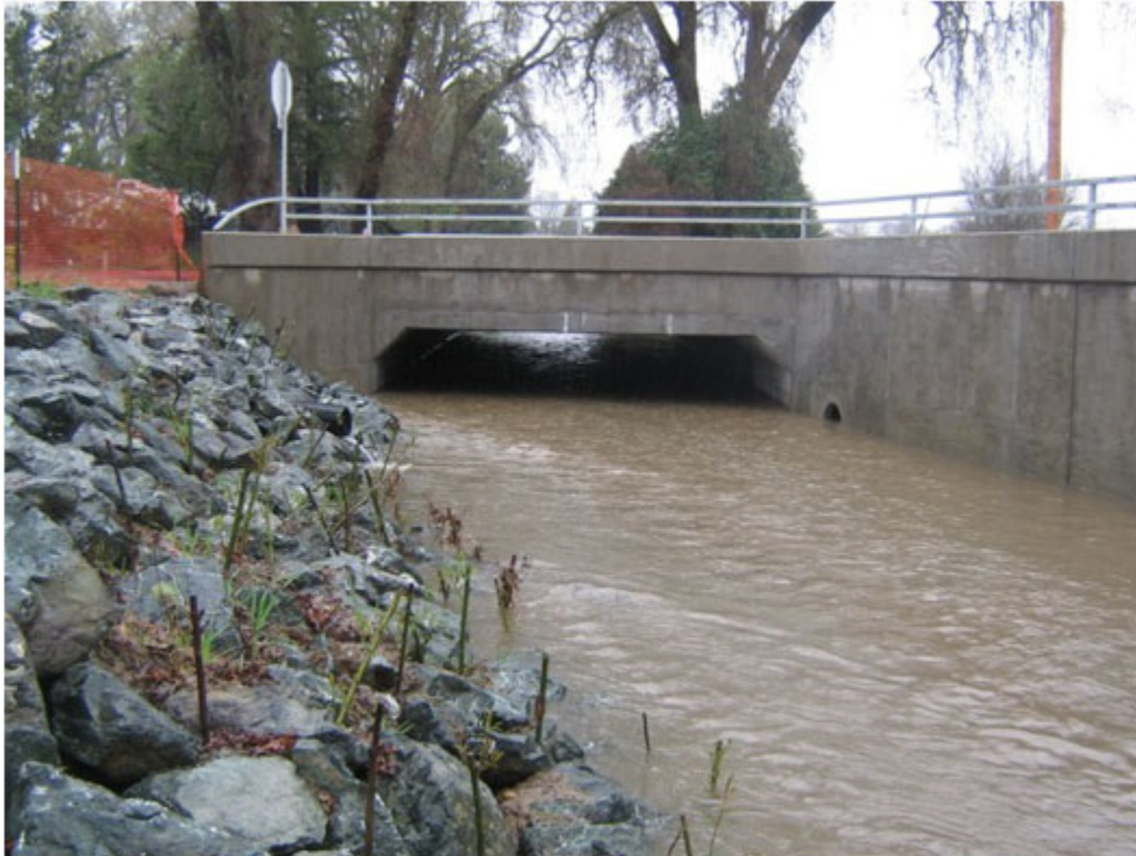
Figure 17- Gibson Creek, Cuttings through RSP (Right After Installation, Fall 2010)
