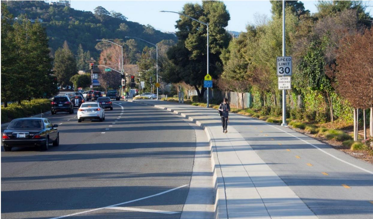
**Figure 5-L - Delineators provide vertical separation on a suburban segment of SR-126 in Fillmore**
