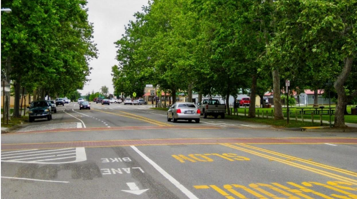
**Figure 5-F – Buffered Class II bike lane on SR-135 in Los Alamos.**
