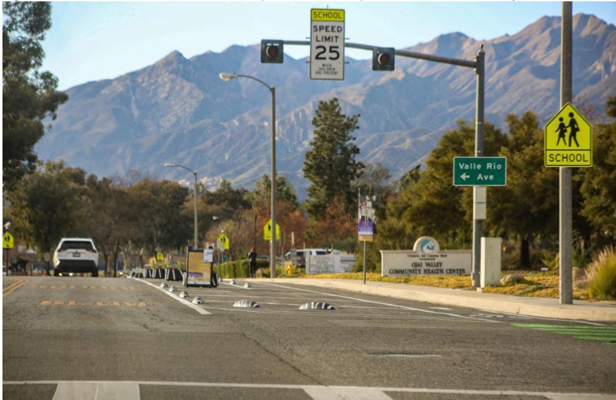
**Figure 5-N – Parking-separated Class IV separated bikeway on SR-41 in Atascadero**
