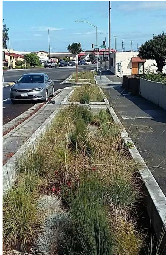
**Figure 8-L – Bioretention features separate modes on SR-123 in El Cerrito**
