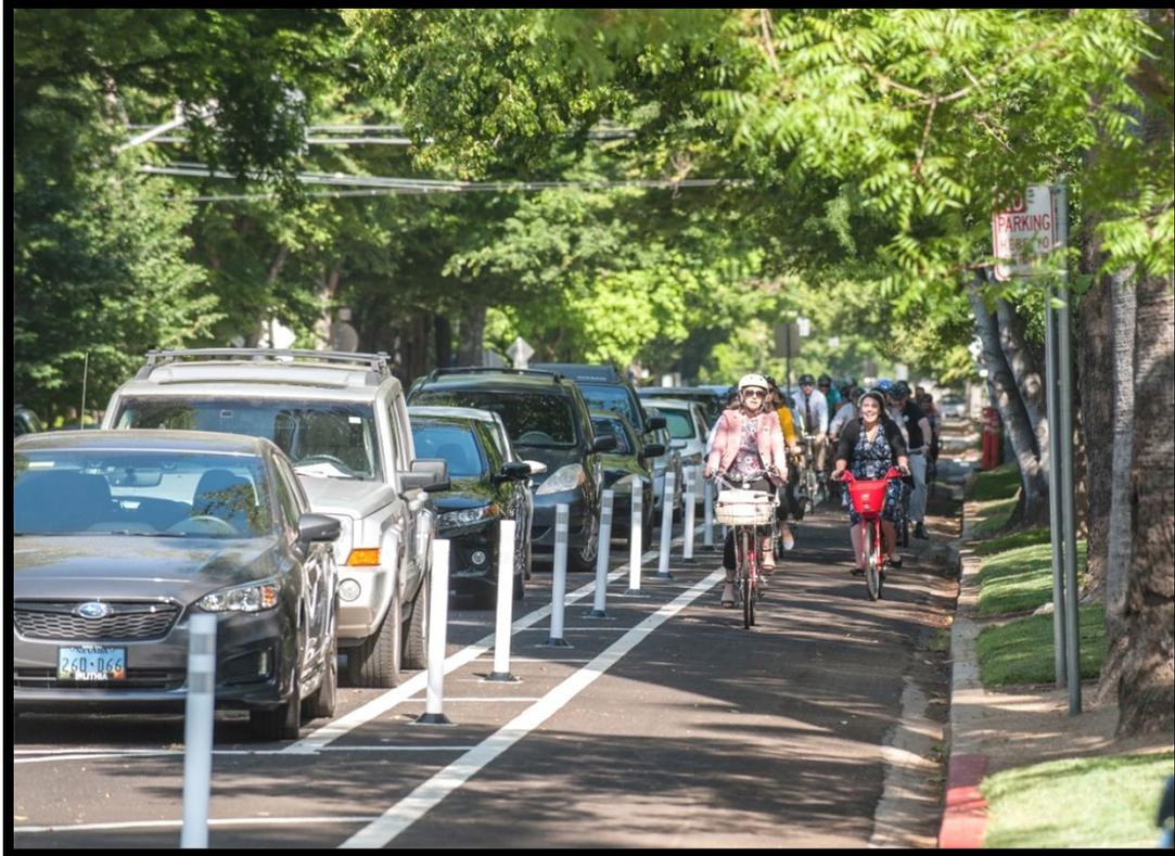
**Photo 3: Separated Bikeway with parking and flexible posts in Sacramento**
