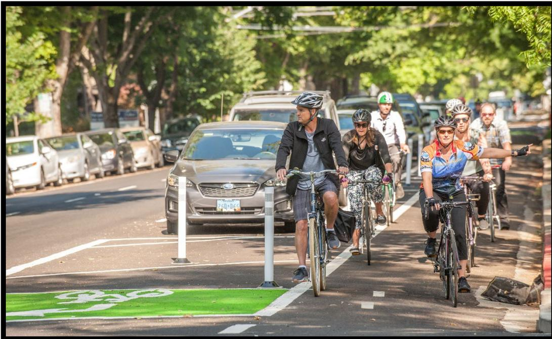
**Photo 7: Separated Bikeway with a Bike Box**
