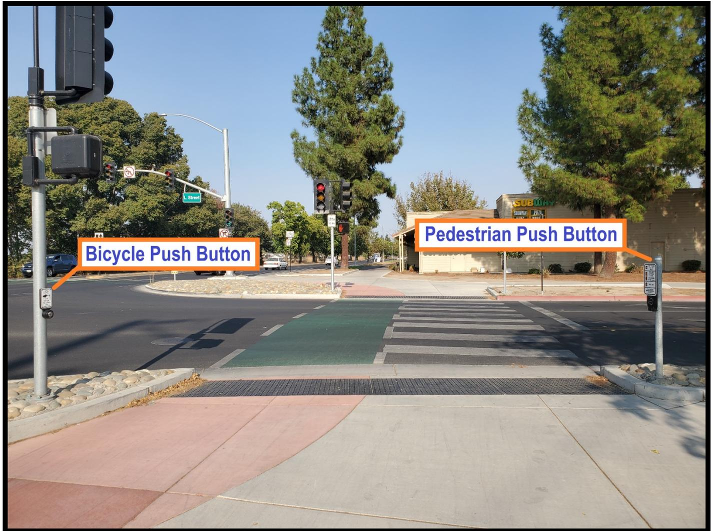
**Photo 8: Separate push button placement for bicyclists and pedestrians**
