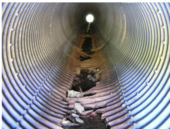
Shape Distortion Caused by Backfill Soil Loss
