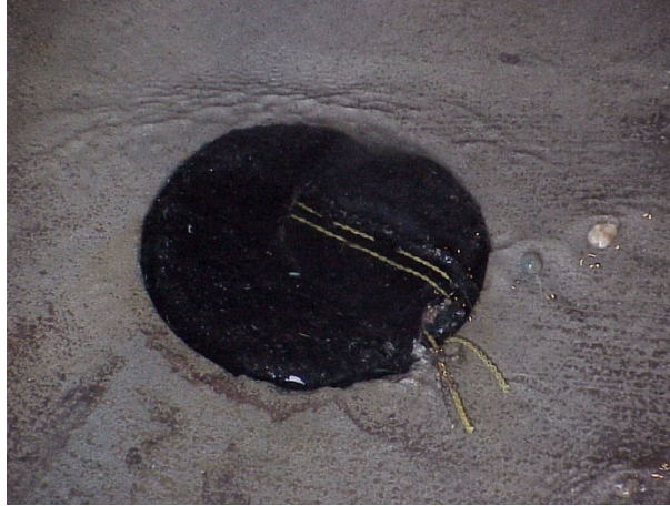
Installed Gravel Filter Bag in Invert Weep
