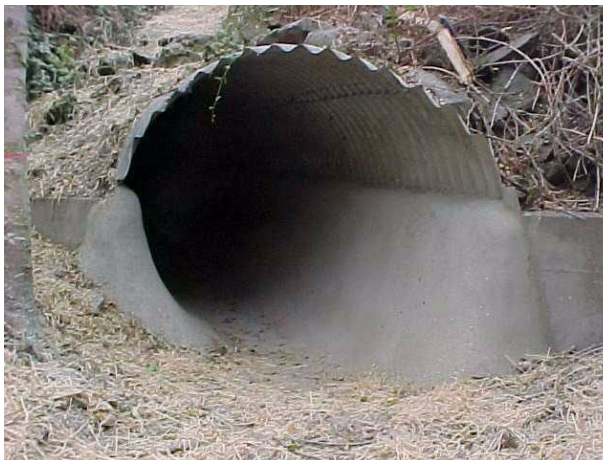
Inlet of 96-Inch Pipe After Repair
