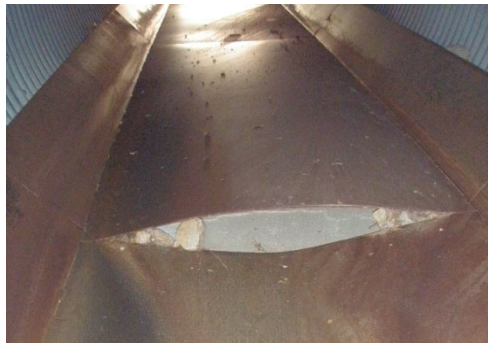
Insufficient Anchorage with No End Treatment
