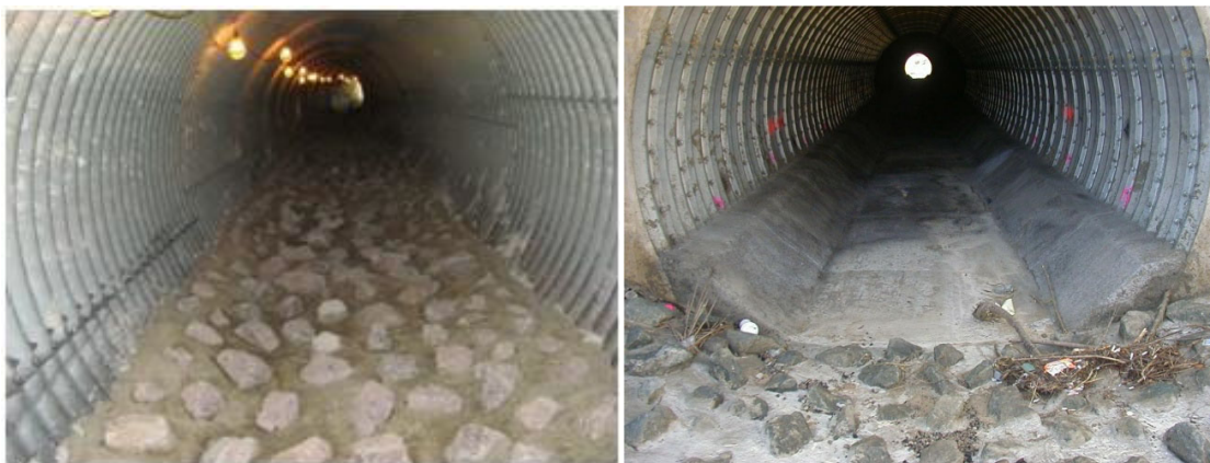
Concreted Rock Slope Protection (CRSP) Calcium Aluminate Abrasion Resistant Concrete
