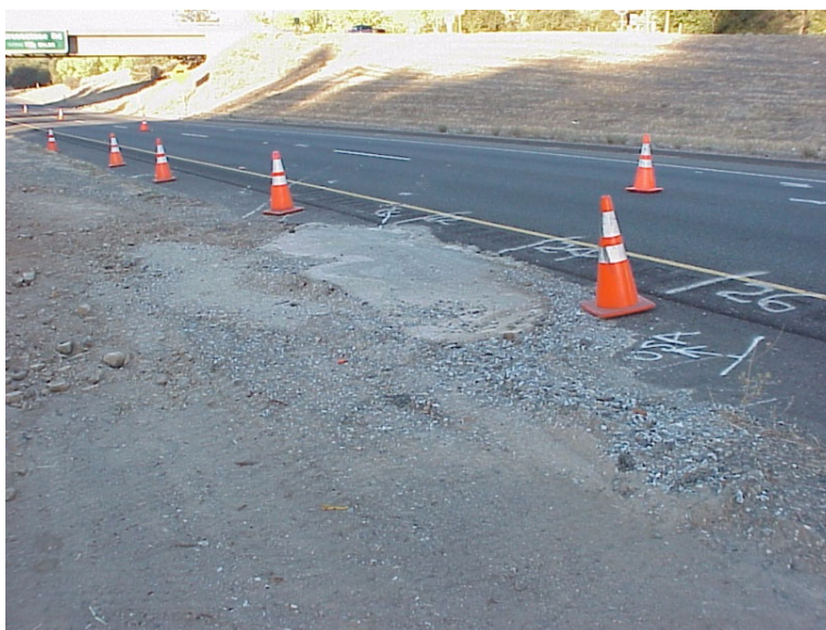
Freshly Placed Slurry where Void Migrated to Surface
