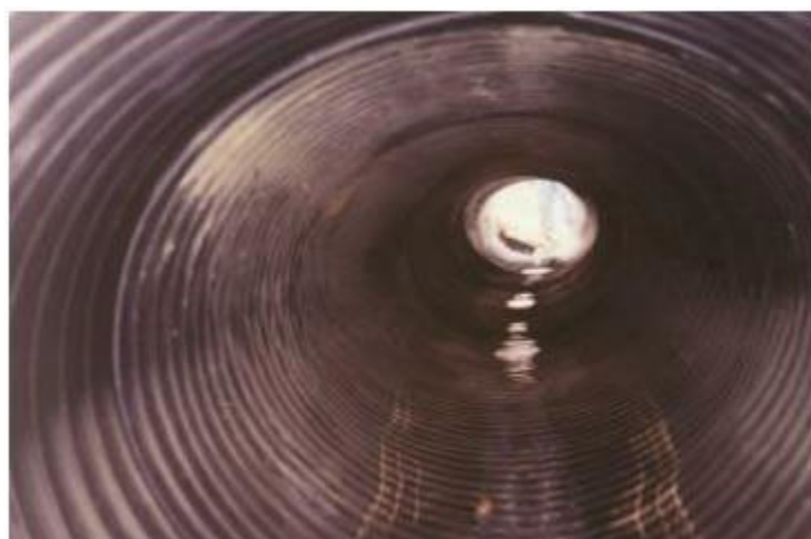
Splitting of 60 inch Diameter Pipe. This Pipe was Installed in 1996 by Another State
