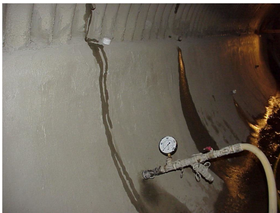
Contact Grouting Through Grout Port
