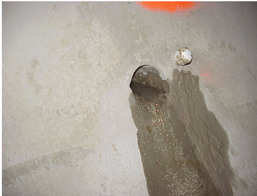
“Cored” Grout Hole in Shotcrete Used to Fill Large Void with 3-Sack Sand Slurry Leaking Groundwater During Contact Grouting. Note capped contact grout port.
