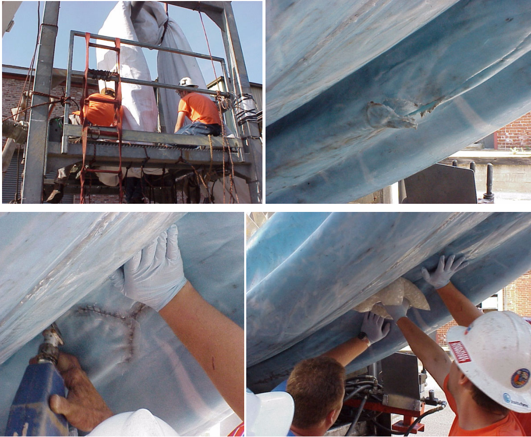
Example of Liner Tear During Installation and Subsequent Repairs
