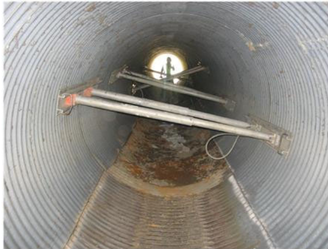
Sawcut CMP Invert Triggering Failure During Invert Repair
