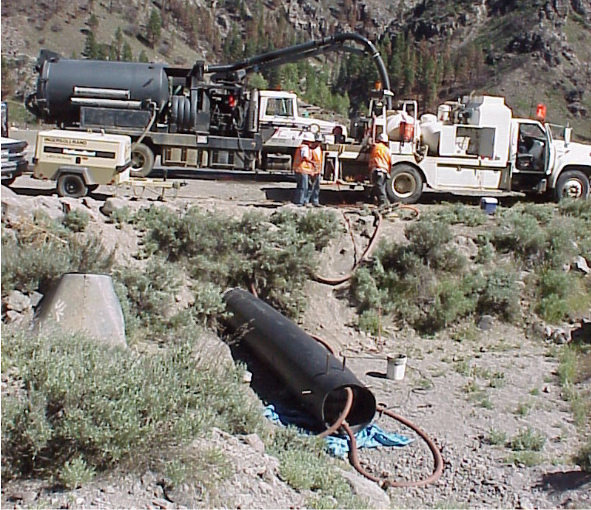
Steam Being Introduced into 30 Inch HDPE Liner
