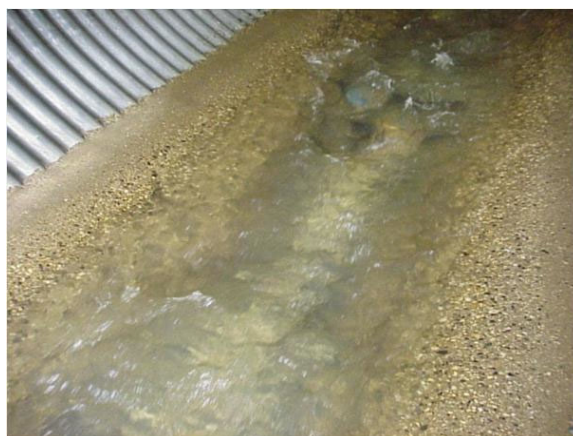
(Above) Example of Insufficient Concrete Invert Paving Design Thickness for Abrasion Level 6
