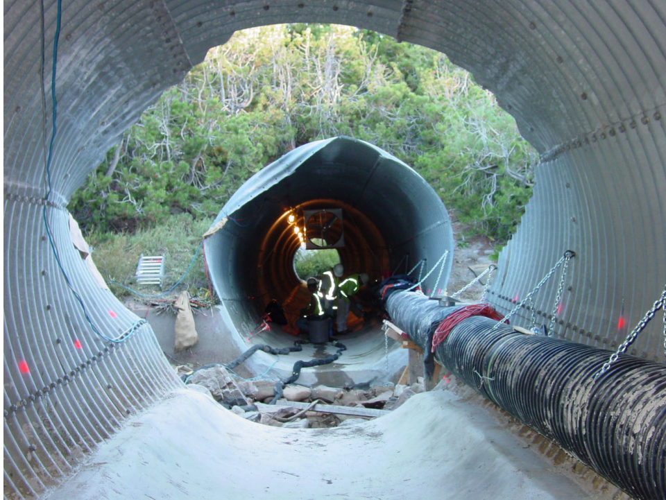
View of Both Pipes After Concrete Invert Paving
