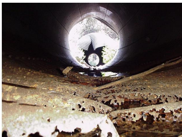
Corroded and Overlapping Invert. Note oval shape of pipe
