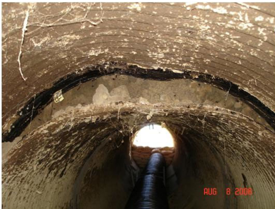
Separated Joint CMP with Physical Separation of Pipe Ends
