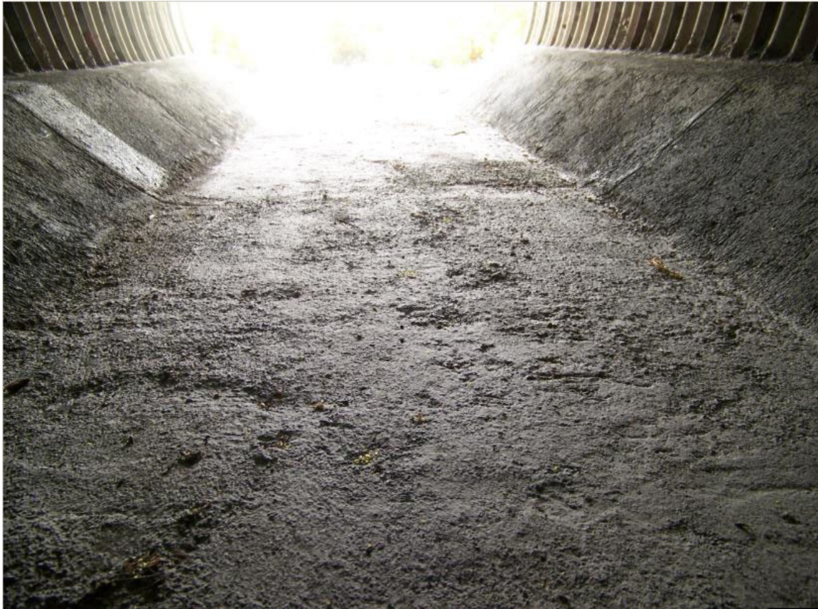
Concrete Invert Repairs with Trapezoidal Section
