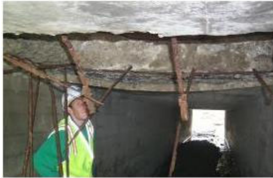
Failed Crown in Reinforced Concrete Box Culvert
