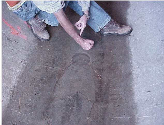
Cored Weep in Shotcrete Invert
