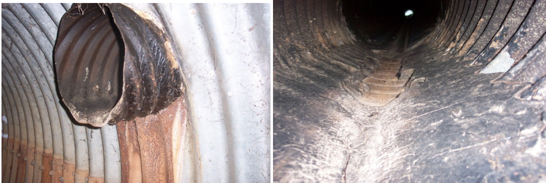
36 Inch Bitumen Coated CMP Tie-In. Note rust stain below from perforated invert. Perforations in invert to 36 inch CMP allowed water to leak behind 96 inch culvert
