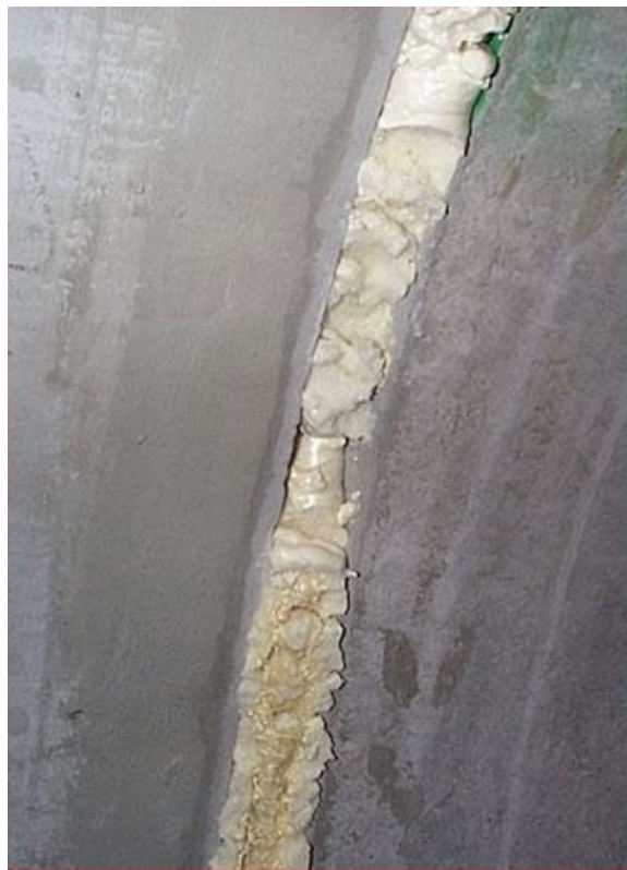
Internal Chemical Grouted Joint (RCP)
