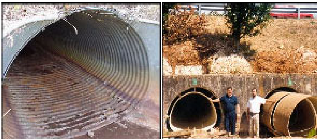
Existing Multi-Plate Arch Before Lining
