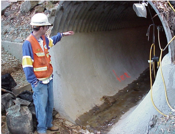
Outlet of 96-inch Pipe After Repair
