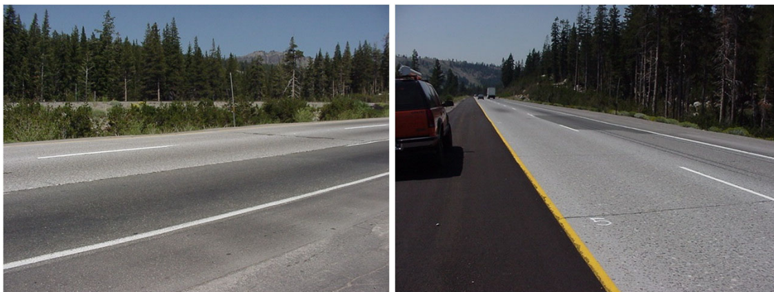
Dip in Number 1 EB Lane. Summer 2002 Dip in entire WB freeway Section. Summer 2002
