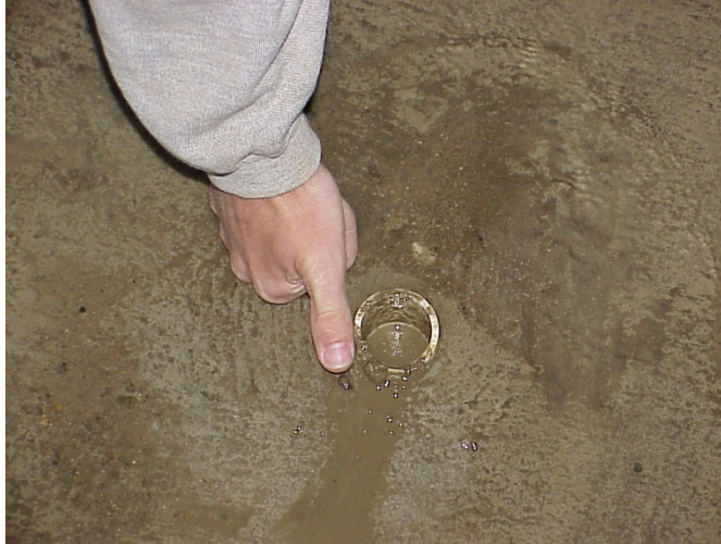
PVC Pipe “Weep” Placed in Rock Below Invert. Later, larger weeps were “cored” in addition in addition to these.
