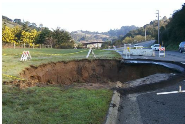
Sink Hole Damage (Location Unknown)
