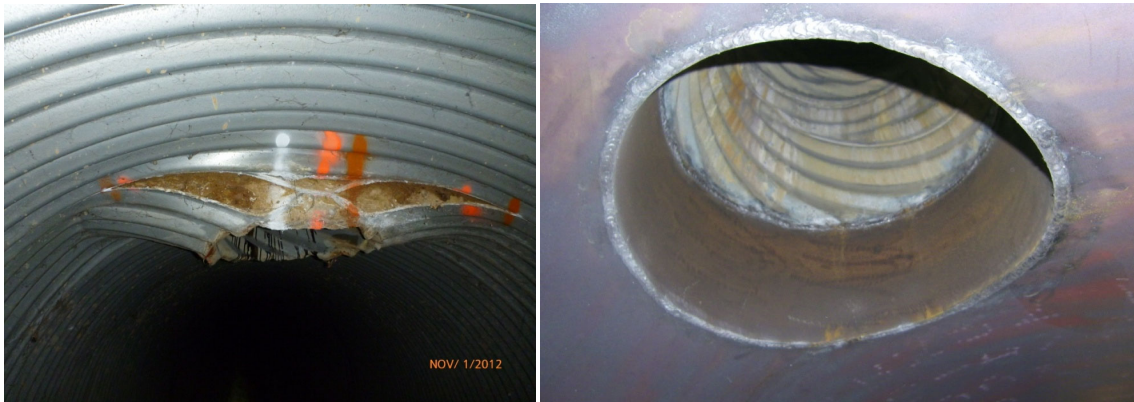
Localized Repair to 84-inch CMP in Vicinity of 18-inch Riser 12-ORA-261-PM 3.74
