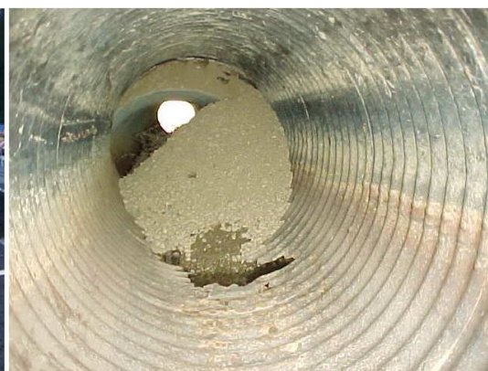
Loss of Backfill Fines
