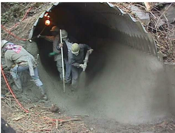
Placing Shotcrete
