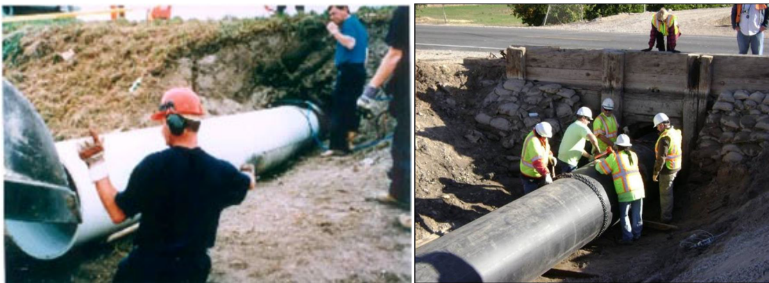
Inserting PVC and HDPE Slipliners
