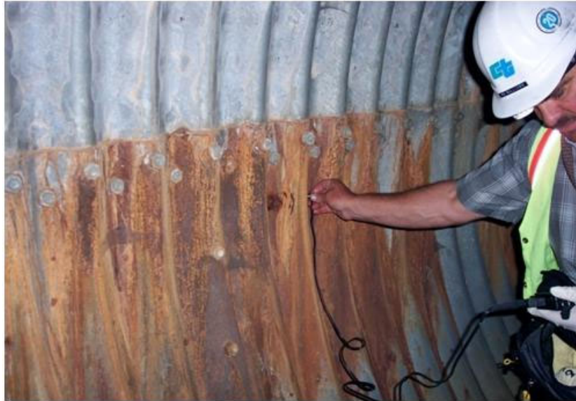
Taking Thickness Measurements. Note Evidence of Leaking Horizontal Seam at Springline
