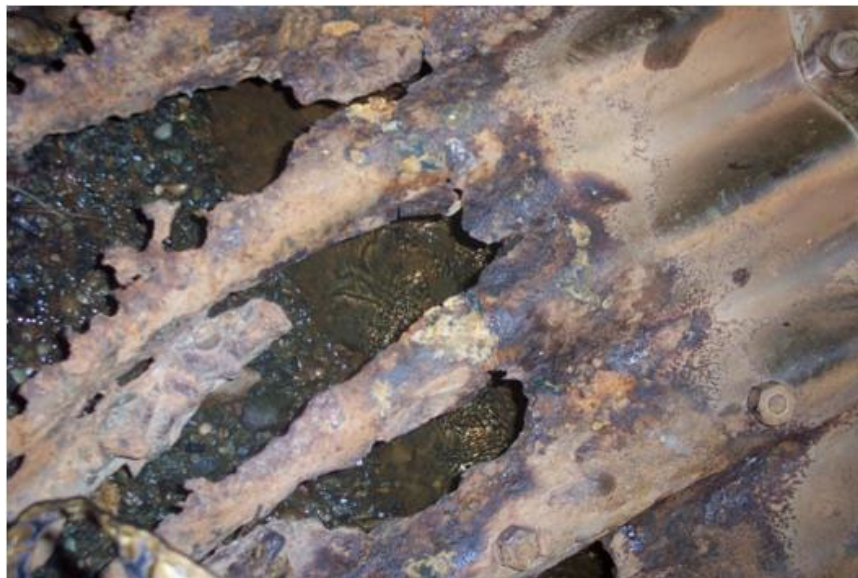
Total Loss of Invert and Existing Nuts Showing Minimal Wear
