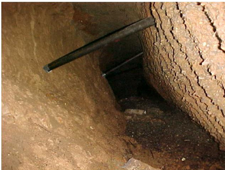
Large, Long Void That Was Located By Probing. Note corroded back side of culvert on right side of picture.
