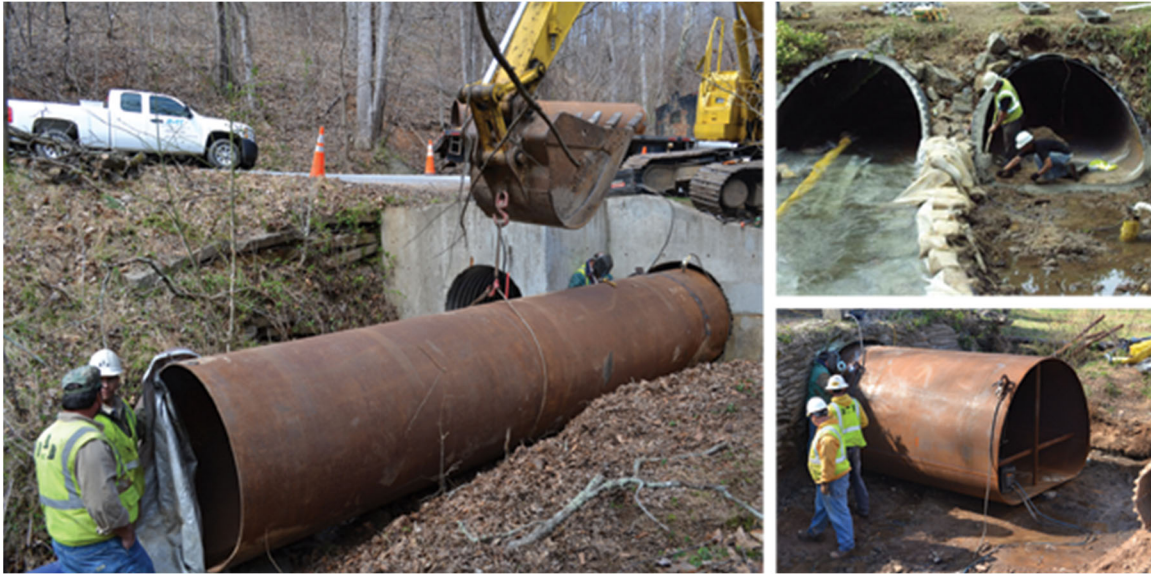
Various Welded Steel Pipeliner Structural Repair Installations (InfraSteel®. Courtesy of Precision Pipe & Products, Inc.)
