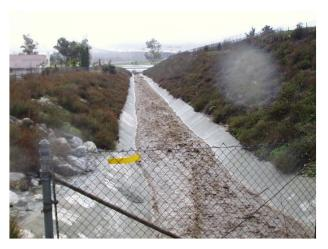
For large flows, consideration should be given to using a minimum bottom width of 12 feet for construction and maintenance purposes, but depths of flow less than one foot are not recommended. Despite the non-erodible nature of rigid linings, they are susceptible to failure from foundation instability and abrasion. The major cause of failure is undermining that can occur in a number of ways.
