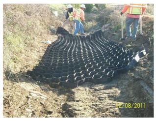
Placing a polyethylene cellular soil confinement system on a steep-sloped channel.
