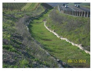
Vegetative flexible lining placed on top of cellular soil confinement system on a steep-sloped channel.
