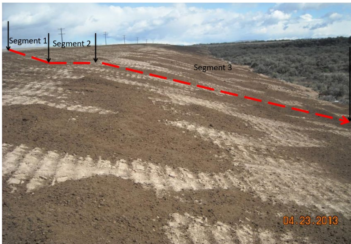
Figure 2-4. Complex slope with multiple segments
