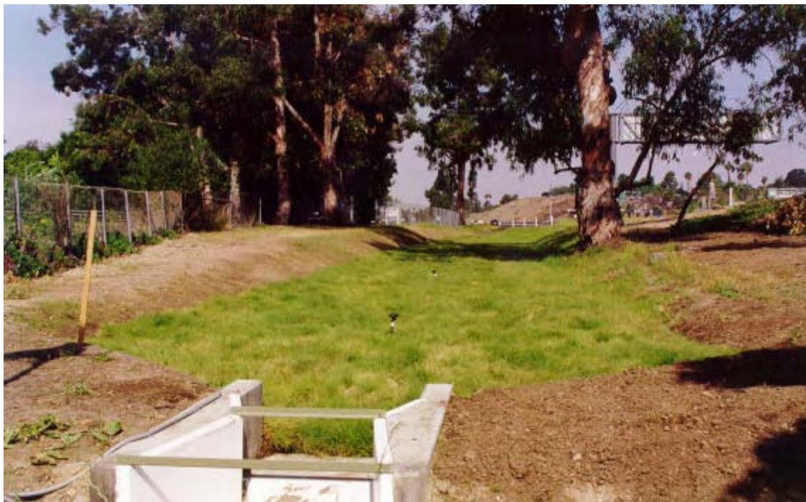
Figure 1-2. Biofiltration Swale (SR-78/Melrose Drive)
