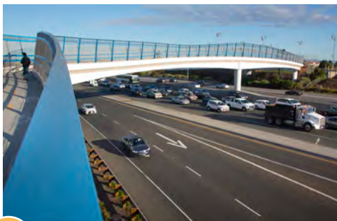
2 Pedestrian/Bicycle Bridge in Belmont
