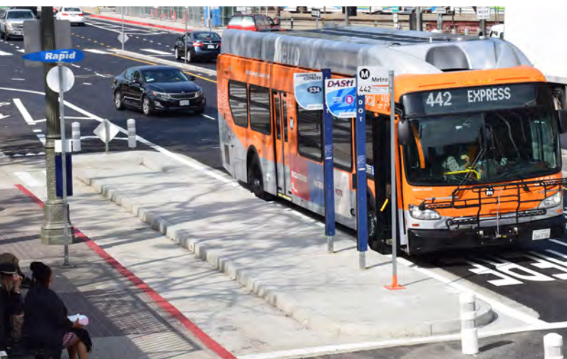
A side boarding island transit stop in Los Angeles is separated from the sidewalk by a bike channel, eliminating conflicts between transit vehicles and bikes at stops. Photo credit: LADOT Bike Blog.
