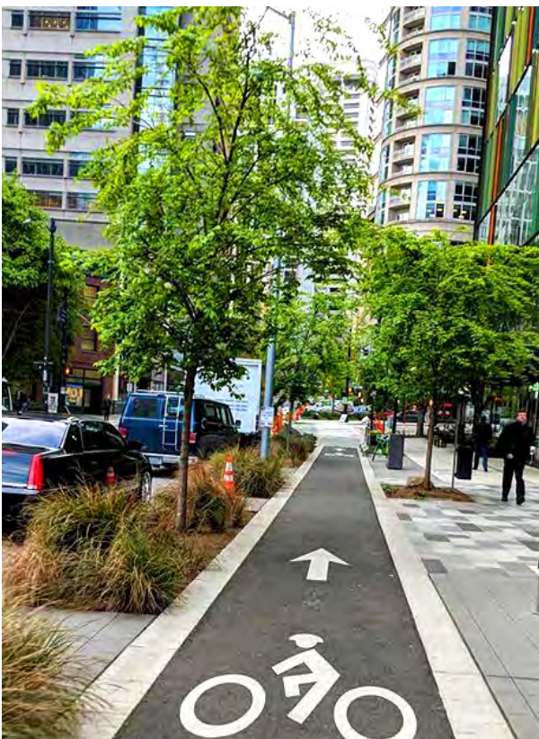
A Class IV Separated Bikeway using planted areas to separate bicyclists from motorized traffic and sidewalk in Seattle. Photo: Seattle DOT, Flickr CCL.
