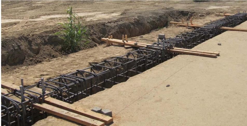
Figure 2-2 Rebar for Barrier
