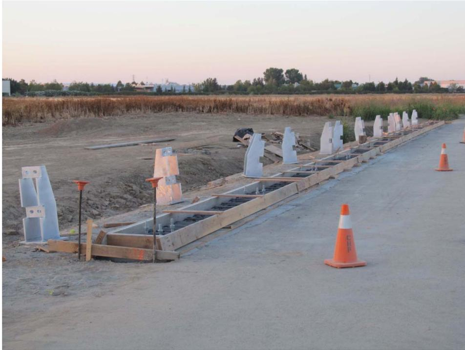
Figure 2-4 Before the Second Concrete Placement For Curb
