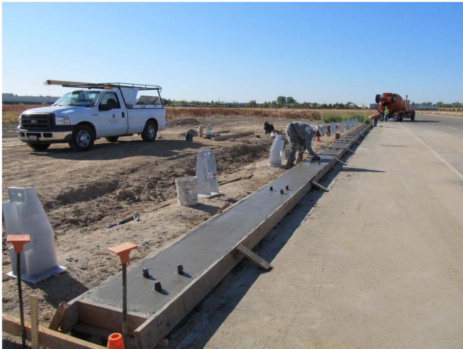
Figure 2-5 After the Second Concrete Placement
