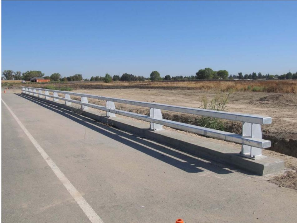
Figure 2-6 Completed Barrier Construction Front
