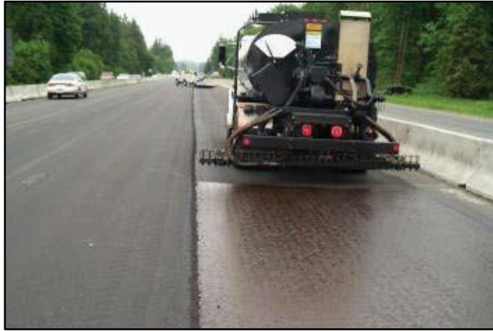
Figure 8-1. A spreader applies tack coat.
