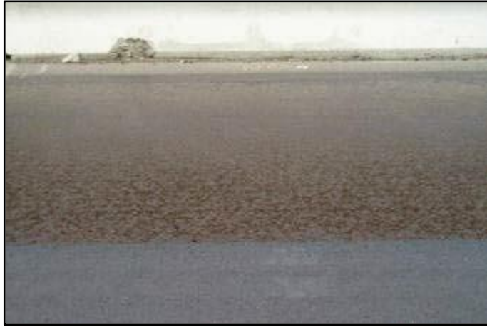
Figure 8-7. The brown color indicates that the freshly placed emulsion tack coat has not yet broken.
