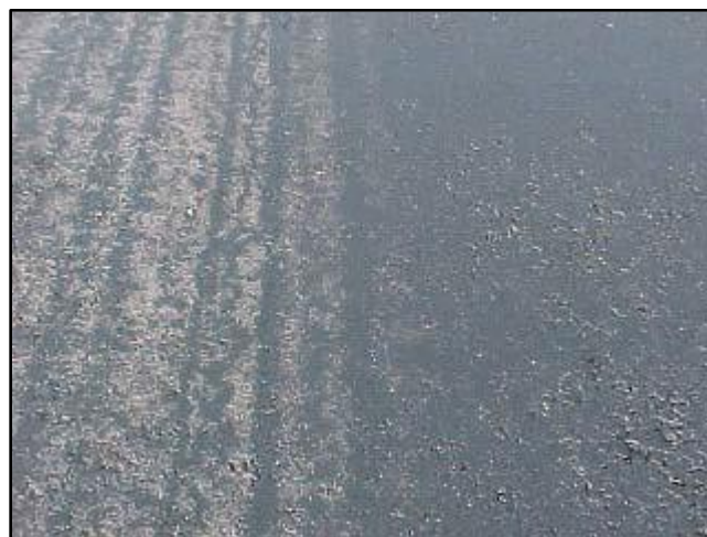
Figure 8-6. Poor, left, versus good, right, tack coat coverage. Note streaky coverage of poor coat and nearly complete coverage of good coat.
