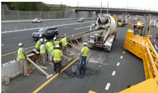
Concrete Barrier Construction Using Mobile Barrier System for Positive Protection Photo Source: Mobile Barriers LLC
