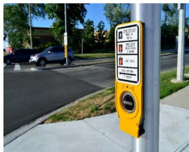
□ Where two PPB are provided on the same corner of a signalized locations, the push buttons should be separated by at least 10 feet.\* {CA-MUTCD – Section 4E.08 07}
