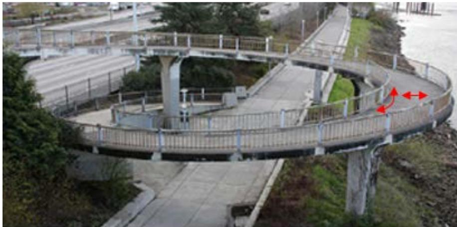
□ Ramps with greater than 5.0 percent running slope and a minimum of 30-inch rise must have landings at the top and bottom of each ramp run (see schematic below).\* {DIB 82-06 4.3.7(1)}
