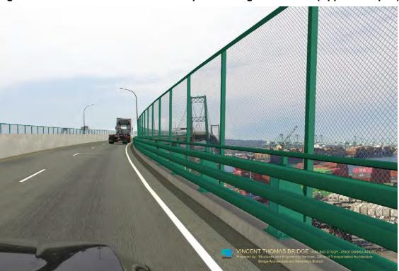
Figure 2.11-10: Photo Simulation or Proposed Bridge Rail/Fence (Approach Span)
