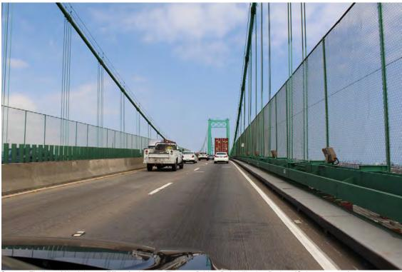
Figure 2.11-7: Existing Bridge Rail (Suspended Span)
