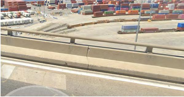
Figure 2.11-5: Existing Type 2 Rail on Approach Spans
