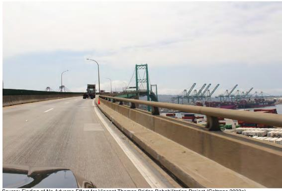
Figure 2.11-9: Existing Bridge Rail (Approach Span)
