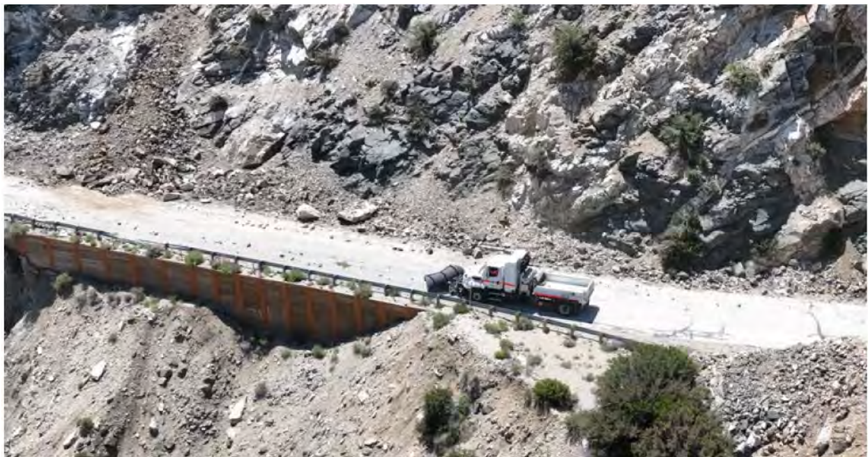
Example from SR-39. Retaining walls should be colored to match existing rock or nearby structure aesthetic treatments.
