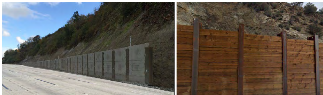
Catchment Wall examples: colored concrete and steel posts (left), and timber lagging and steel posts (right).
