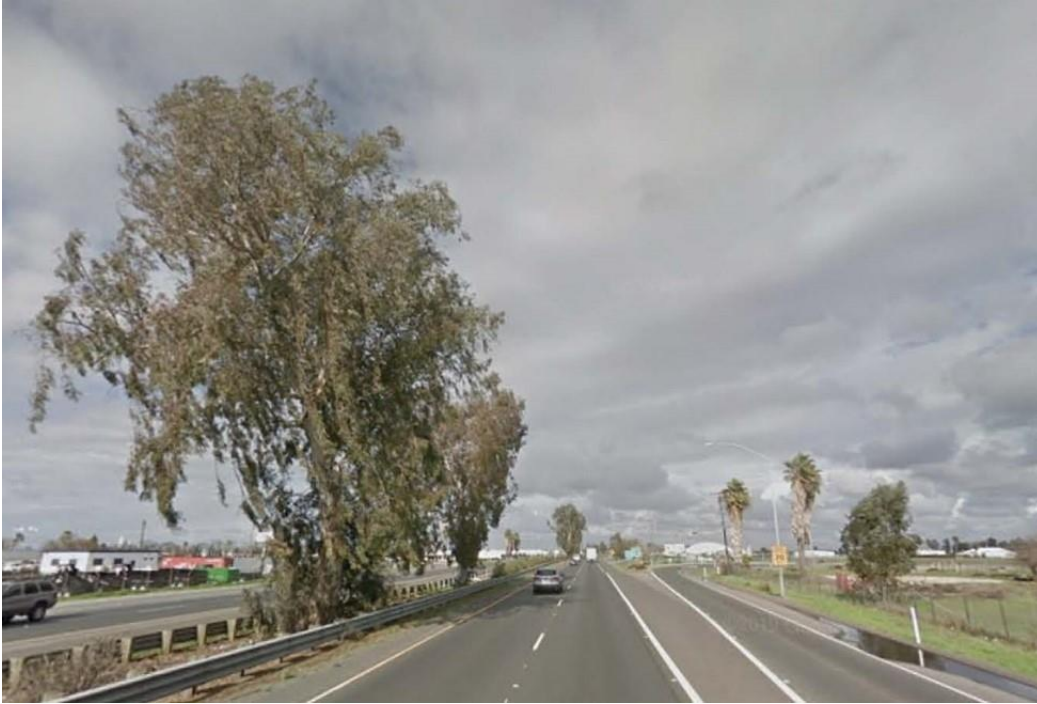
Figure 2-3: Existing Conditions of State Route 99 at Post Mile 25.4, North of the Avenue 200 Overcrossing
