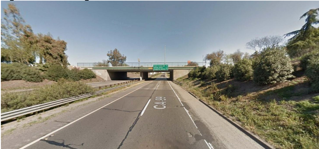
Figure 2-7: Existing Conditions at Post Mile 28.5
