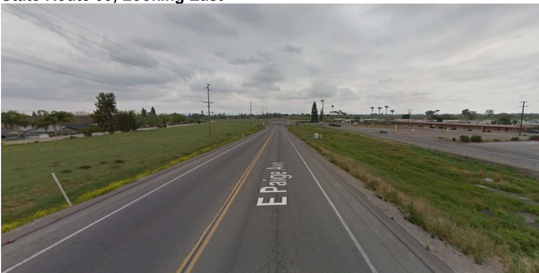
Figure 2-6: Existing Conditions on Paige Avenue on the East Side of State Route 99, Looking East
