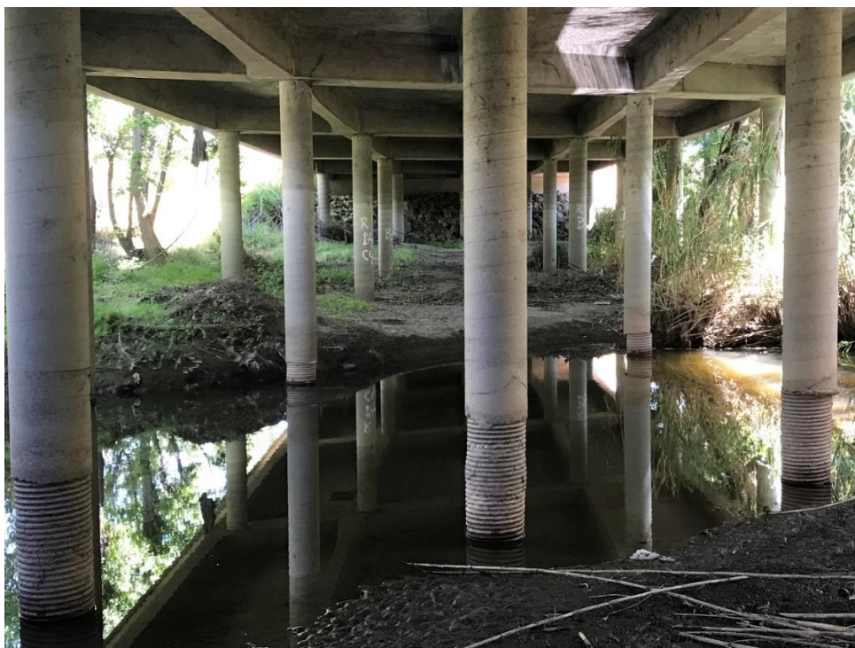
Figure 1-3 Mainline Exposed Bridge Piles
