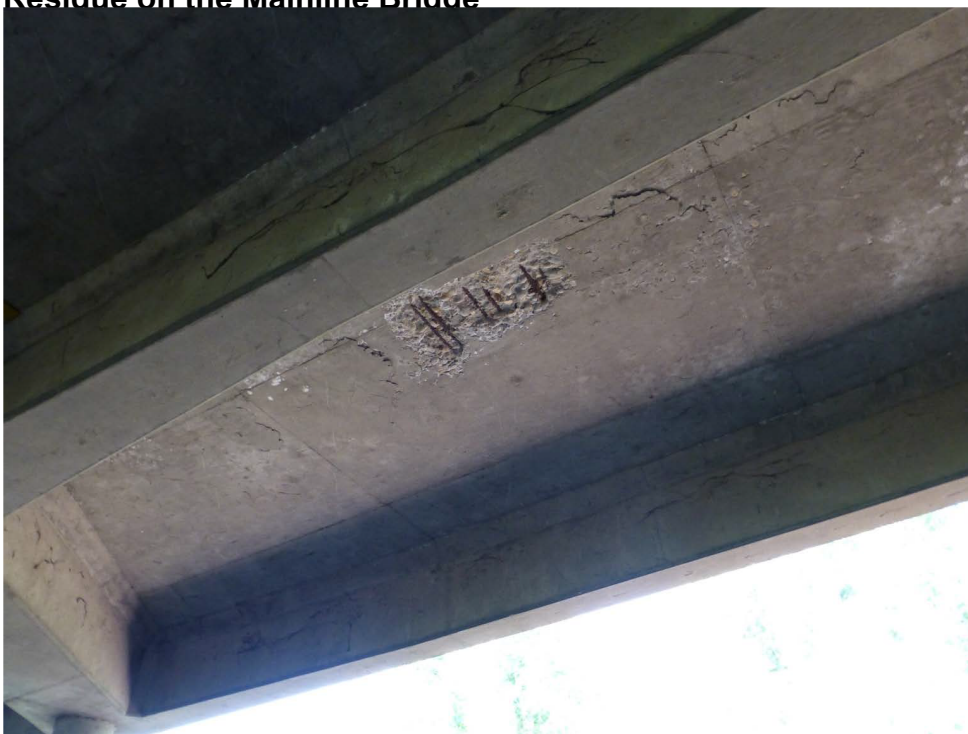
Figure 1-4 Bridge Soffit Distress, with Exposed Rebar, Cracks, and Salt Residue on the Mainline Bridge
