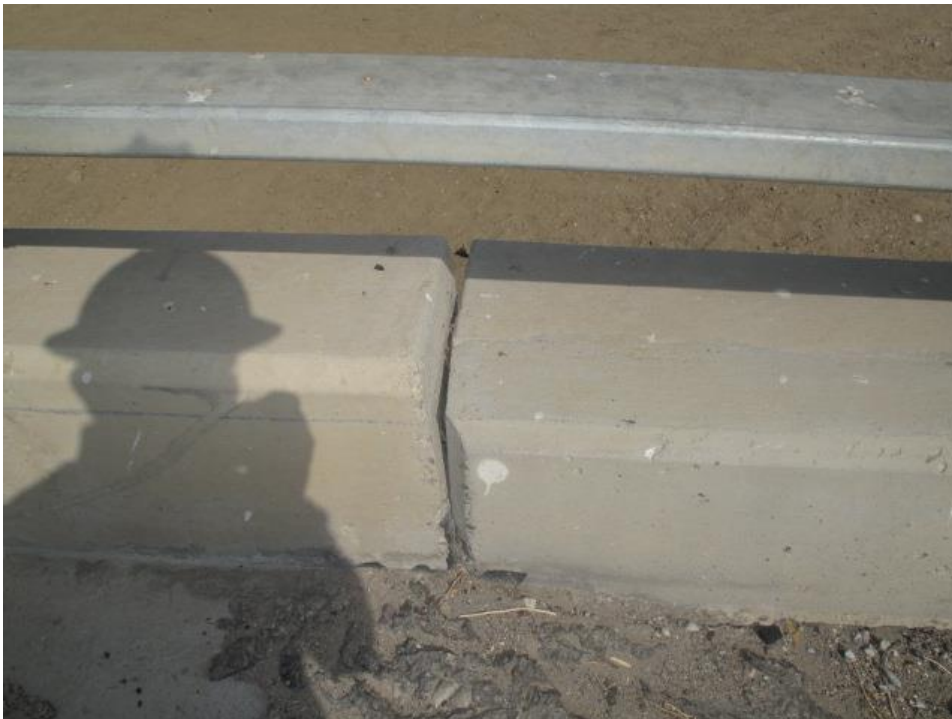
Displacement of the rail at an abutment can be seen in this image.
